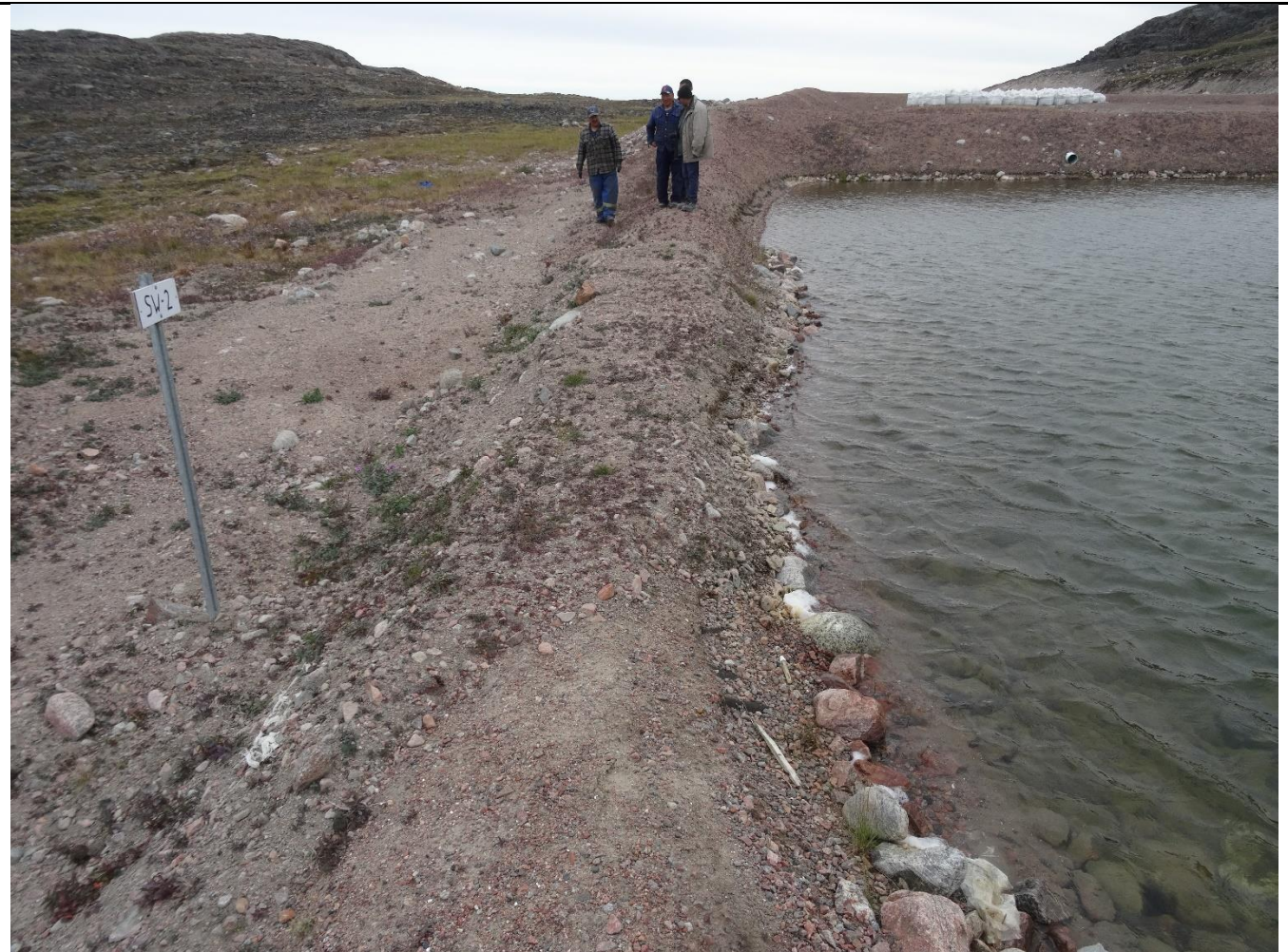
Description: Berm Repair adjacent to Sample Station SW-2 has been completed as requested from last Inspection – Thank you
