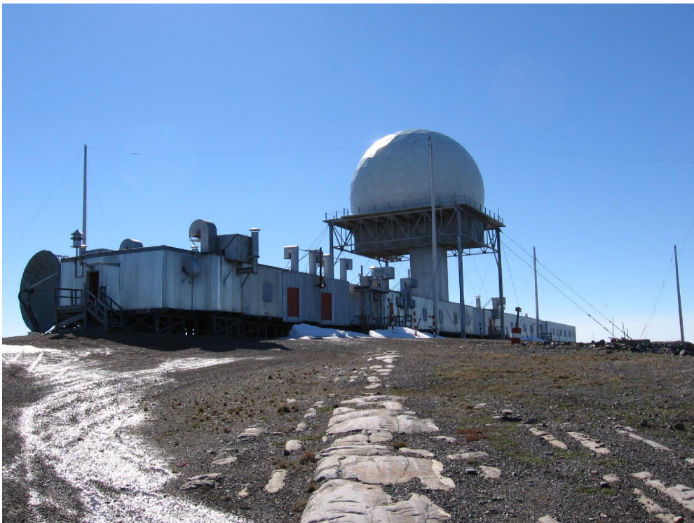
Photo 47: Module Train and Radome
