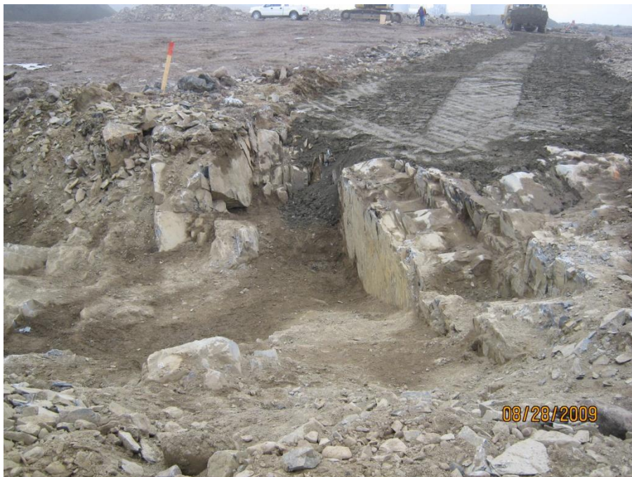
Photograph 2. Preparation of Tier II Key trench ___ ↑
