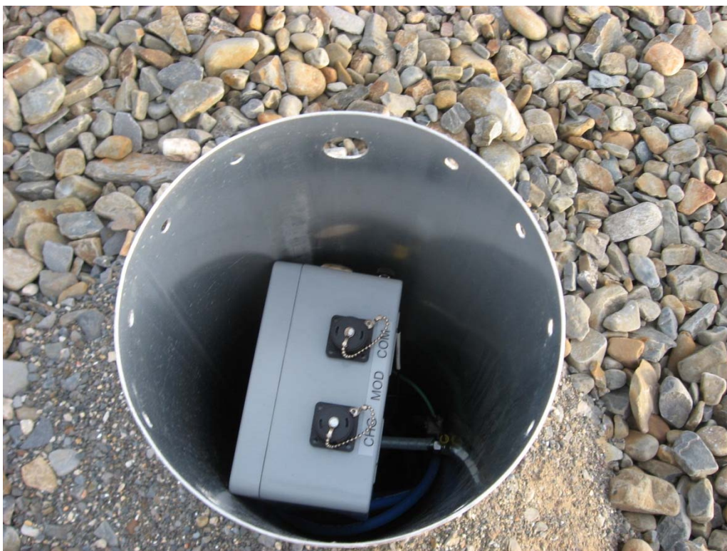
Photograph 117. VT-5 Data Logger (WP 109, FOX-2 24). ↑
