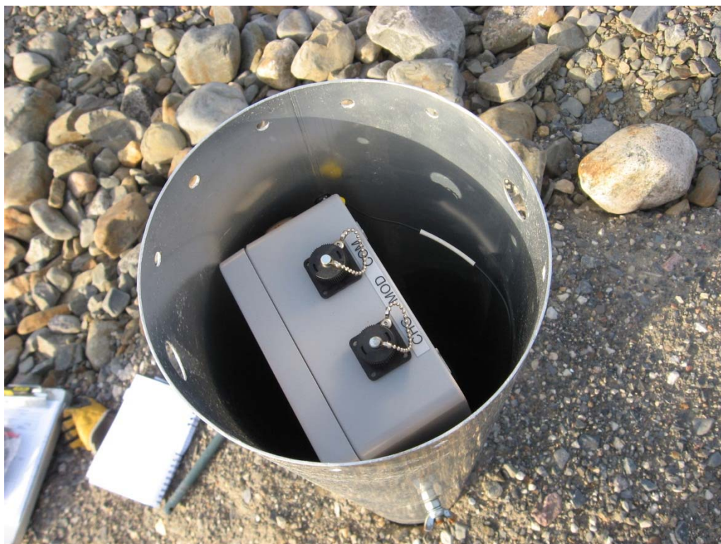
Photograph 115. VT-7 Data Logger (WP 107, FOX-2 22). ↑
