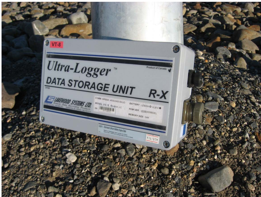
Photograph 126. VT-8 Data Logger (FOX-2 33). ↑
