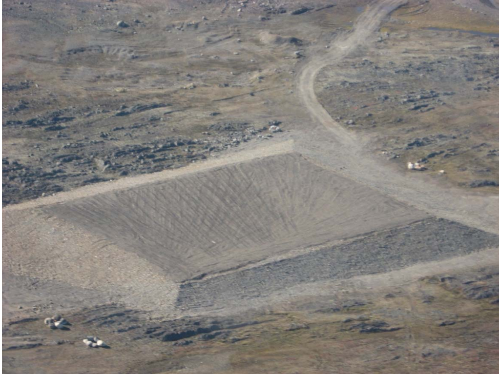
Photograph 144. Hangar Non-Hazardous Waste Landfill (FOX-2 154). ↑
