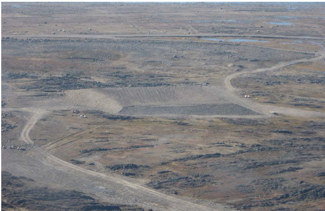
Photograph 143. Hangar Non-Hazardous Waste Landfill (FOX-2 149). ↑
