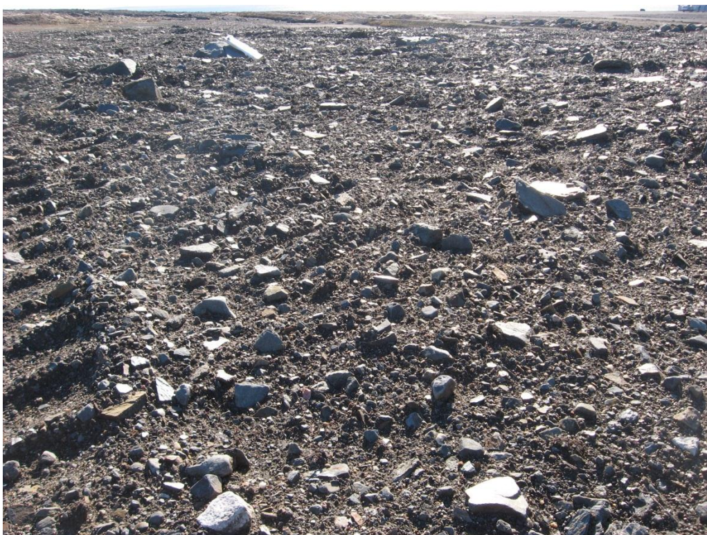
Photograph 12. Rough Finish Grading/Minor Settlement – Looking S (WP 153). ↑
