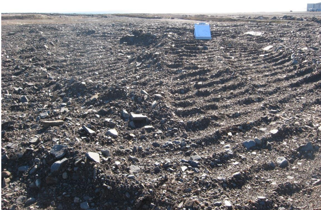
Photograph 14. Rough Finish Grading/Minor Settlement – Looking SW (WP 155). ↑
