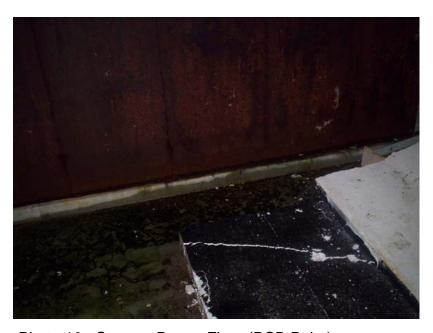
Photo 10: Storage Pantry Floor (PCB Paint)
