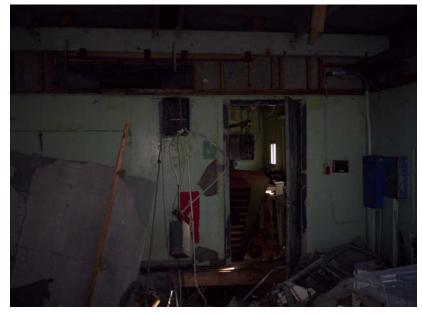
Photo 23: Green Paint in Radio Room (Lead Paint)
