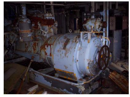
Photo 16: Generator in West Wing Engine Room (Lead Paint)
