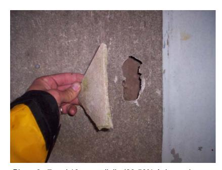
Photo 6: 7 and 10mm wall tile (20-50% Asbestos)
