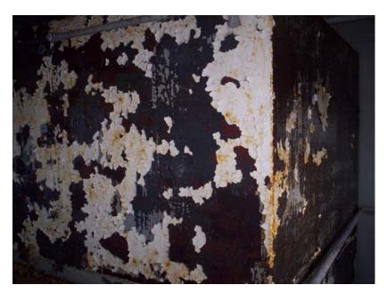
Photo 30: Tank in East Wing Fuel Room (Lead Paint)
