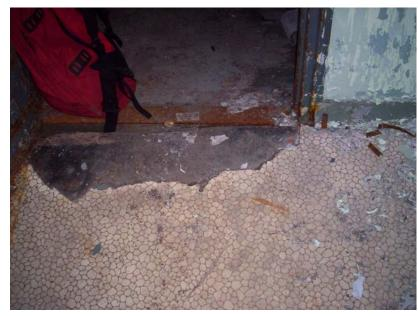
Photo 24: Sheet Floor in Covered Walkway (No Asbestos)
