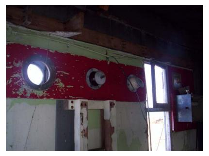
Photo 22: Red Paint in Radio Room (PCB Paint)
