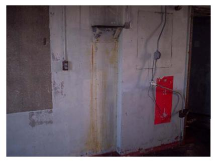
Photo 25: Grey Paint in East Wing Engine Room (Lead Paint)
