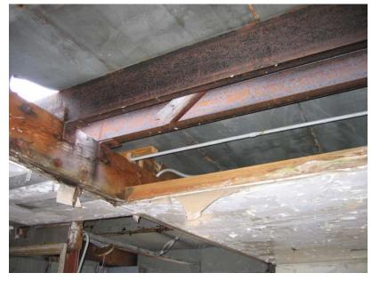
Photo 67: Roof Construction with Steel Channels
