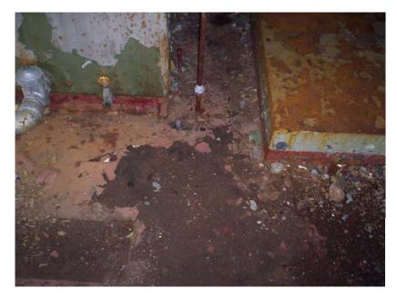
Photo 29: Floor Paint in East Wing Fuel Room (Lead Paint)
