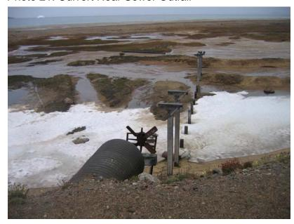
Photo 23: Supports for Water Line to ATB
