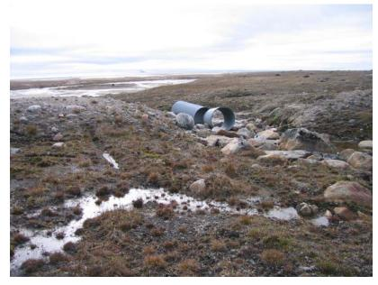
Photo 32: Washed Out Culvert at Old Road
