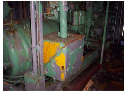
Photo 15: Generator in West Wing Engine Room (Lead Paint)
