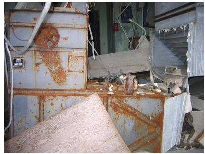
Photo 51: AC Unit Collapsed with Floor
