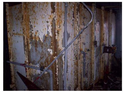
Photo 20: Fuel Tank in West Wing Vehicle Parts Storage (Lead Paint)
