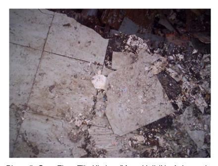
Photo 5: Grey Floor Tile Kitchen/Mess Hall (No Asbestos)
