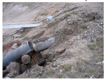
Photo 48: Failed Sections at Culvert Outlet Near Main Station Building
