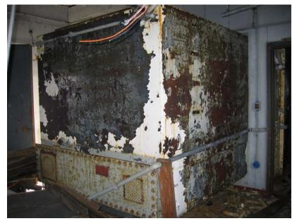
Photo 19: Fuel Tank in West Wing Fuel Room (Lead Paint)
