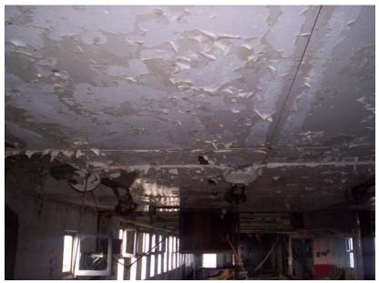
Photo 8: Kitchen Ceiling Paint (PCB Paint)
