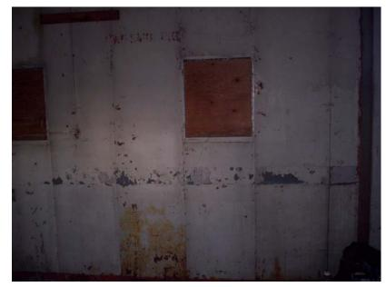
Photo 32: Grey paint of East Wing Garage Interior (PCB Paint)
