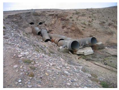
Photo 44: Embankment Culvert Failure at South End of Reservoir Road
