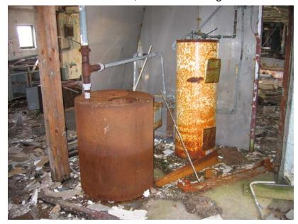
Photo 64: Kitchen Area Tanks, Hot Water and Grease Vat
