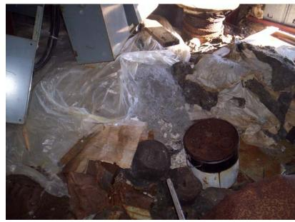
Photo 43: Insulation at East End of Hazmat building (30% Asbestos)
