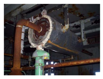
Photo 1: Tank Insulation in East Wing Engine Room (No Asbestos) Photo 2: White Pipe Insulation (20-40% Asbestos)
