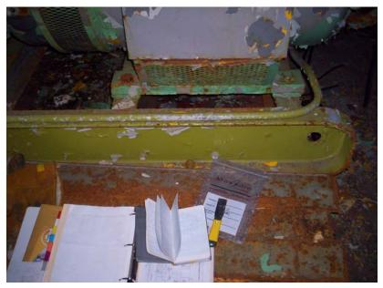
Photo 28: Green Paint on Base of Generator (Lead Paint)
