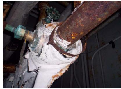
Photo 3: Grey Pipe Joint Insulation (40-60% Asbestos)
