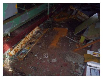
Photo 14: West Wing Engine Room Floor (Lead Paint)
