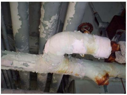
Photo 4: White Pipe Elbow Insulation (40% Asbestos)
