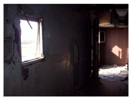
Photo 17: Grey Paint on Walls of West Wing Engine Room (Lead Paint)
