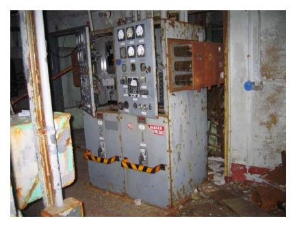
Photo 46: Electrical Panel for SE Generators
