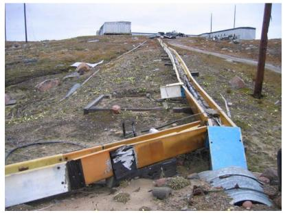
Photo 24: Branching of Utilidor at Road Corner
