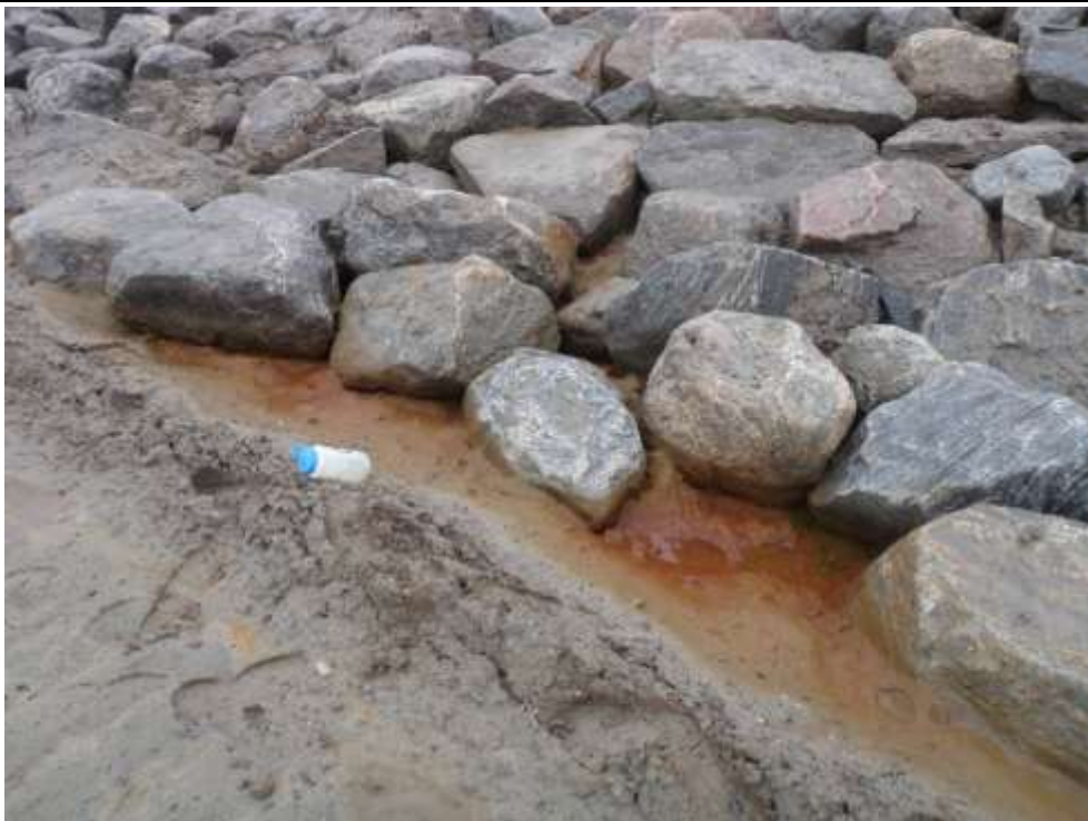
Ponded water with staining along the toe of NHL near the southwest corner. Viewpoint 61 (Figure A-1; Appendix A). Photograph reference 61 (CD-ROM). Direction photo taken: NE
