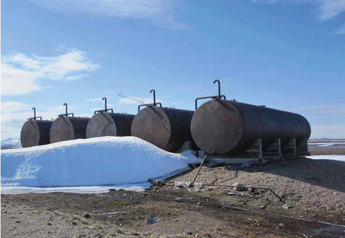
The Five (5) 100,000 Litres each Aboveground Storage Tanks (Before Remediation)
