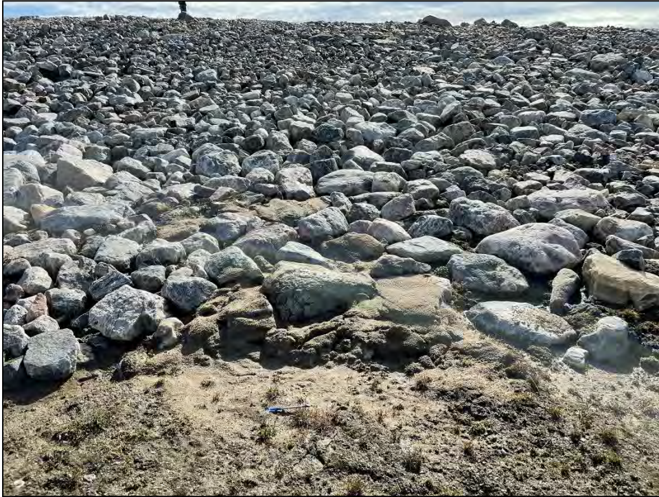
Photo 37: Sign of erosion on the northern berm (Feature U), facing south.
