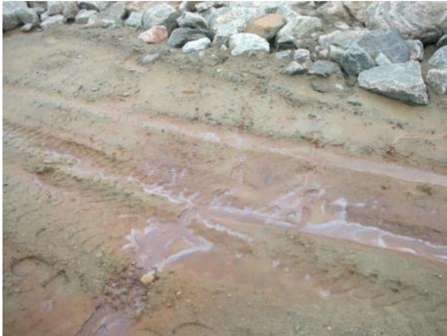
Small erosion channel and staining near the north side of the NHWL. Soil sample CC-SS2/DUP1 collected from this area. Viewpoint 83 (Figure A-1; Appendix A). Photograph reference 83 (CD-ROM). Direction photo taken: SE
