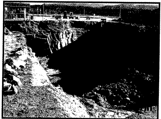
Excavating 8000 m 3 of Petroleum Hydrocarbon Contaminated Soil
