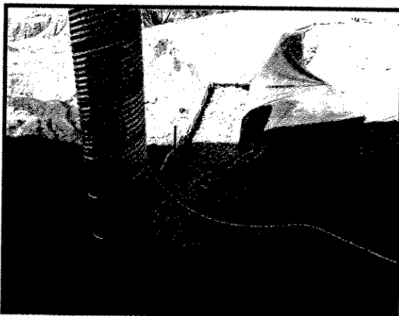
Installing Collection Pipe in French Drain
