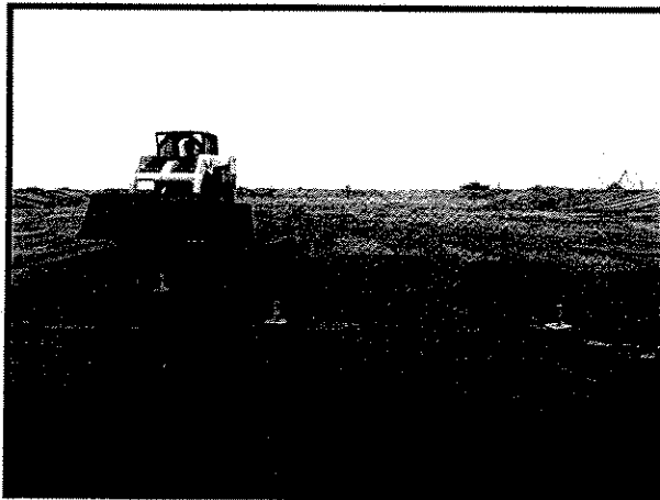
Placing Sand Bed on Liner in Land Treatment Unit
