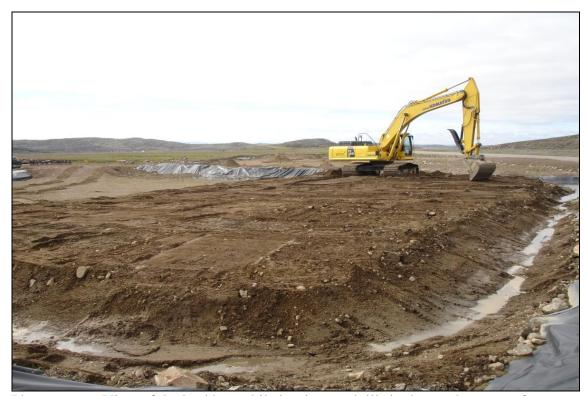
Photo 6: View of the backhoe while it mixes and tills in the north corner of the pad.
