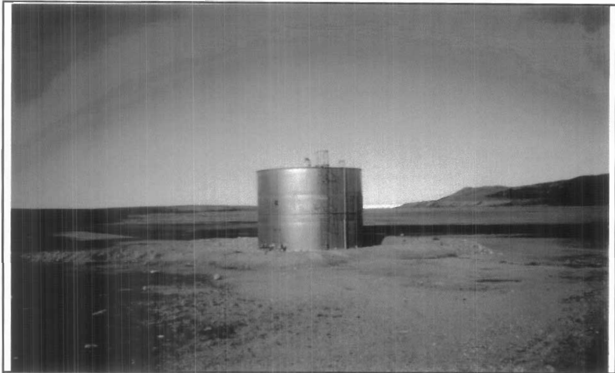
Photo 11: 65,000 gallon POL tank at the Lower Site.
