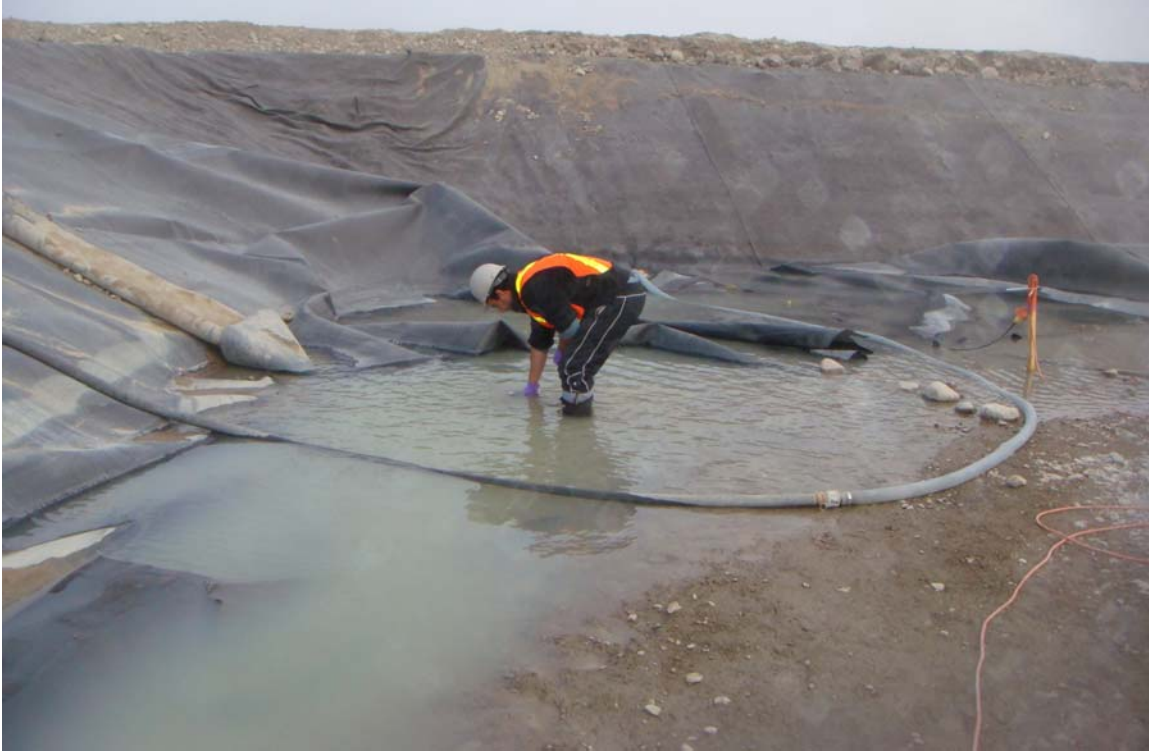
Photo 6 (DSC01620): Sample 09-22271 and 09-23816 photo is taken from the top of the western berm of the land farm looking east along the trench dug for removing upwelling groundwater in the landfarm from entering into the discharging water.
