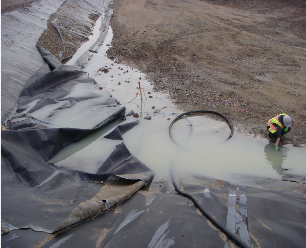
Photo 5 (DSC00746): Sample 09-17599 east along the trench dug for removing upwelling groundwater in the landfarm. The area is also bermed off to prevent any surface water from the landfarm from entering into the discharging water.
