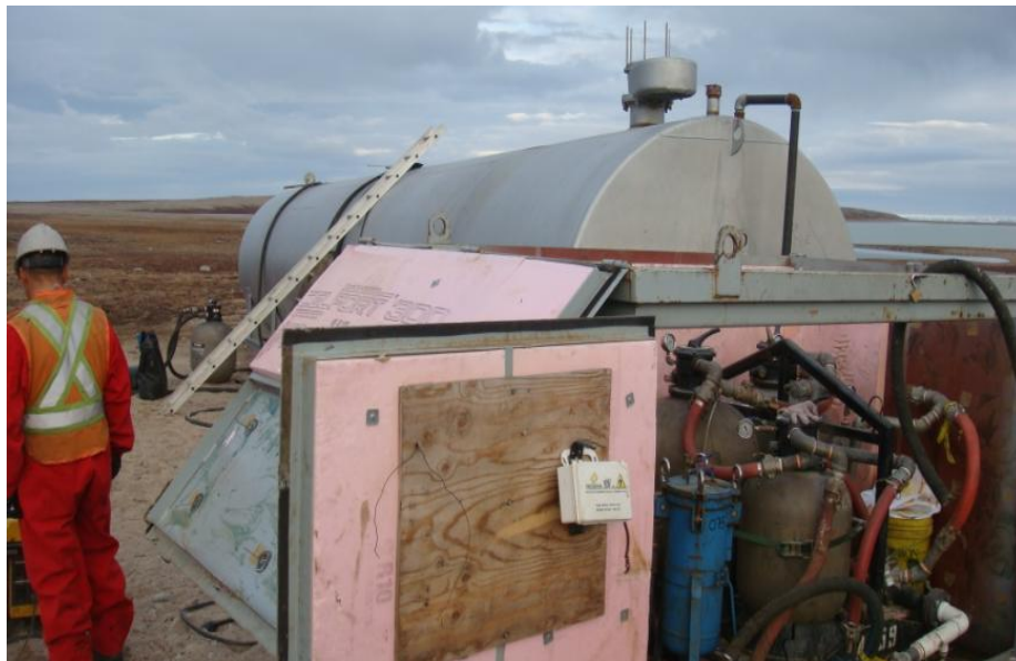
Photo 6 (DSC01723) Sample 10-28669: Wide angle of Tank 2, facing NW. The sample was collected from a hole in the top of the tank. The primary wastewater treatment system is in the foreground and a second wastewater treatment system is visible behind the ladder on the left of the picture.
