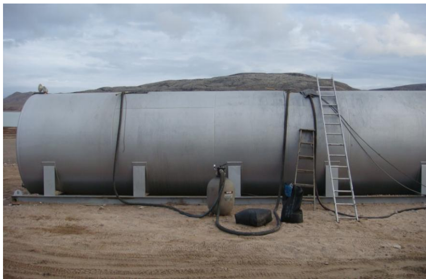
Photo 7 (DSC01722) Sample 10-28670: Wide angle of Tank 2, facing north. The sample was collected from the effluent from the activated carbon wastewater treatment system. The effluent is pumped back into the tank at the left side of the picture.
