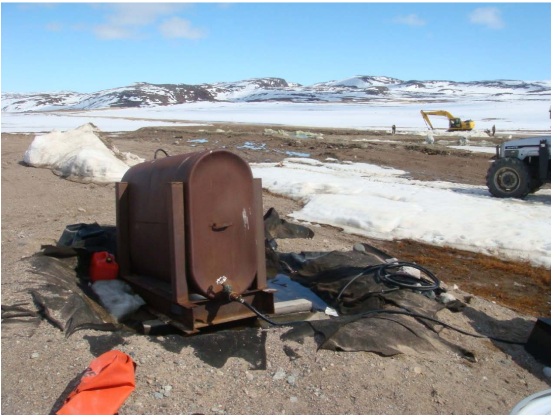
Photograph 1 (DSC00932): Diesel Tank and hose where the fuel leaked from (coiled on the berm to the right of the photo) with Cell 1 and 2 of the Sewage Lagoon in the background.
