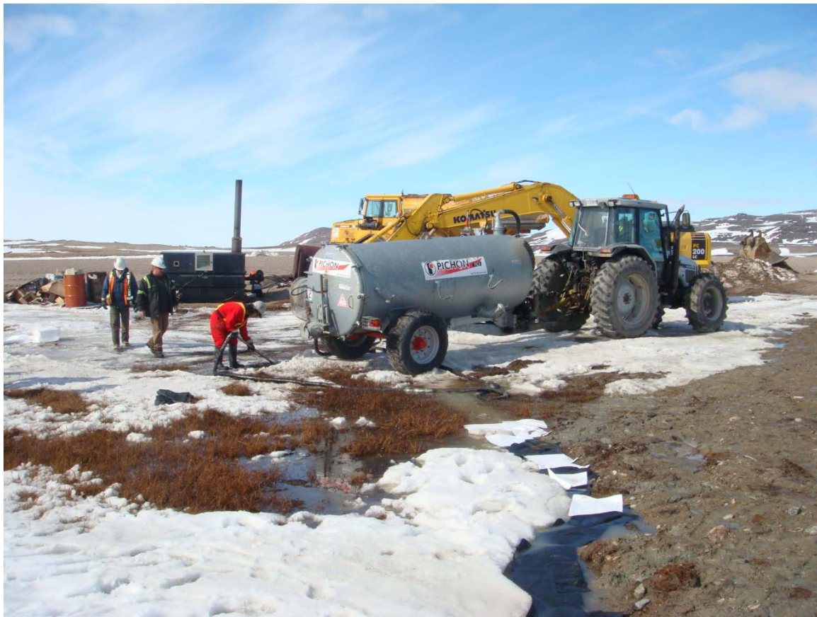
Photograph 2 (DSC00944): Biogenie employee using the Pichon vacuum system to skim the free product from the melt water stream. Absorbent pads downgradient of the spill in the melt water stream are seen in the foreground. The Incinerator and fuel tank are visible in the background.
