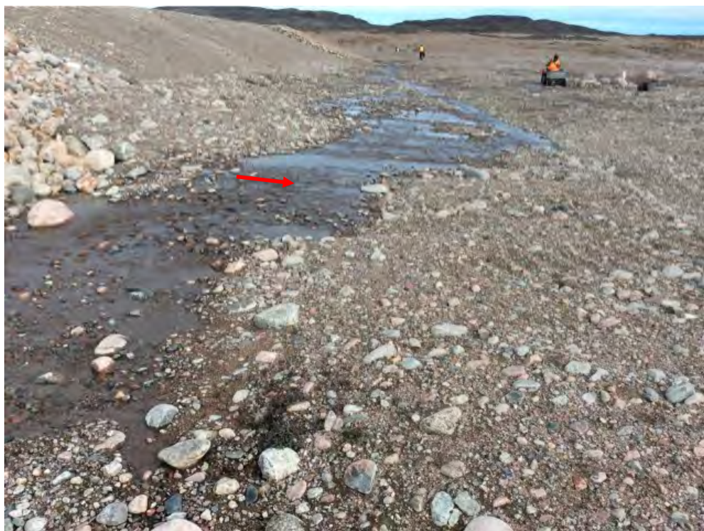
Photo 101: Non-Hazardous Waste Landfill- South toe, Feature E-Ponded/Running water along toe, facing east (Acceptable) (CAM5_Photo35.jpg)
