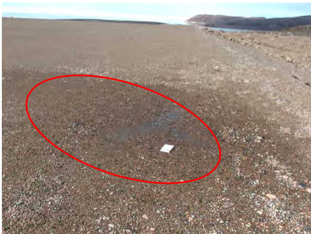
Photo 113: Non-Hazardous Waste Landfill- Cover surface, Feature P-Pond water and wet area, facing north (Acceptable) (CAM5_Photo17.jpg)
