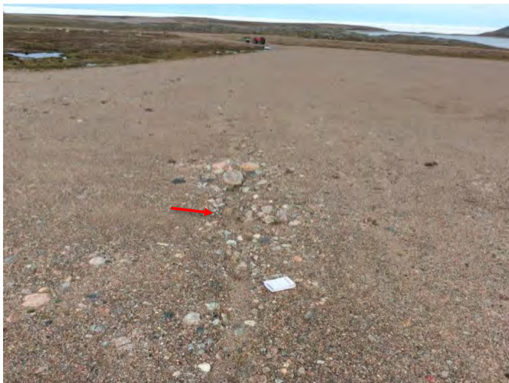
Photo 26: Lower Site Landfill South- Southwest crest, Feature D-Linear depression, facing northwest (Acceptable) (CAM5_Photo66.jpg)
