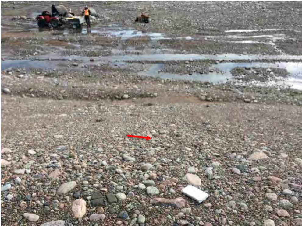
Photo 97: Non-Hazardous Waste Landfill- South slope, Feature H-Self-armouring erosion, facing southeast (Acceptable) (CAM5_Photo32.jpg)
