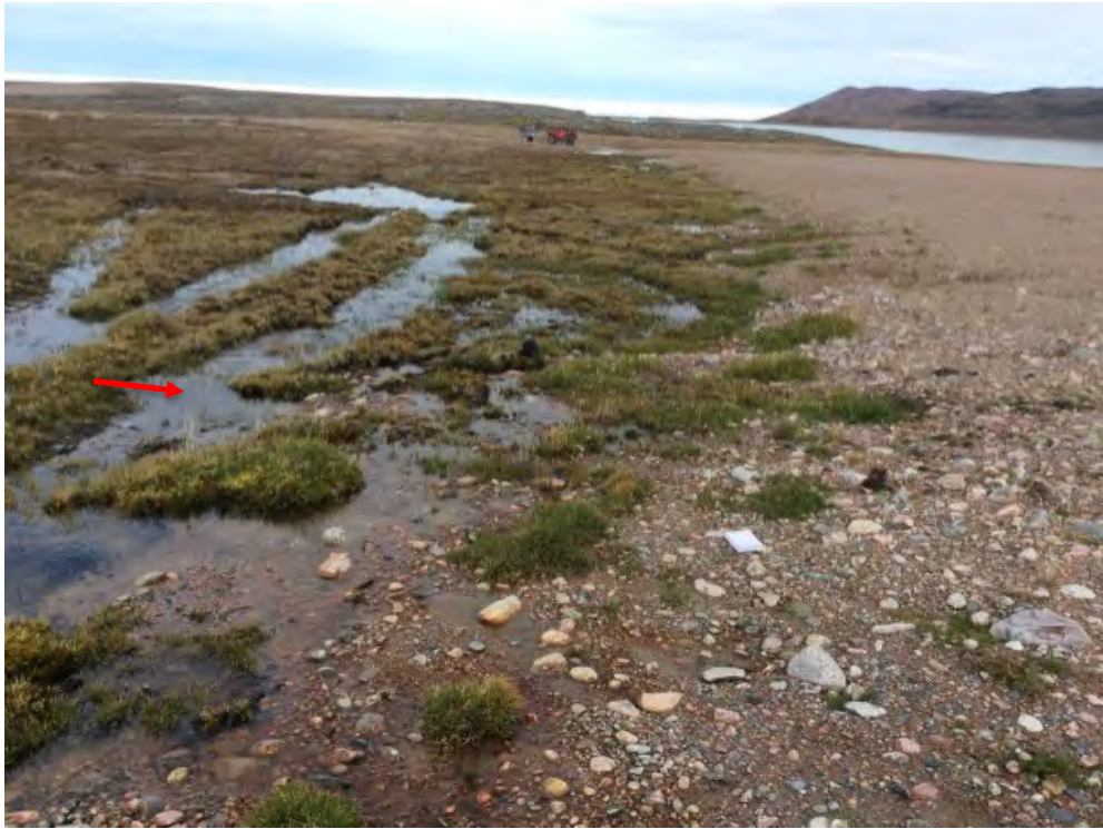
Photo 45: Lower Site Landfill South- Southwest toe, Feature Q1-Ponded water along toe, facing northwest (Acceptable) (CAM5_Photo57.jpg)
