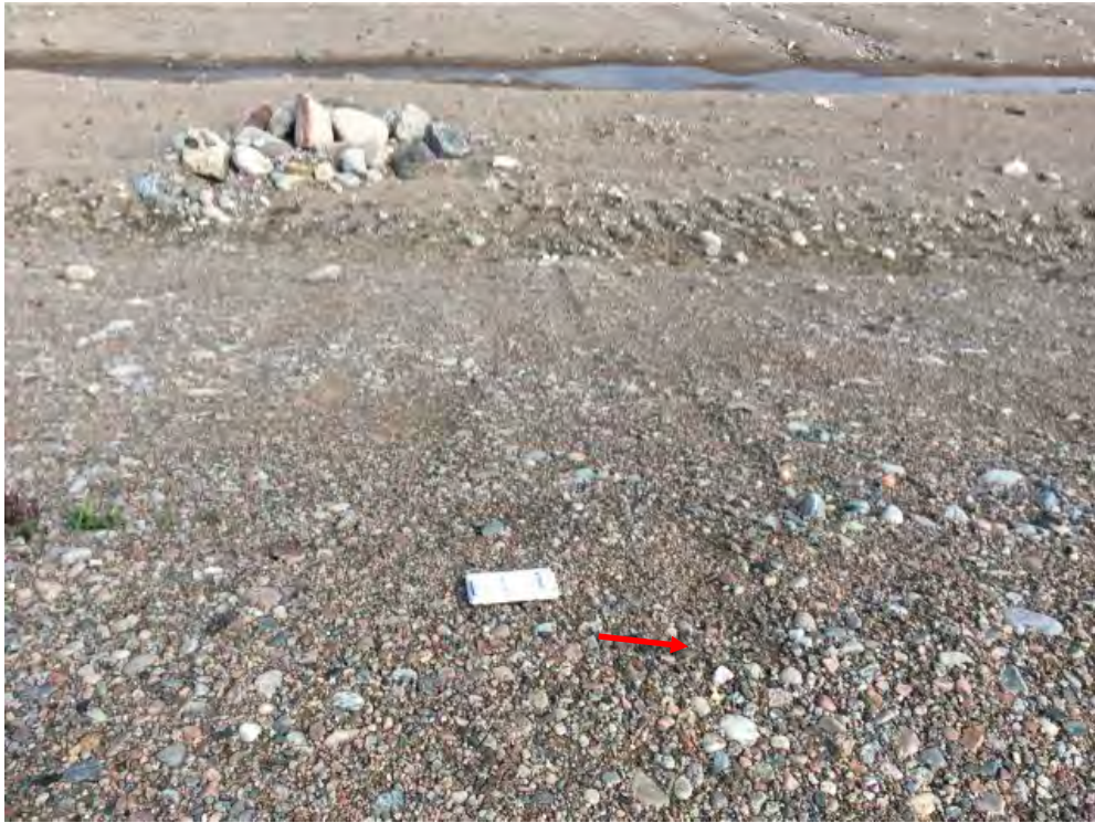
Photo 107: Non-Hazardous Waste Landfill- East slope, Feature L-Self-armouring erosion, facing northeast (Acceptable) (CAM5_Photo19.jpg)
