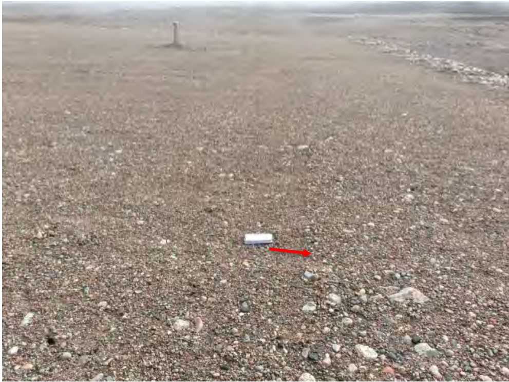
Photo 191: Tier II Disposal Facility- Cover surface, Feature F-Minor erosion channel, facing southeast (Acceptable) (CAM5_Photo4.jpg)
