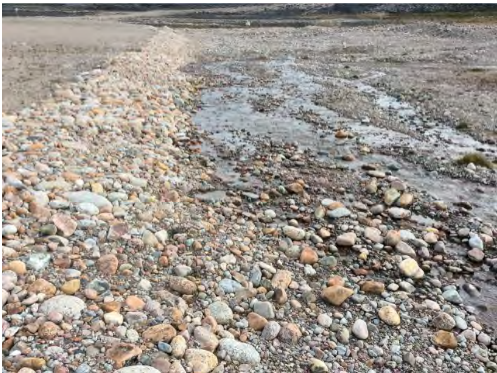
Photo 154: USAF & Asbestos Landfill- West toe, Feature O-Ponded water along toe, facing southeast (Acceptable) facing south (CAM5_Photo45.jpg)
