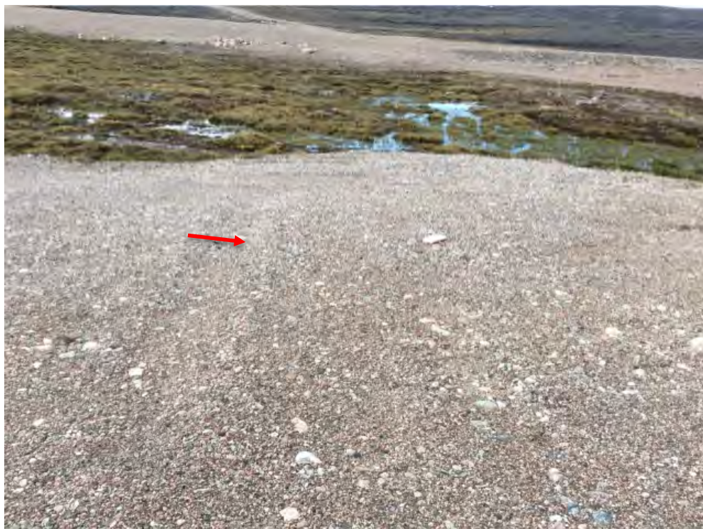
Photo 50: Lower Site Landfill South- cover surface near south slope, Feature V2-Minor erosion channels, facing southwest (Acceptable) (CAM5_Photo62.jpg)
