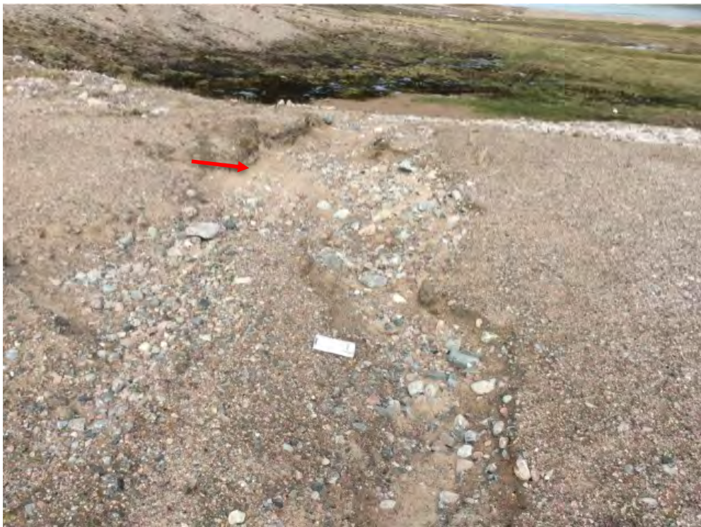
Photo 32: Lower Site Landfill South- Northwest slope, Feature H-Major erosion gully, facing northwest (Acceptable) (CAM5_Photo90.jpg)
