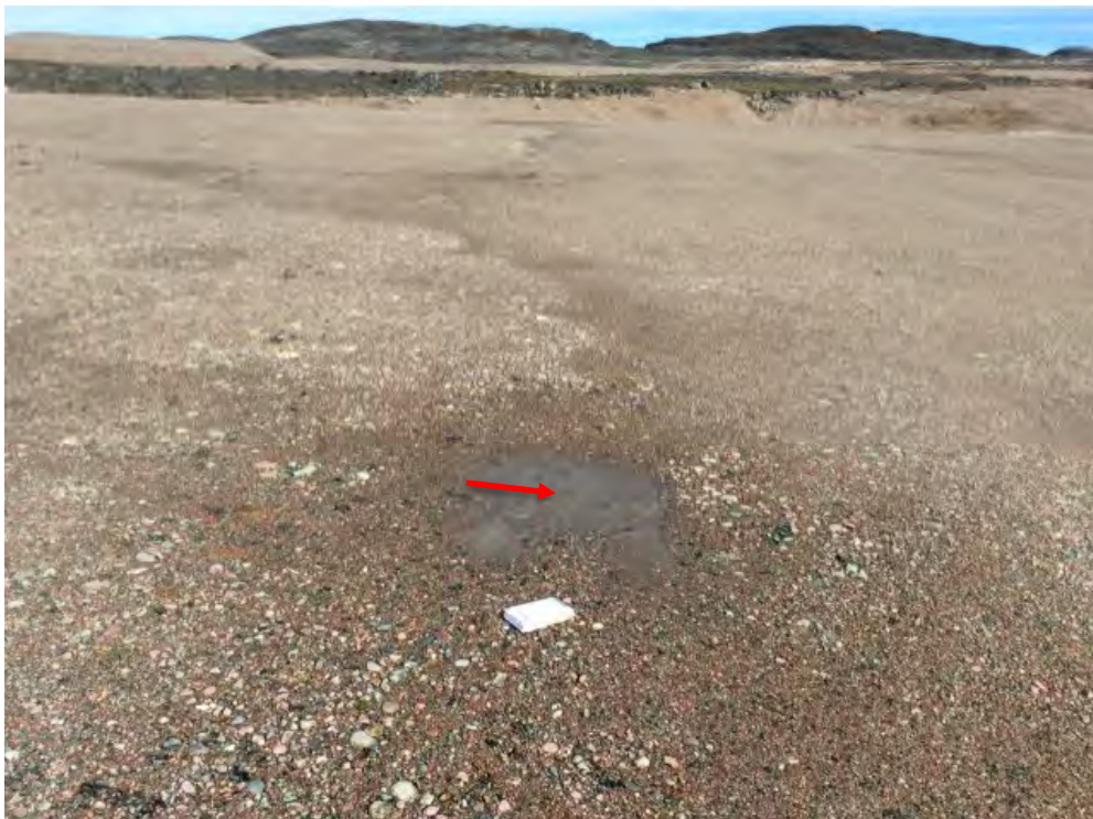
Photo 116: Non-Hazardous Waste Landfill- Cover surface, Feature P -Ponded water, facing east (Acceptable) (CAM5_Photo30.jpg)
