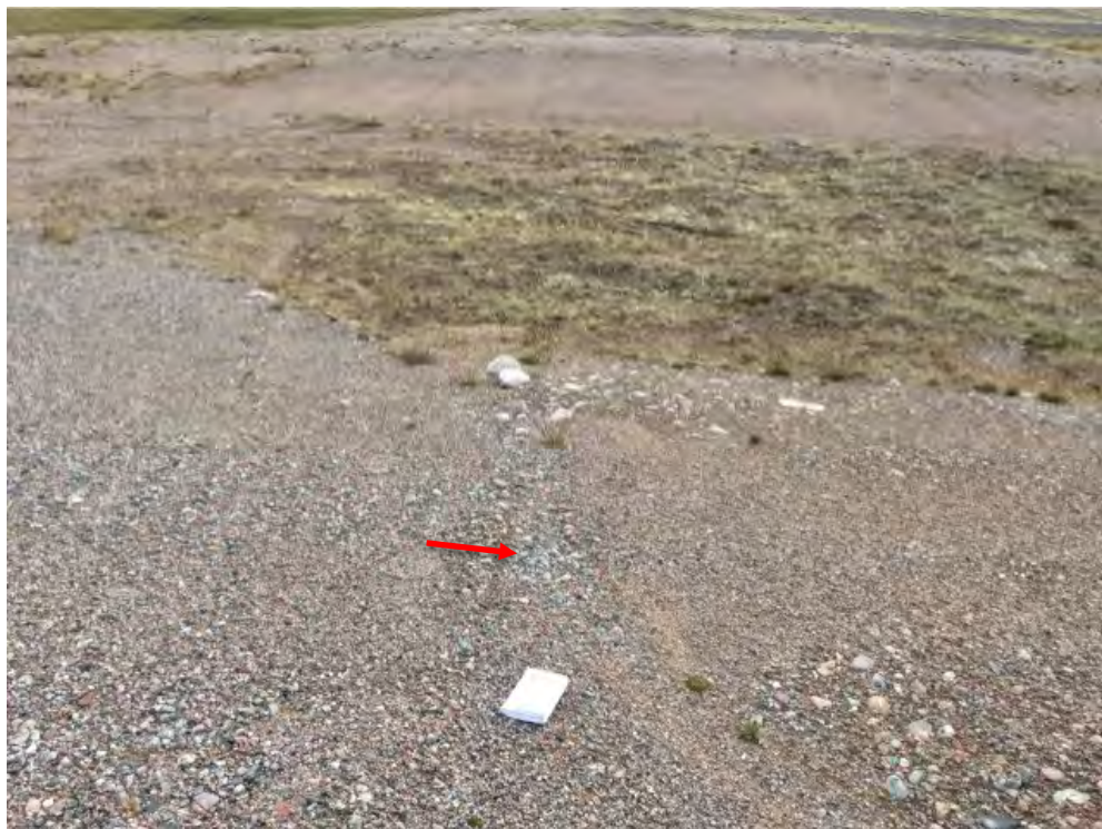
Photo 59: Lower Site Landfill South- Southeast slope, Feature AA -Self armouring erosion, facing southeast (Acceptable) (CAM5_Photo69.jpg)
