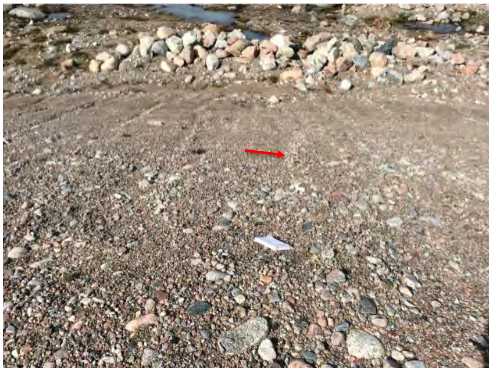
Photo 92: Non-Hazardous Waste Landfill- North slope, Feature B-Self-armouring erosion, facing northwest (Acceptable) (CAM5_Photo25.jpg)
