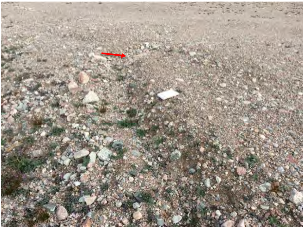
Photo 150: USAF & Asbestos Landfill- Northwest slope, Feature L-Minor erosion channel, facing east (Acceptable) (CAM5_Photo46.jpg)
