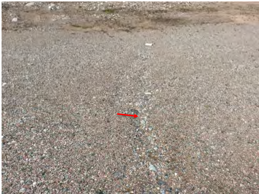
Photo 34: Lower Site Landfill South- Northwest slope, Feature J-Minor erosion channel, facing northwest (Acceptable) (CAM5_Photo91.jpg)
