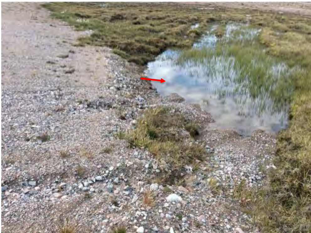
Photo 42: Lower Site Landfill South- Northwest toe, Feature O-Ponded water at toe, facing west (Acceptable) (CAM5_Photo94.jpg)
