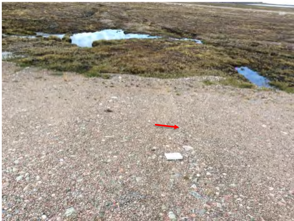
Photo 21: Lower Site Landfill South- West slope, Feature A4-Minor self-armouring erosion, facing southwest (Acceptable) (CAM5_Photo56.jpg)
