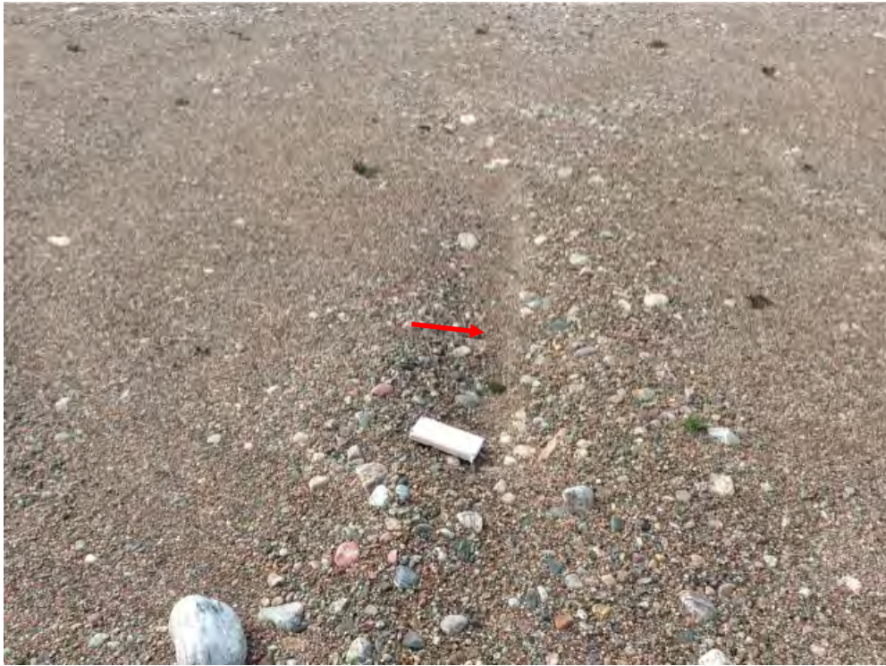
Photo 149: USAF & Asbestos Landfill- Southeast crest surface, Feature K-Linear depression, facing north (Acceptable) (CAM5_Photo39.jpg)
