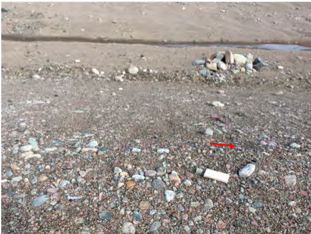
Photo 104: Non-Hazardous Waste Landfill- East slope, Feature L-Self-armouring erosion, facing northeast (Acceptable) (CAM5_Photo20.jpg)
