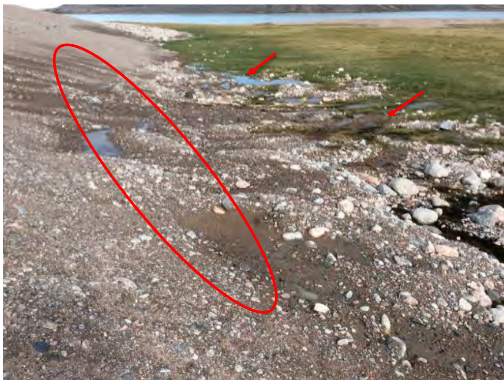
Photo 29: Lower Site Landfill South- East toe, Feature G-Intermittent ponded water (arrows) along toe with less iron staining, Feature W2-Wet area on slope (ellipse), facing northwest (Acceptable) (CAM5_Photo80.jpg)
