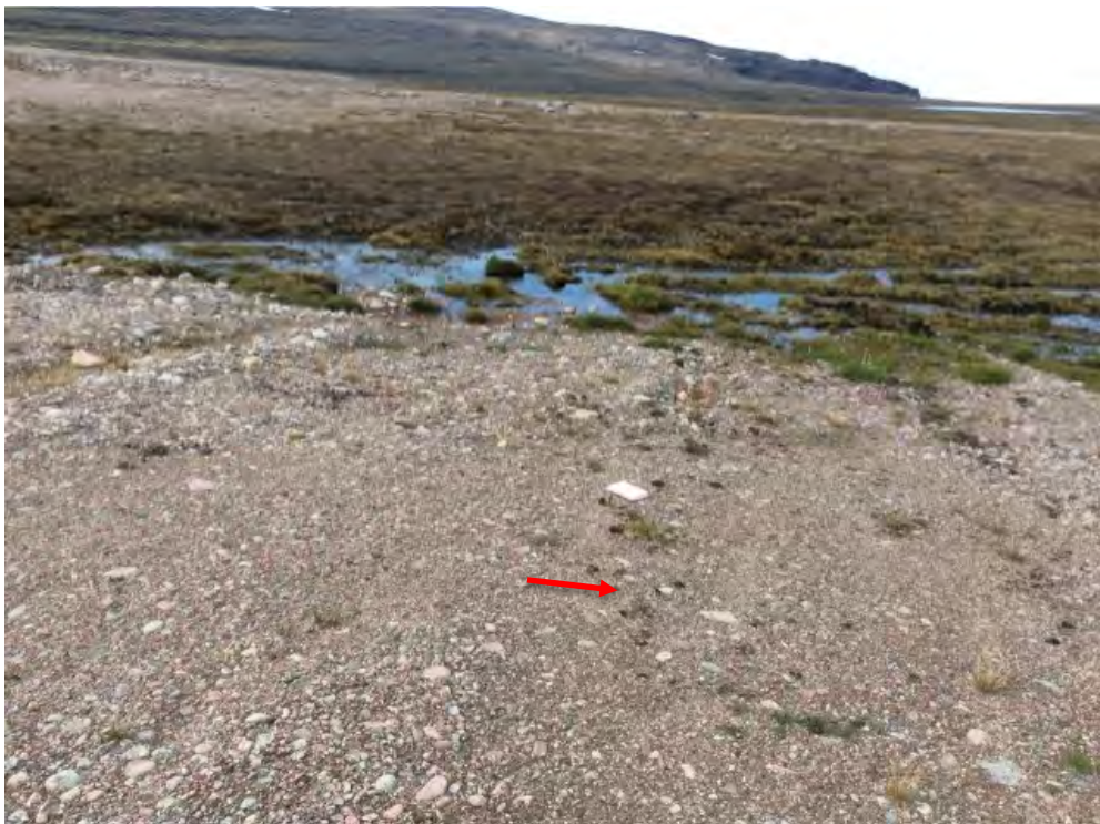
Photo 24: Lower Site Landfill South- West slope, Feature A5-Minor self-armouring erosion, facing southwest (Acceptable) (CAM5_Photo59.jpg)
