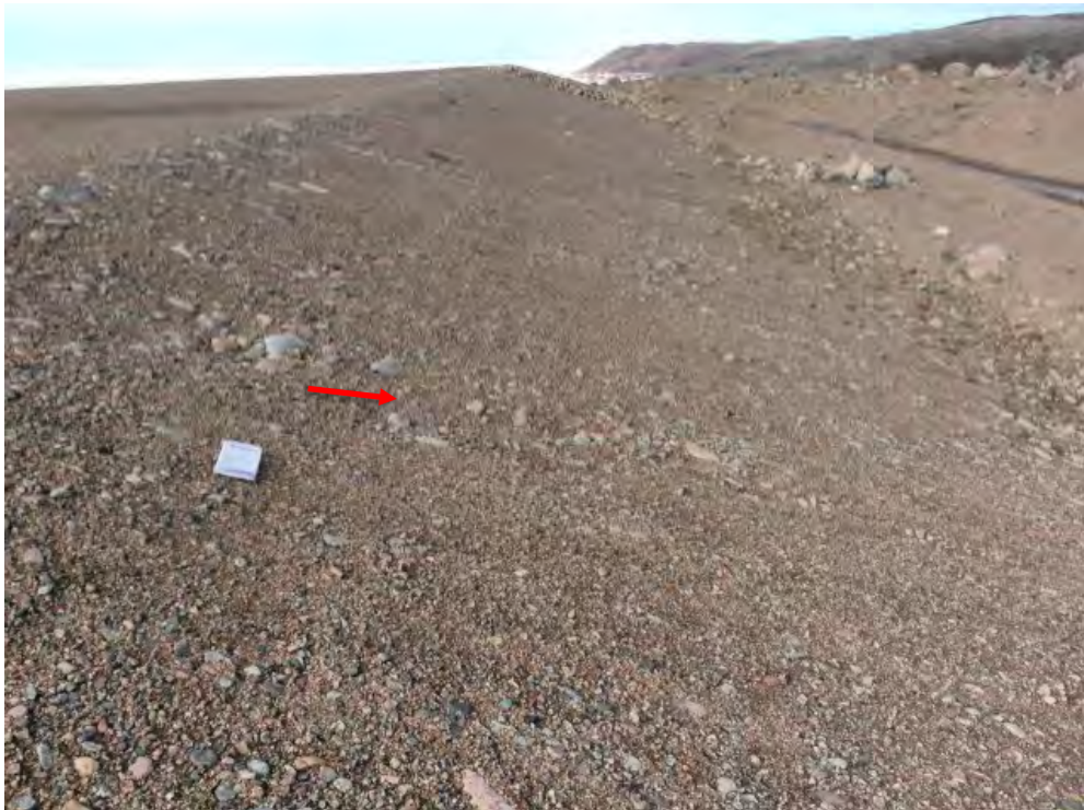
Photo 108: Non-Hazardous Waste Landfill- East slope, Feature L-Self-armouring erosion, facing northwest (Acceptable) (CAM5_Photo18.jpg)
