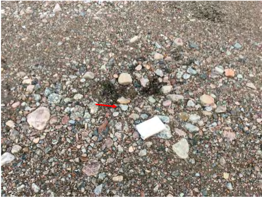
Photo 153: USAF & Asbestos Landfill- Northeast crest surface, Feature N-Minor settlement, facing south (Acceptable) (CAM5_Photo49.jpg)
