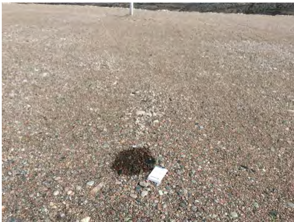
Photo 185: Tier II Disposal Facility- Central crest surface, Feature C-Possible hydrocarbon stain, facing northeast (Acceptable) (CAM5_Photo8.jpg)
