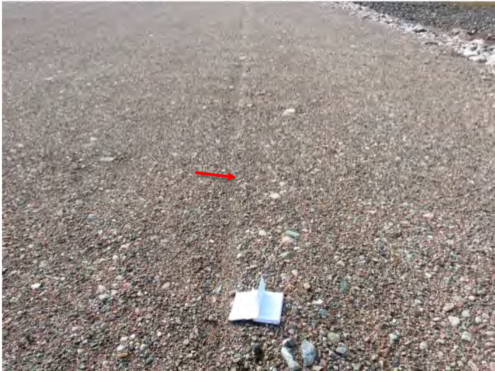
Photo 187: Tier II Disposal Facility- Northeast crest surface, Feature E-Minor erosion channel, facing southwest (Acceptable) (CAM5_Photo9.jpg)
