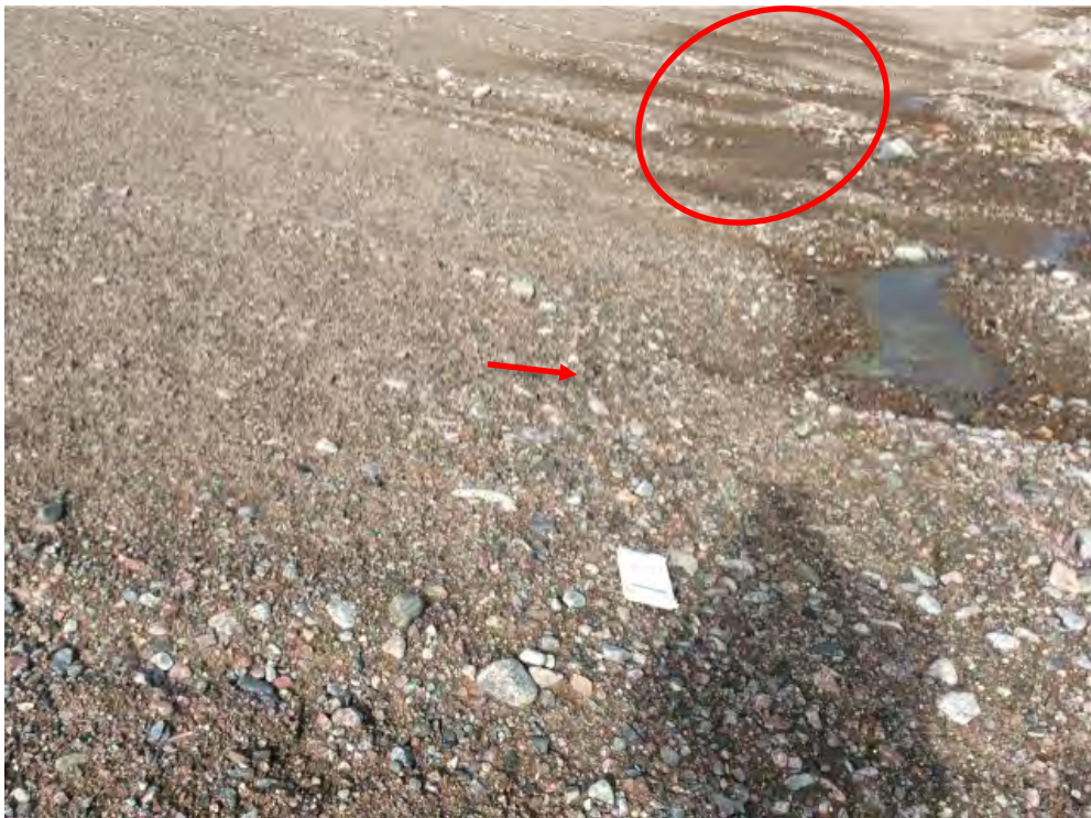
Photo 28: Lower Site Landfill South- Toe of east slope, Feature F1-Previously observed crack on slope above toe (arrow), Feature W2-Wet area on slope (circle), facing northwest (Acceptable) (CAM5_Photo81.jpg)
