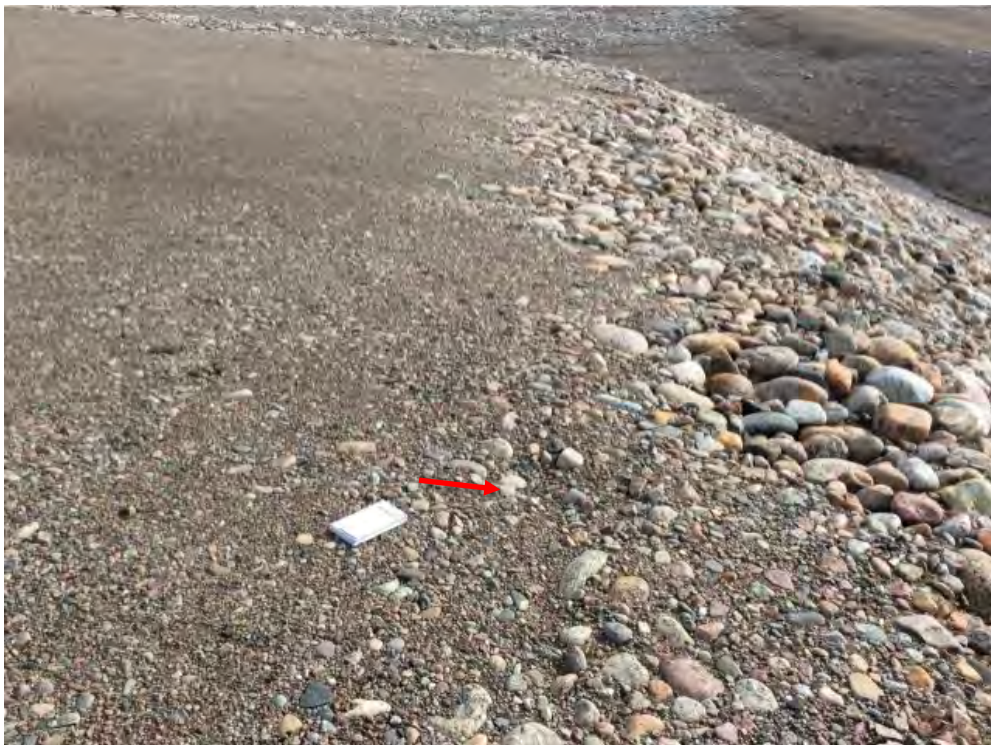
Photo 96: Non-Hazardous Waste Landfill- Southwest corner along crest, Feature G-Minor linear settlement near crest, facing southeast (Acceptable) (CAM5_Photo28.jpg)
