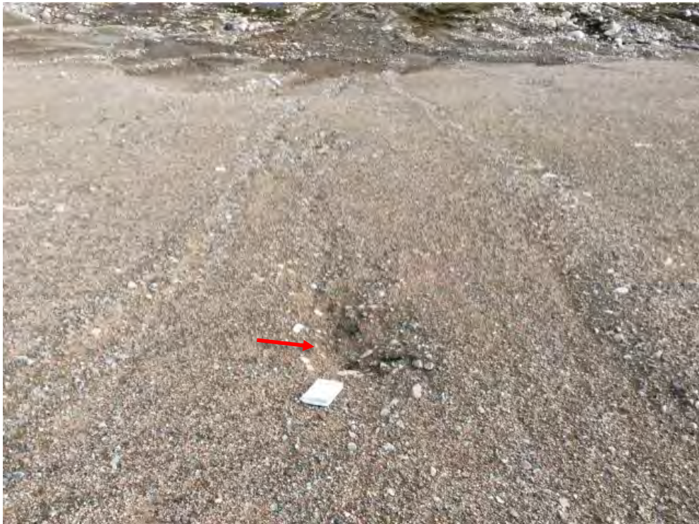
Photo 38: Lower Site Landfill South- East crest, Feature M-Minor settlement, facing northeast (Acceptable) (CAM5_Photo78.jpg)
