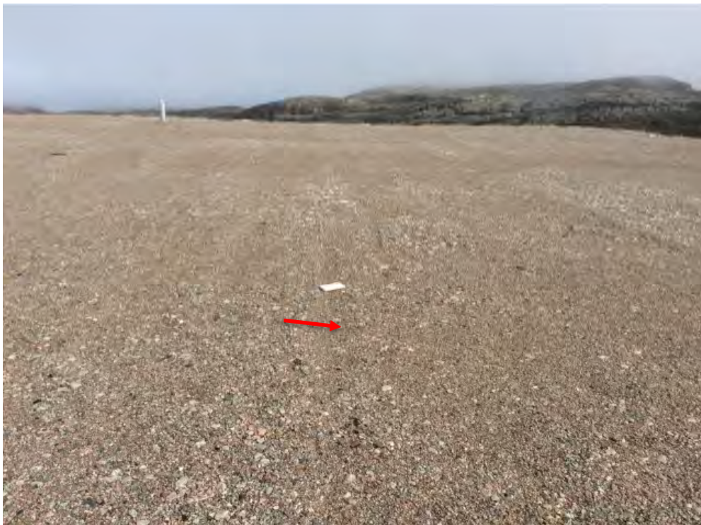
Photo 190: Tier II Disposal Facility- Cover surface, Feature E-Minor erosion channel, facing northeast (Acceptable) (CAM5_Photo7.jpg)
