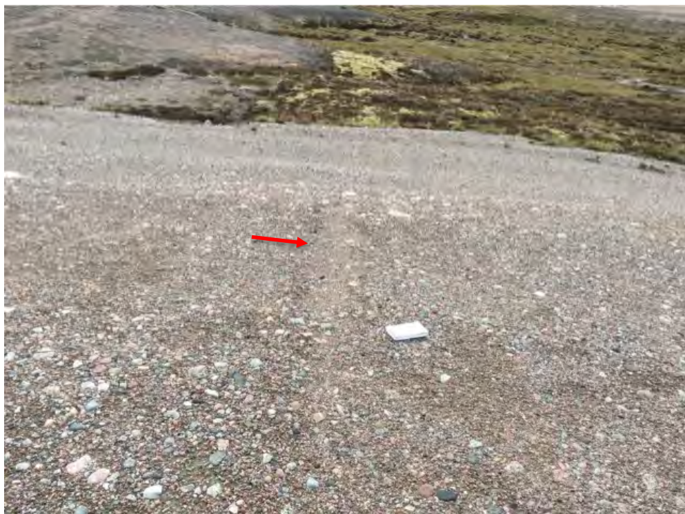
Photo 52: Lower Site Landfill South- South slope, Feature V1-Minor erosion channels, facing southeast (Acceptable) (CAM5_Photo65.jpg)
