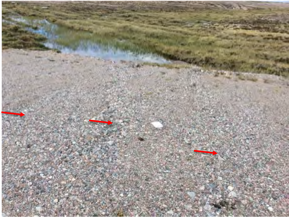
Photo 33: Lower Site Landfill South- Northwest slope, Feature I-Minor self-armouring erosion, facing northwest (Acceptable) (CAM5_Photo93.jpg)
