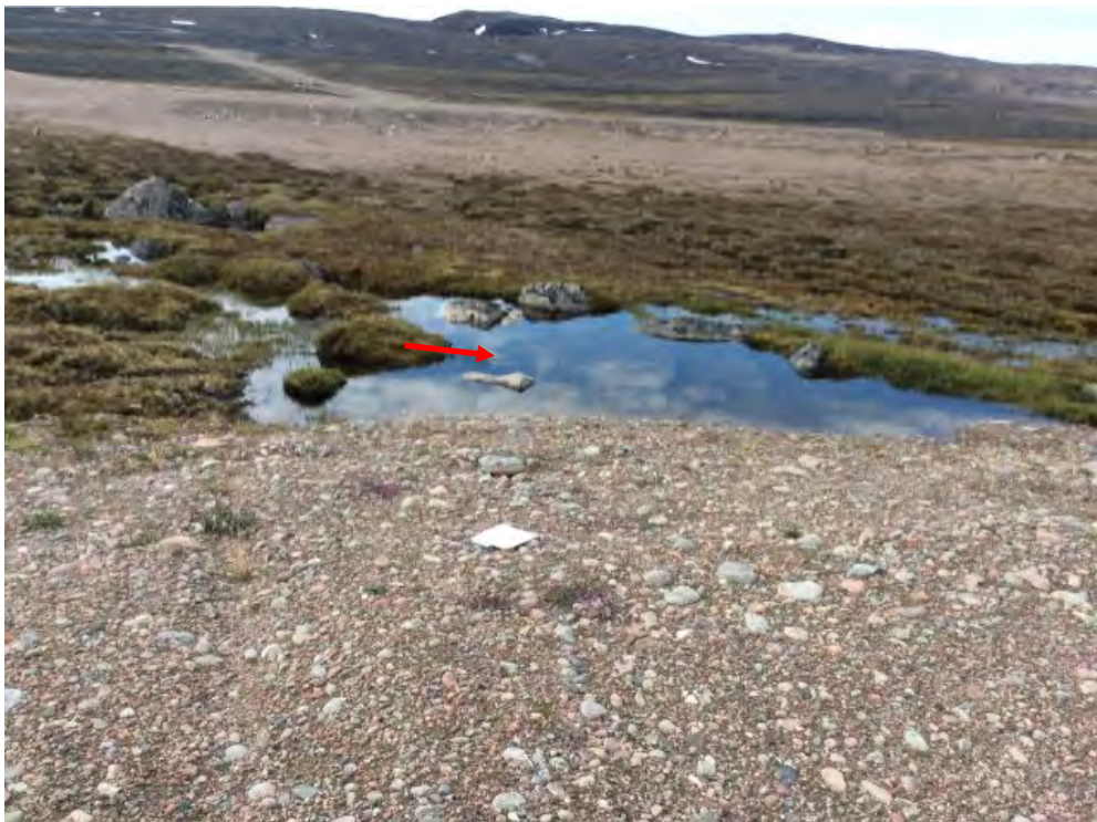
Photo 46: Lower Site Landfill South- Southwest toe, Feature Q1-Ponded water along toe, facing south (Acceptable) (CAM5_Photo60.jpg)
