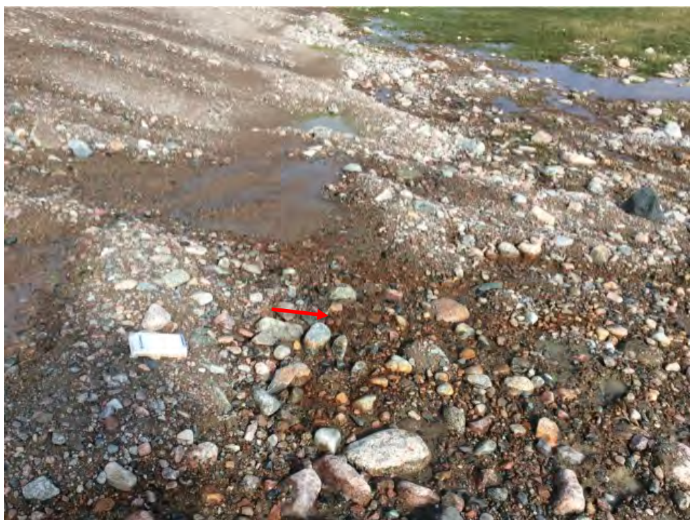
Photo 30: Lower Site Landfill South- East toe, Feature G-Previously reported as seepage with iron staining, intermittent ponded water with less staining in 2017, facing northwest (Acceptable) (CAM5_Photo83.jpg)
