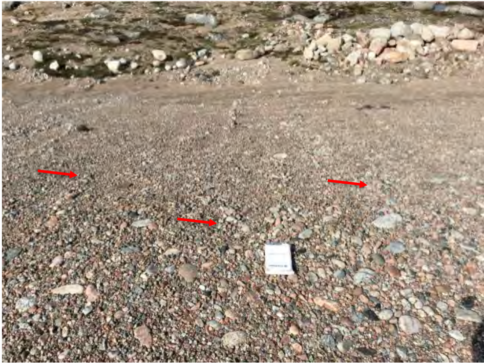
Photo 103: Non-Hazardous Waste Landfill- North slope, Feature K-Self-armouring erosion, facing northwest (Acceptable) (CAM5_Photo26.jpg)
