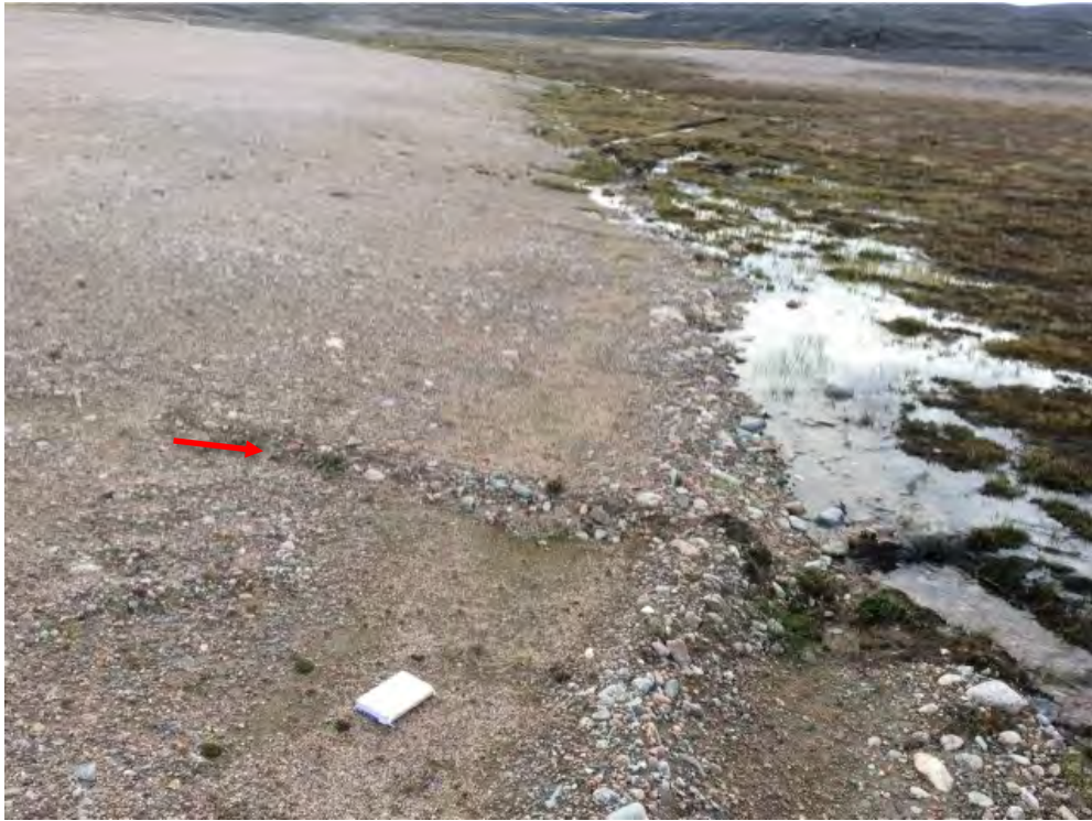
Photo 23: Lower Site Landfill South- West slope, Feature A2-Minor self-armouring erosion, facing southeast (Acceptable) (CAM5_Photo54.jpg)
