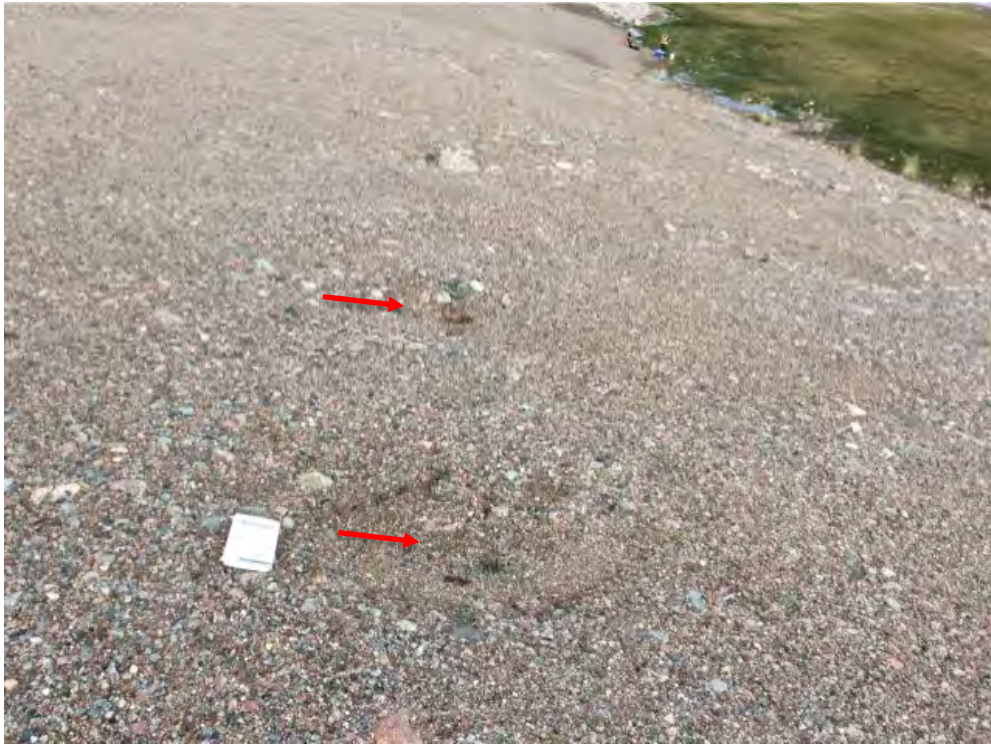
Photo 27: Lower Site Landfill South- Cover surface east corner, Feature E-Two small minor settlement areas, facing northwest (Acceptable) (CAM5_Photo70.jpg)
