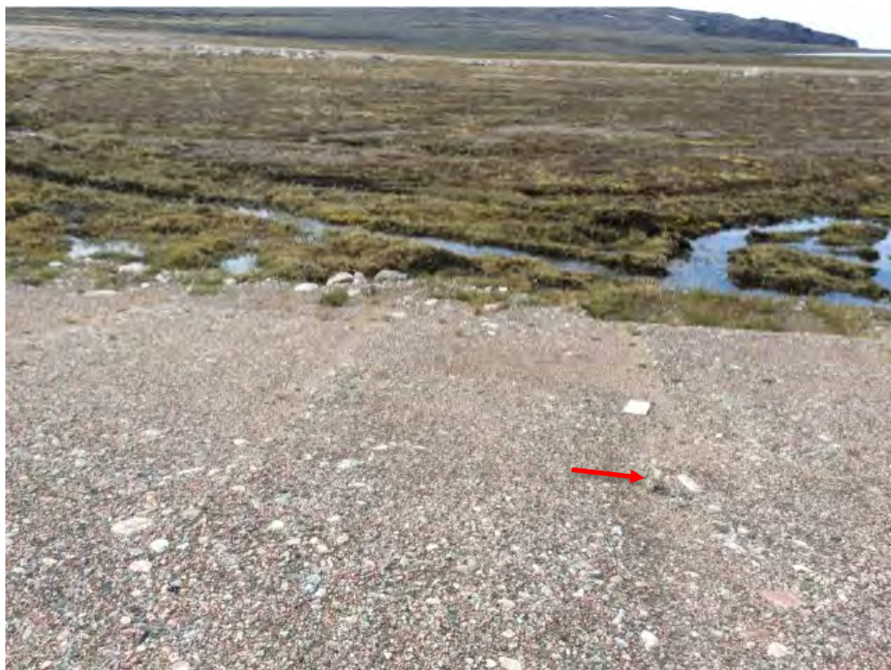
Photo 22: Lower Site Landfill South- West slope, Feature A3-Minor self-armouring erosion, facing southwest (Acceptable) (CAM5_Photo55.jpg)
