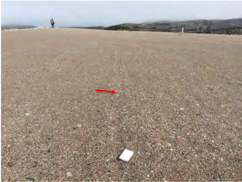
Photo 189: Tier II Disposal Facility- Cover surface, Feature E-Minor erosion channel, facing northeast (Acceptable) (CAM5_Photo5.jpg)
