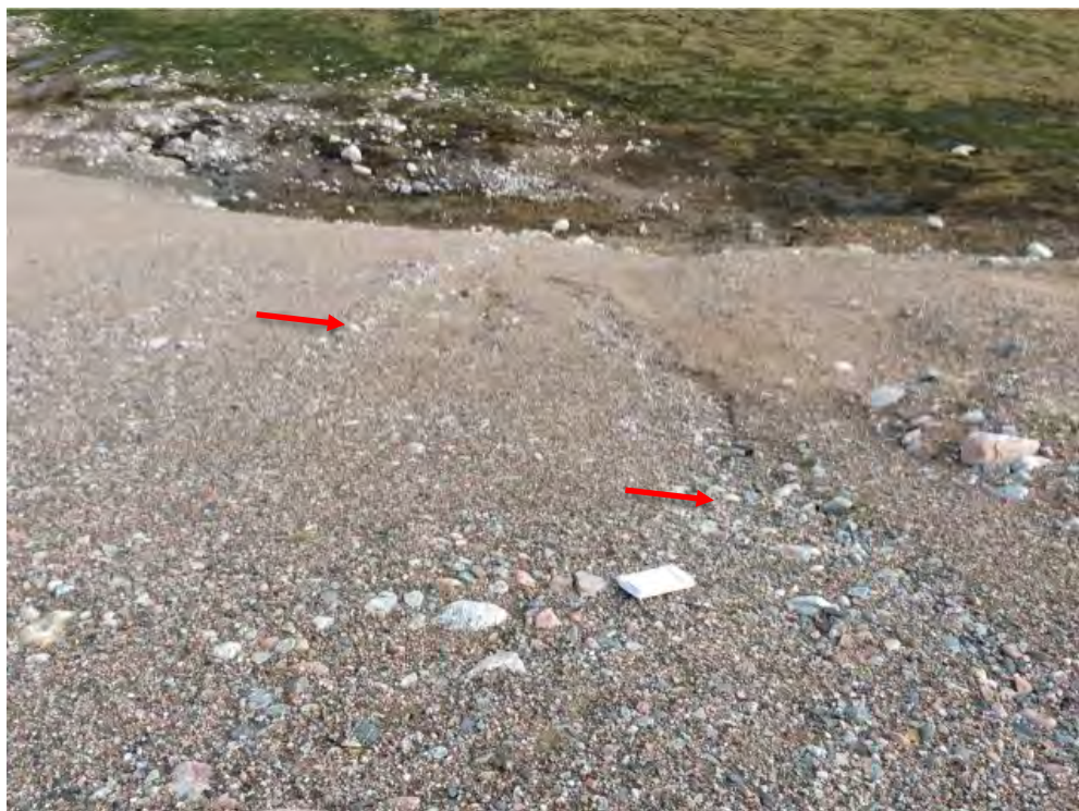
Photo 54: Lower Site Landfill South- East slope, Feature X-Minor self-armouring erosion, facing northeast (Acceptable) (CAM5_Photo73.jpg)
