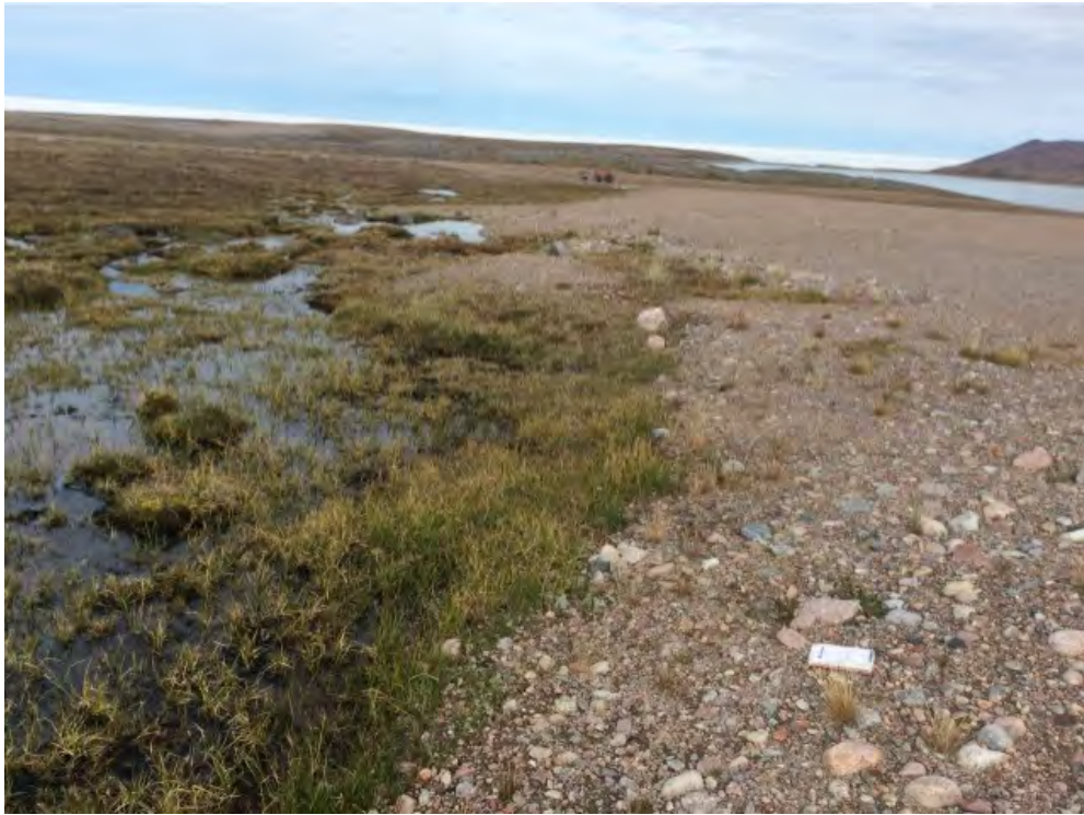
Photo 47: Lower Site Landfill South- Southwest toe, Feature Q1-Ponded water along toe, facing northwest (Acceptable) (CAM5_Photo61.jpg)
