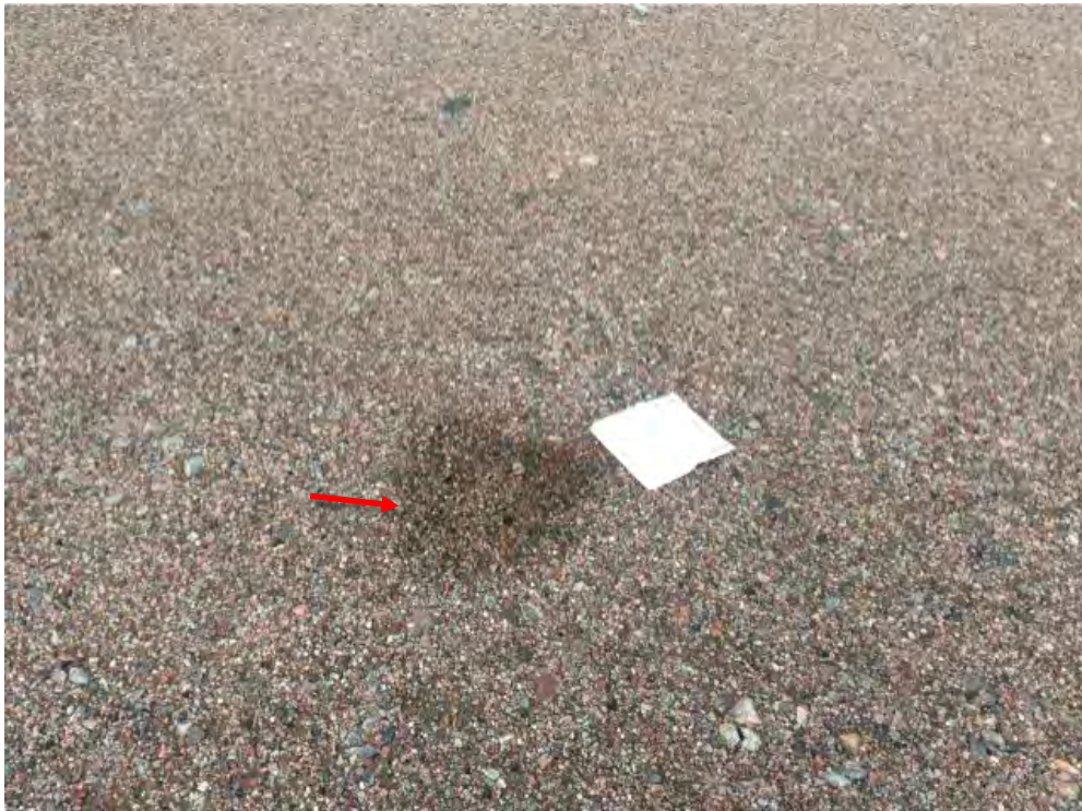
Photo 36: Lower Site Landfill South- Cover surface, Feature L-Small hydrocarbon stain (Acceptable) (CAM5_Photo71.jpg)
