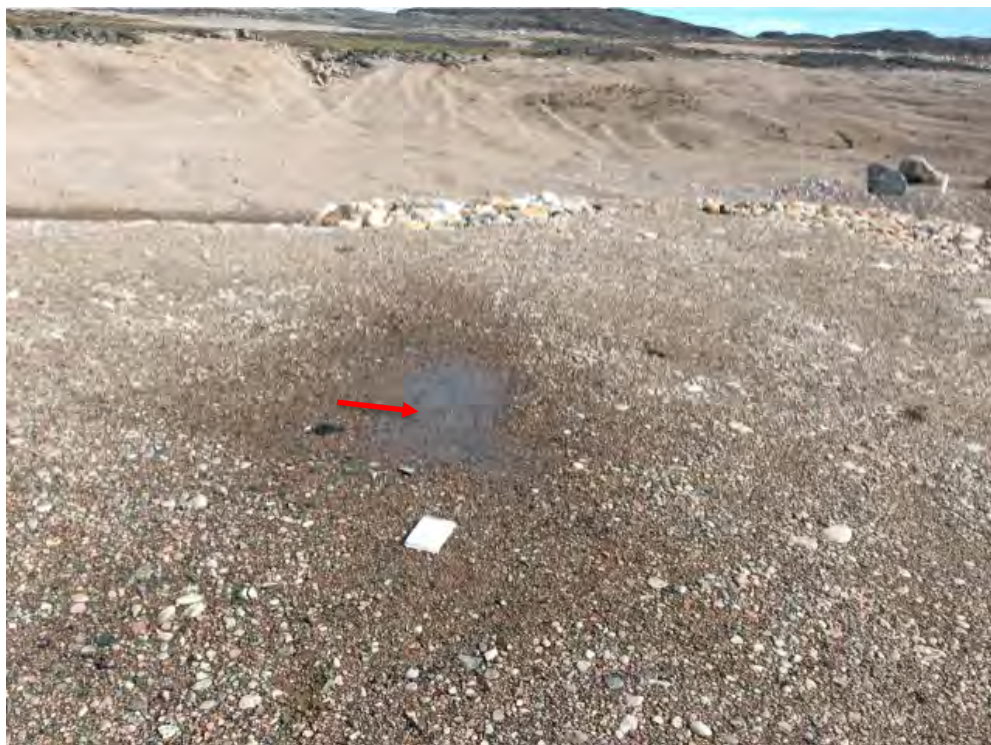
Photo 112: Non-Hazardous Waste Landfill- South east corner, Feature P-Ponded Water, facing east (Acceptable) (CAM5_Photo16.jpg)
