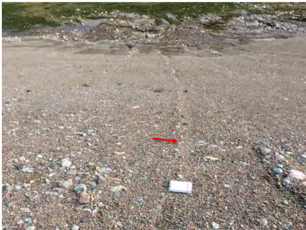
Photo 39: Lower Site Landfill South- East slope, Feature N-Minor erosion channel, facing northeast (Acceptable) (CAM5_Photo79.jpg)
