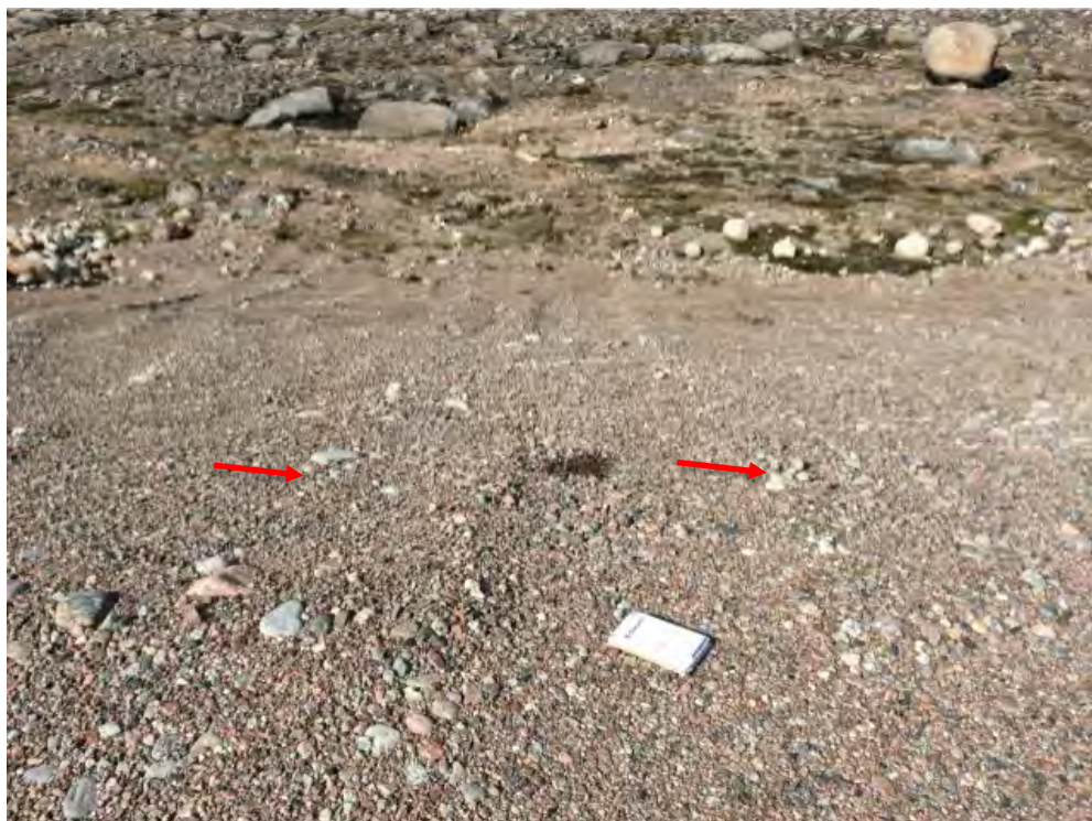
Photo 102: Non-Hazardous Waste Landfill- North slope, Feature K-Self-armouring erosion, facing northwest (Acceptable) (CAM5_Photo27.jpg)
