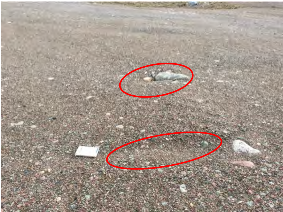
Photo 58: Lower Site Landfill South- Cover surface, Feature Z- Two small settlement areas, facing east (Acceptable) (CAM5_Photo68.jpg)
