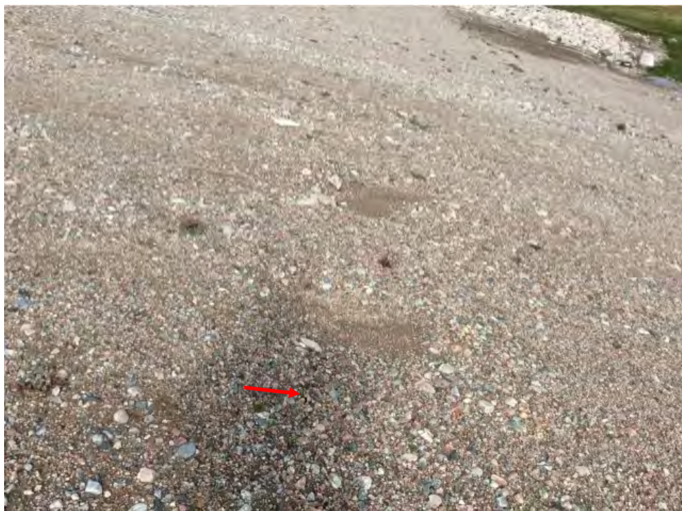
Photo 56: Lower Site Landfill South- East slope near crest, Feature Y-Crack on slope near crest, facing northwest (Acceptable) (CAM5_Photo86.jpg)
