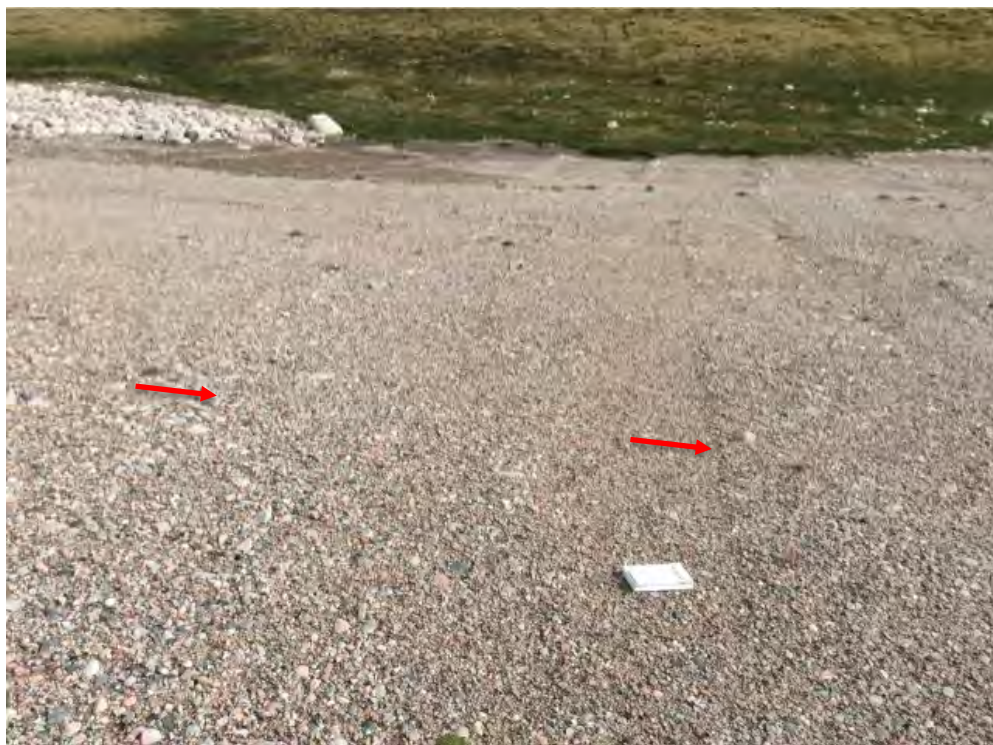
Photo 40: Lower Site Landfill South- East slope, Feature N-Minor self-armouring erosion, facing northeast (Acceptable) (CAM5_Photo89.jpg)
