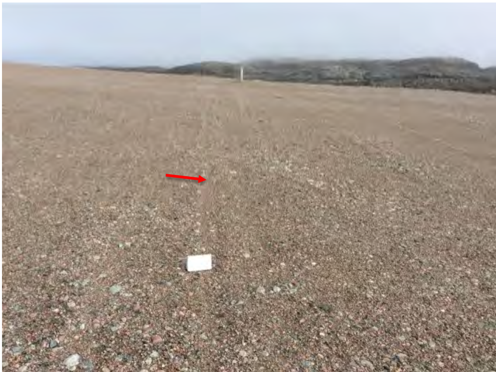
Photo 188: Tier II Disposal Facility- Cover surface, Feature E-Minor erosion channel, facing northeast (Acceptable) (CAM5_Photo6.jpg)
