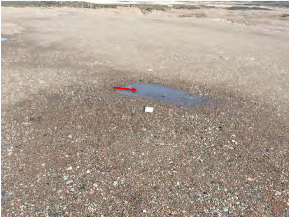
Photo 115: Non-Hazardous Waste Landfill- Cover surface, Feature P-Ponded water, facing east (Acceptable) (CAM5_Photo29.jpg)
