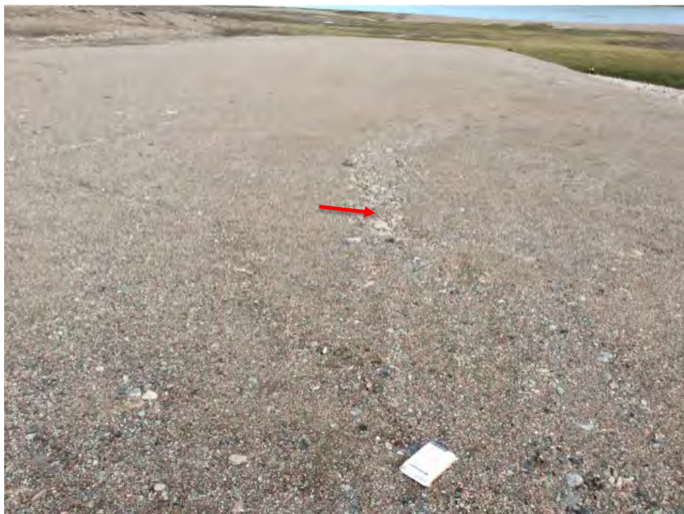
Photo 60: Lower Site Landfill South- Cover surface, Feature J -Self armouring erosion along northeast crest, facing northwest (CAM5_Photo76.jpg)
