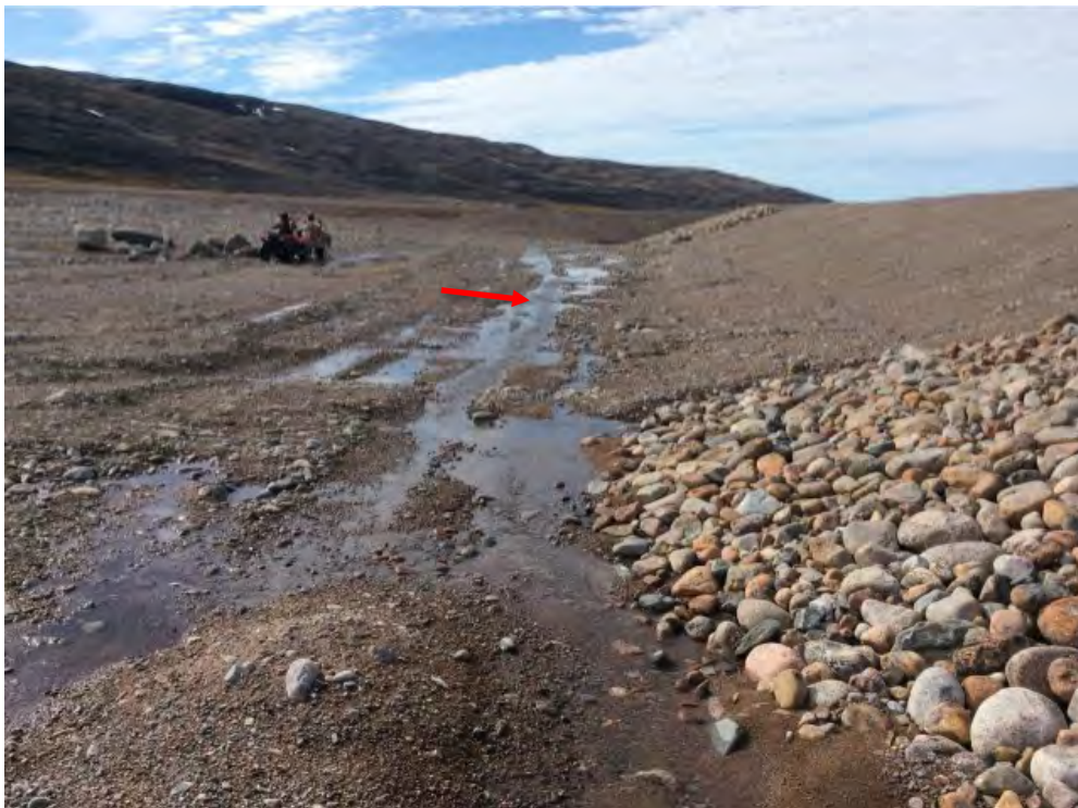
Photo 94: Non-Hazardous Waste Landfill- South toe, Feature E-Running water along toe, facing southwest (Acceptable) (CAM5_Photo12.jpg)
