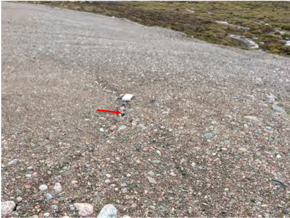
Photo 57: Lower Site Landfill South- West slope, Feature V3- Minor self-armouring erosion with new infilled cracking, facing southeast (Acceptable) (CAM5_Photo63.jpg)
