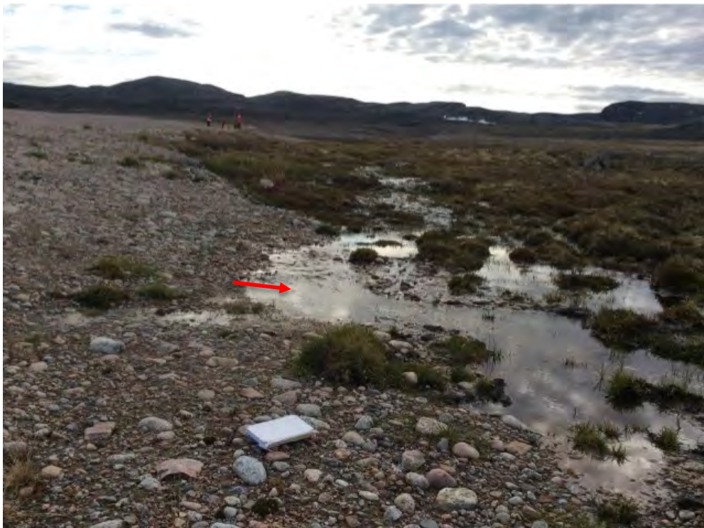
Photo 44: Lower Site Landfill South- Southwest toe, Feature Q1-Ponded water along toe, facing southeast (Acceptable) (CAM5_Photo58.jpg)
