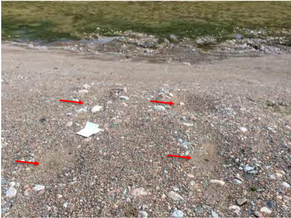
Photo 37: Lower Site Landfill South- East crest, Feature M-Minor settlement depressions, facing northeast (Acceptable) (CAM5_Photo77.jpg)
