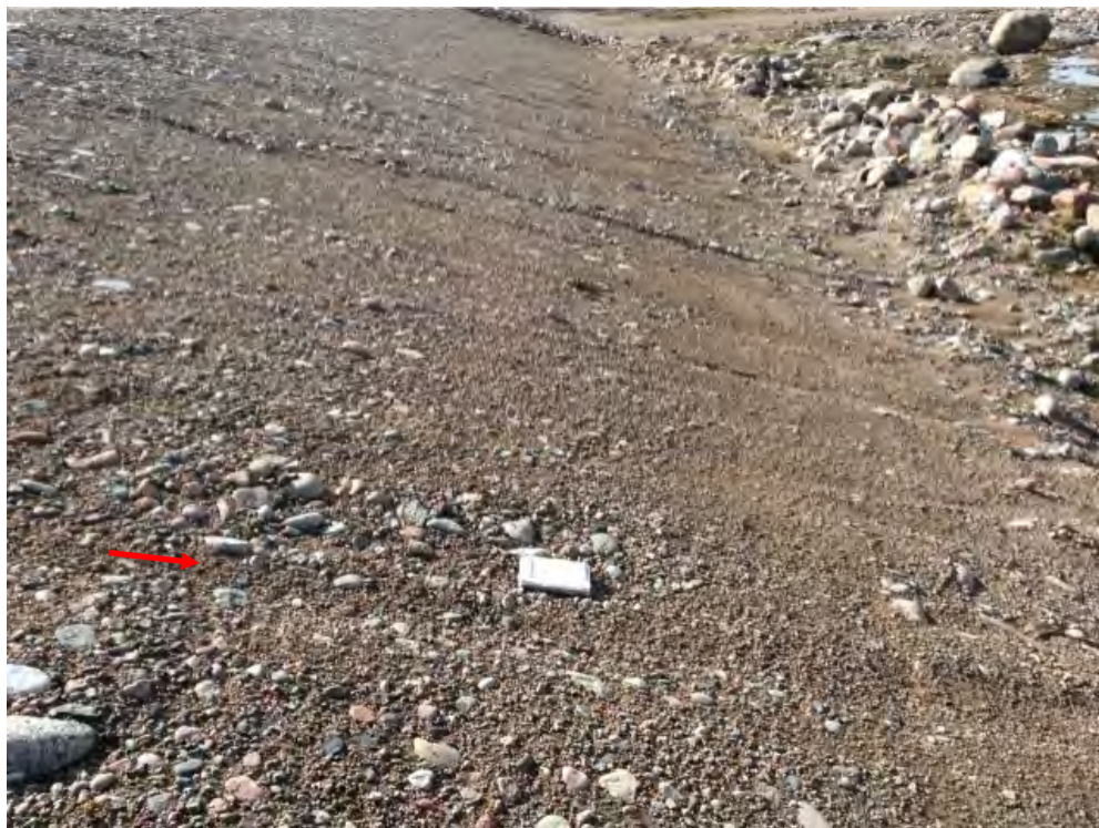
Photo 91: Non-Hazardous Waste Landfill- North slope, Feature B-Self-armouring erosion, facing southwest (Acceptable) (CAM5_Photo24.jpg)
