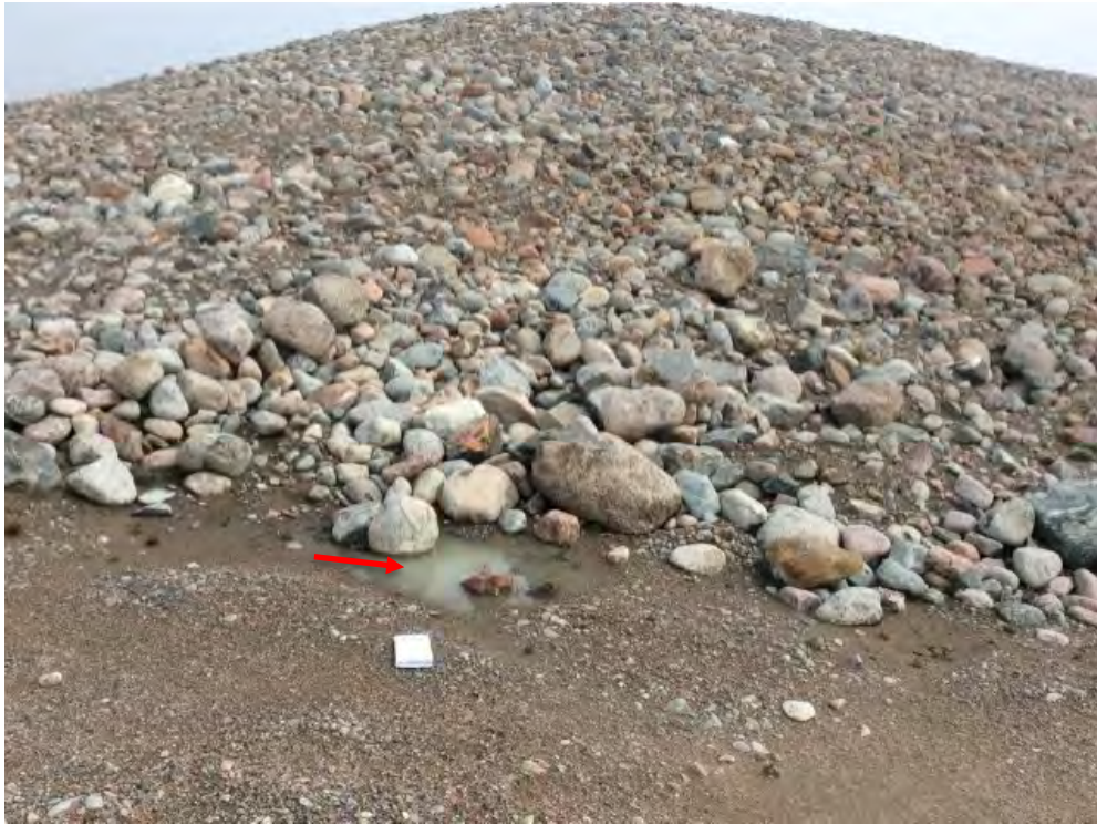
Photo 193: Tier II Disposal Facility- West toe corner, Feature H-Small ponded water, facing east (Acceptable) (CAM5_Photo2.jpg)
