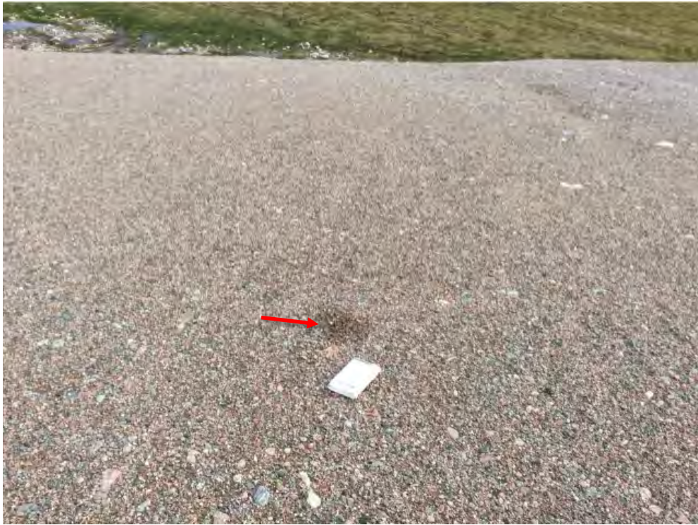
Photo 35: Lower Site Landfill South- Cover surface, Feature L-Small hydrocarbon stain, facing northeast (Acceptable) (CAM5_Photo72.jpg)
