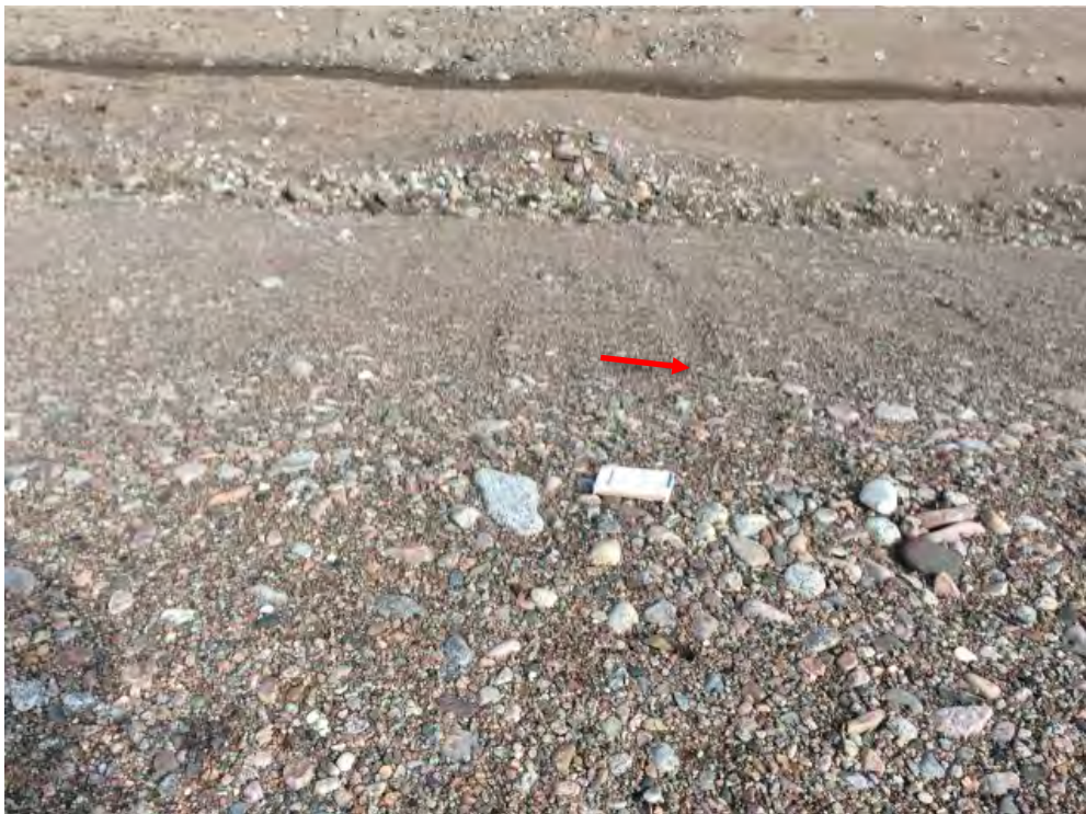
Photo 106: Non-Hazardous Waste Landfill- East slope, Feature L-Self-armouring erosion, facing northeast (Acceptable) (CAM5_Photo21.jpg)
