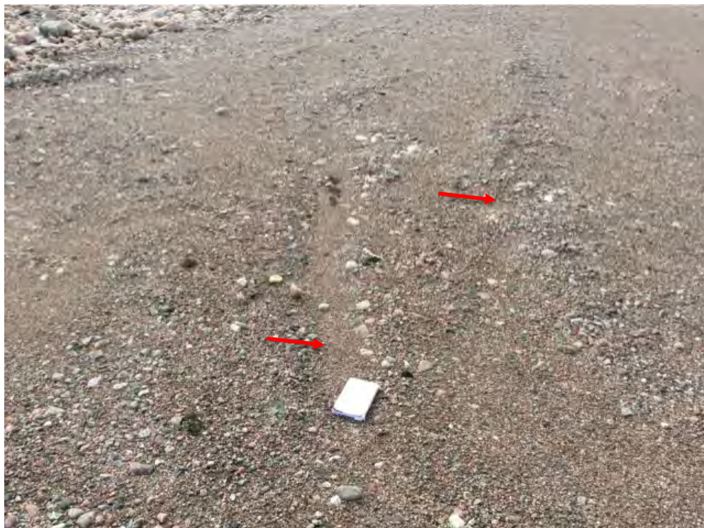
Photo 145: USAF & Asbestos Landfill- Southeast crest surface, Feature E-Vehicle rutting with minor erosion, facing northwest (Acceptable) (CAM5_Photo37.jpg)
