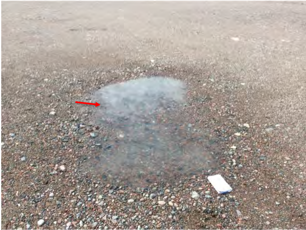
Photo 93: Non-Hazardous Waste Landfill- South crest surface, Feature D-Minor settlement with ponded water, facing east (Acceptable) (CAM5_Photo33.jpg)
