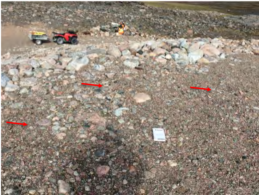
Photo 184: Tier II Disposal Facility- Northeast crest surface, Feature A-Minor depressions, facing north (Acceptable) (CAM5_Photo10.jpg)
