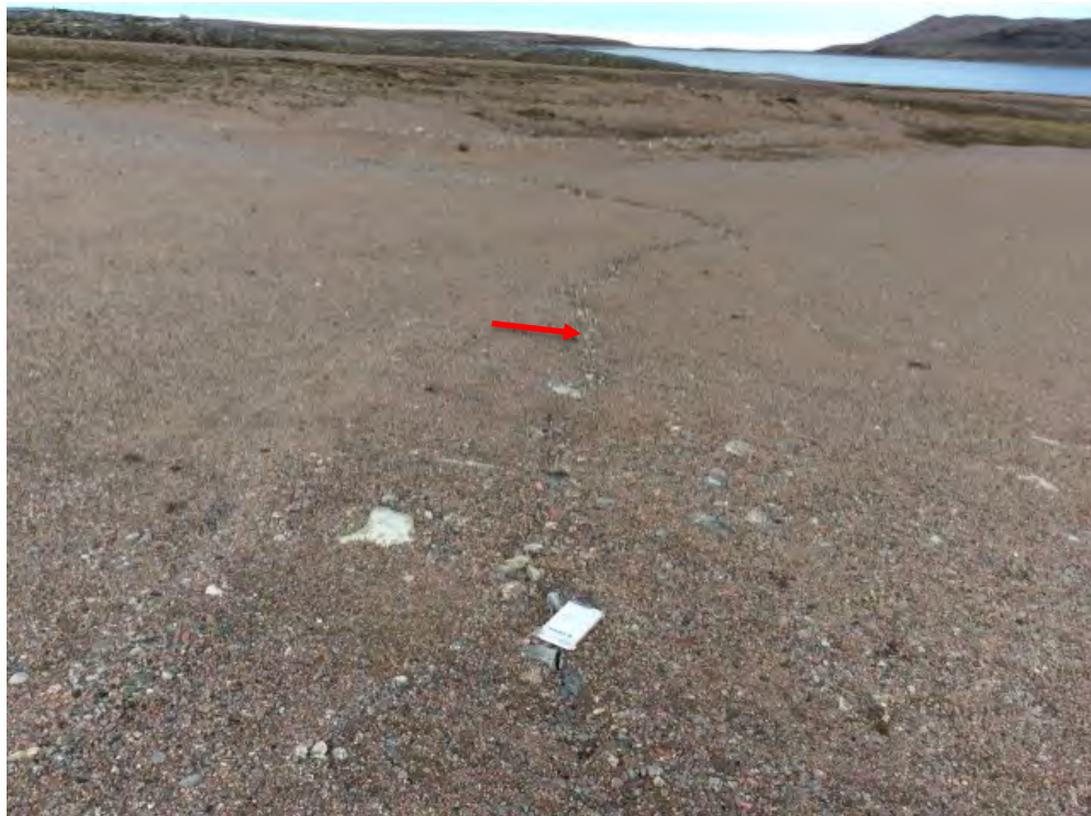
Photo 55: Lower Site Landfill South- Northwest crest and slope, Feature S-Crack and erosion channel, facing northwest (Acceptable) (CAM5_Photo75.jpg)
