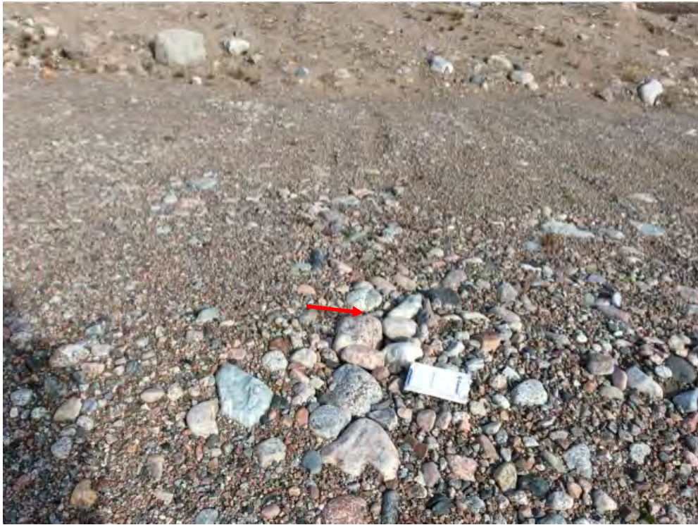
Photo 105: Non-Hazardous Waste Landfill- East slope, Feature L-Self-armouring erosion, facing northeast (Acceptable) (CAM5_Photo22.jpg)
