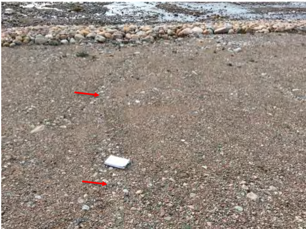
Photo 156: USAF & Asbestos Landfill- West crest, Feature P -Self armouring erosion, facing southwest (CAM5_Photo41.jpg)
