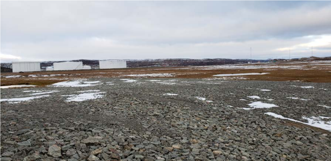
Photo 7: Secondary capped area – Vehicle Storage Area. (looking southeast)
