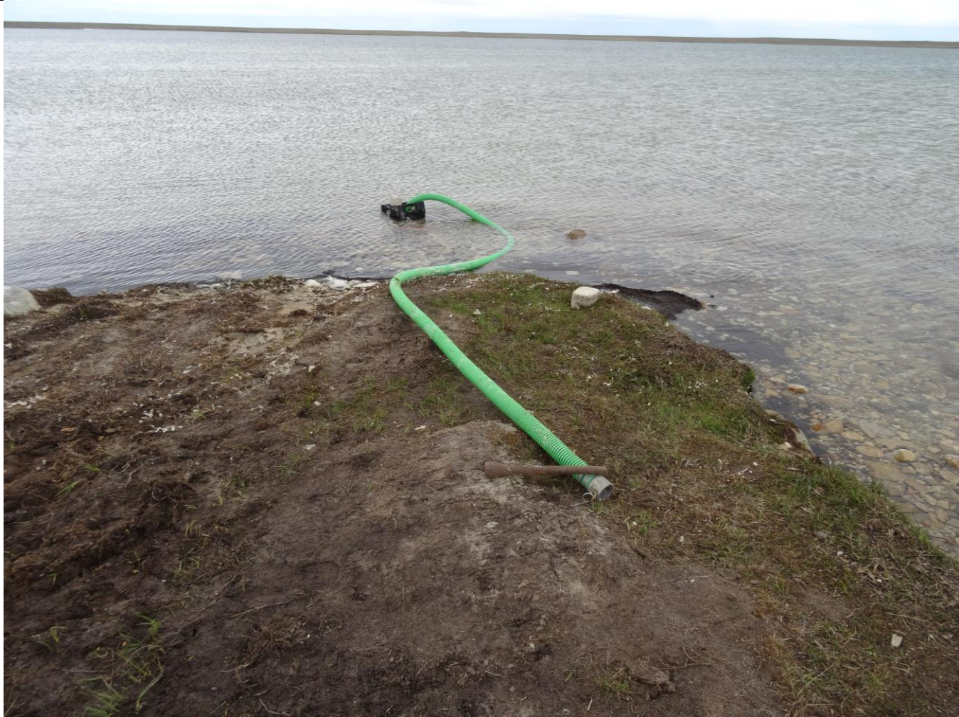
Description: Raw Water Intake Hose at Water Lake – NO SIGNAGE
