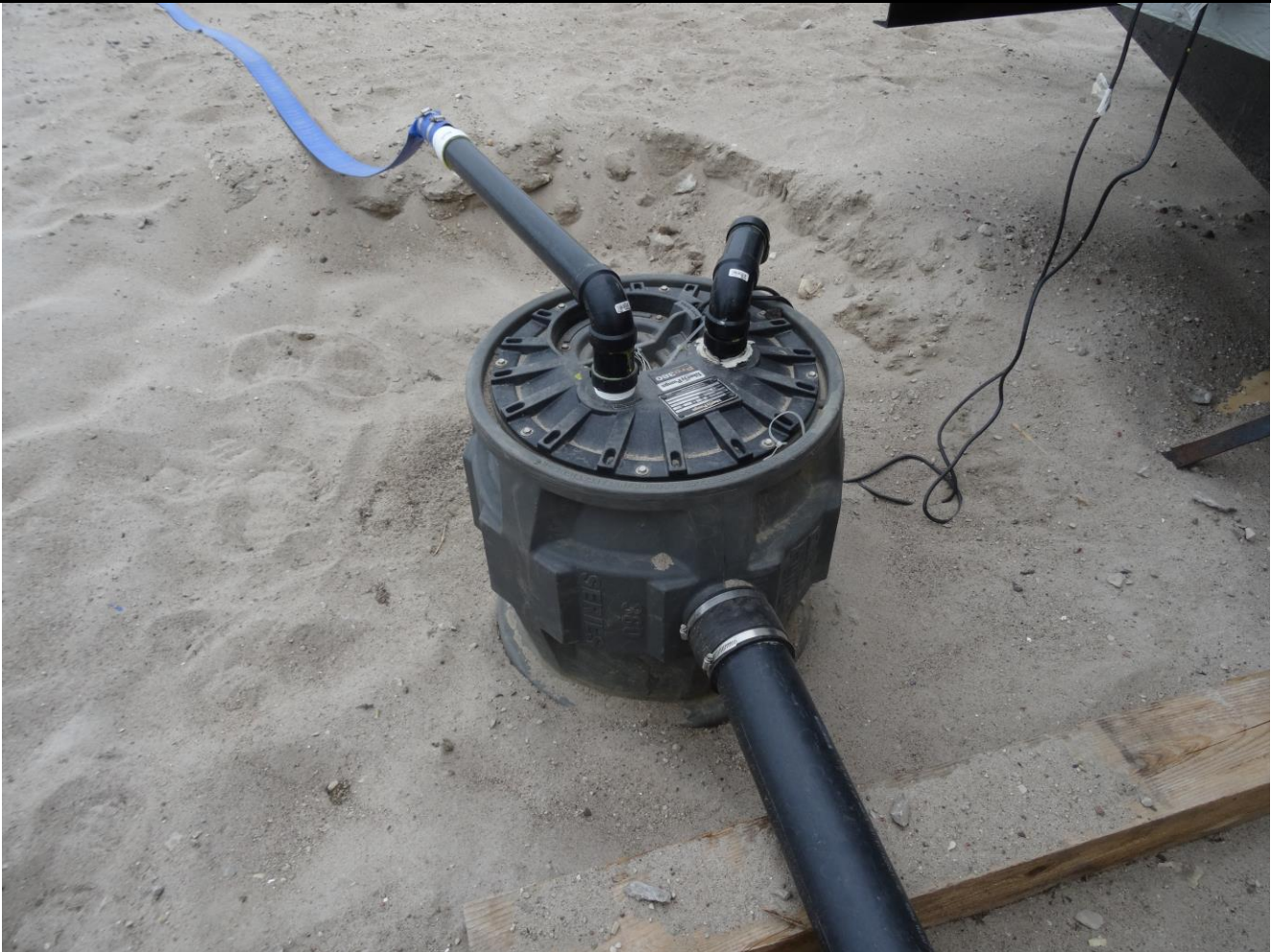
Description: Grey/Black Water Pump/Mulcher
