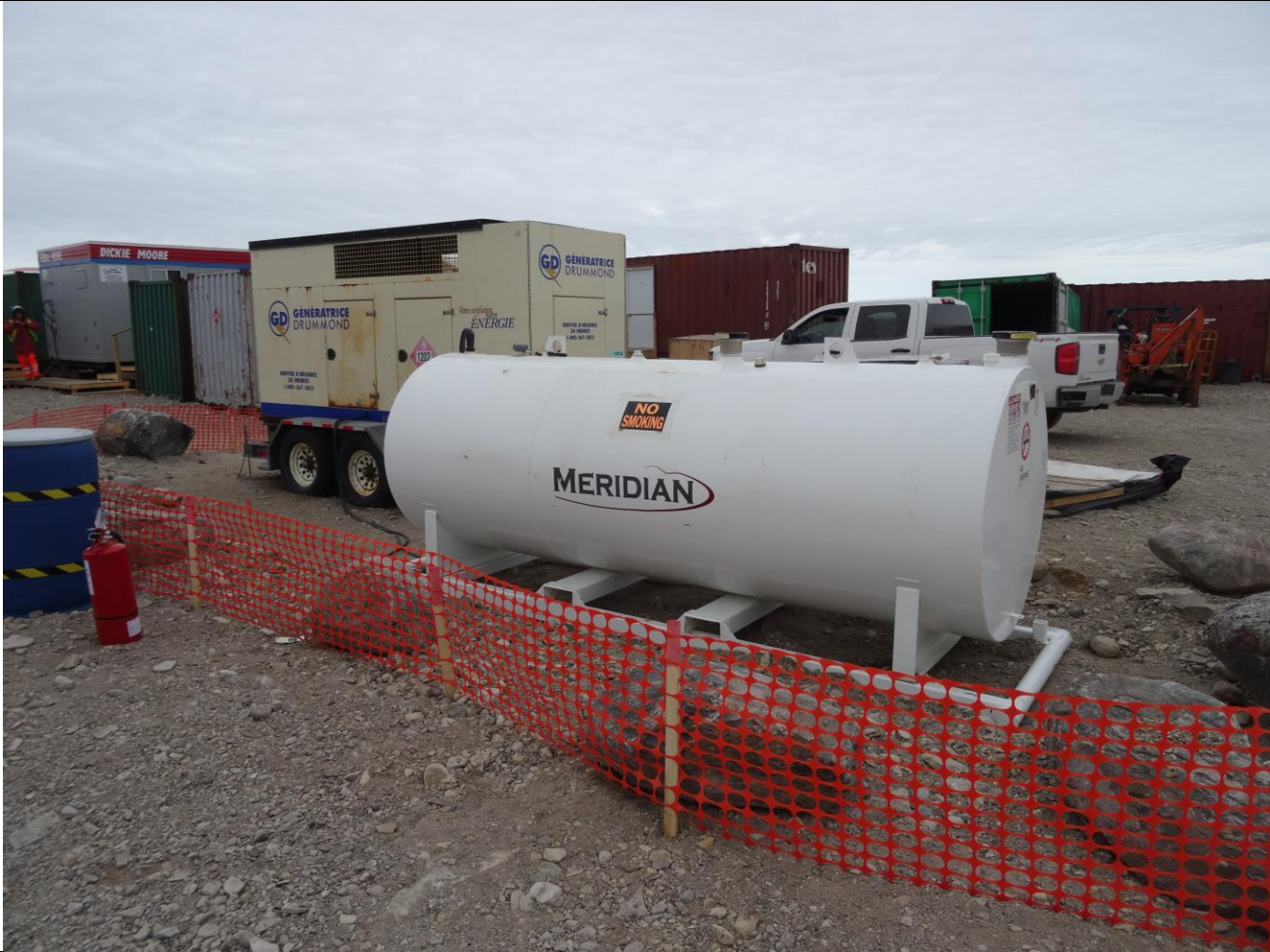
Description: Double Walled Fuel Tank and Camp Generator
