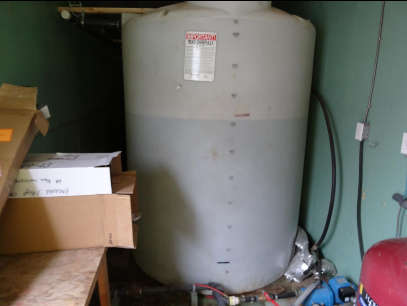
Description: Raw Water Storage Tank – 1 of 5 inside Sea Can Container
