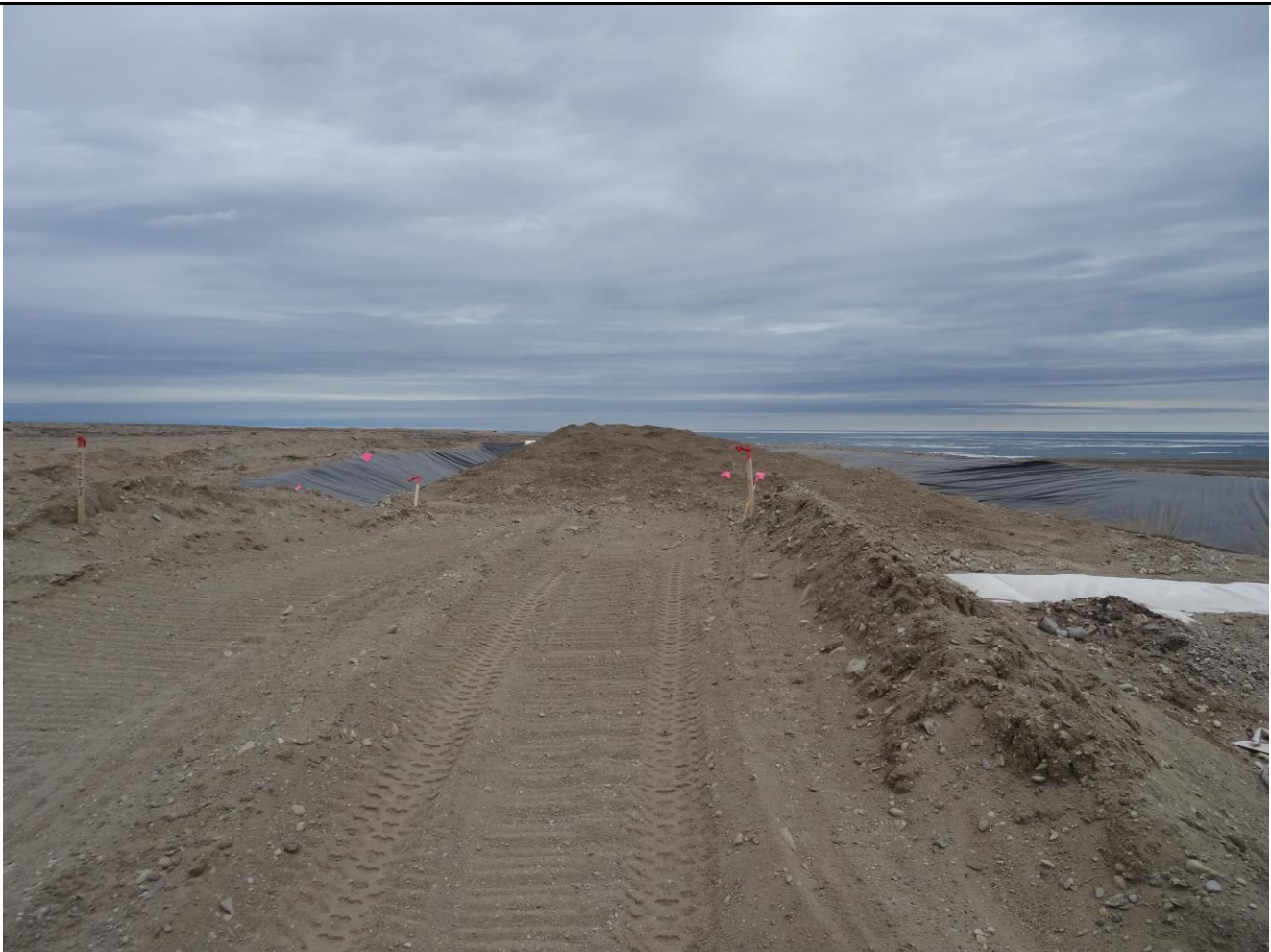
Description: Land Farm Treatment Area – Lined and Bermed
