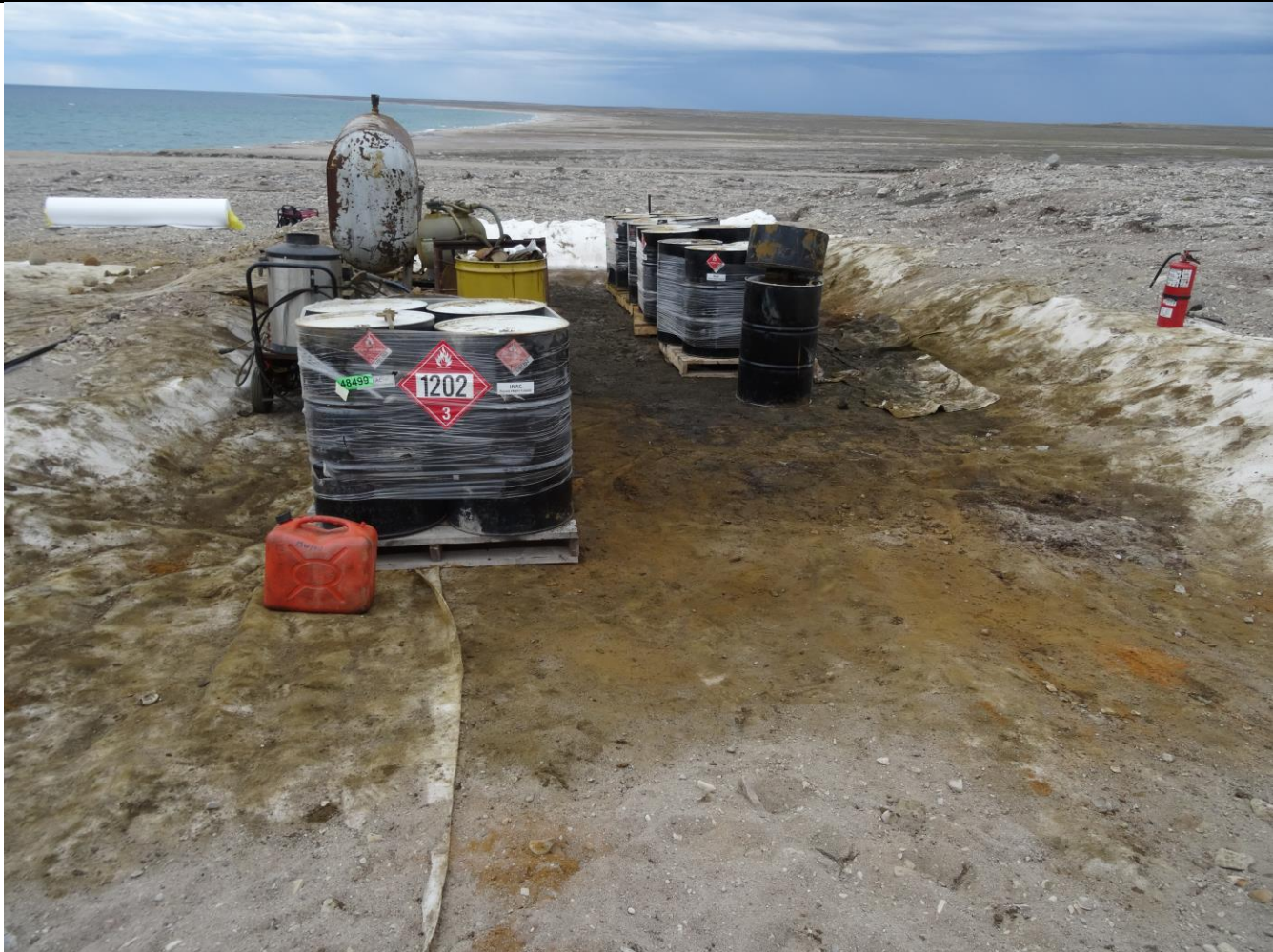
Description: Barrel Processing Area – Lined and Bermed
