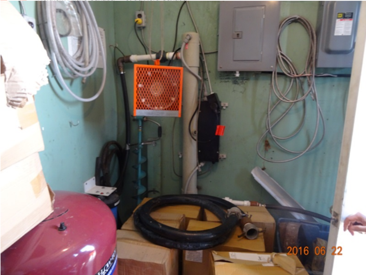
Figure 11 Sand filters and UV water treatment
