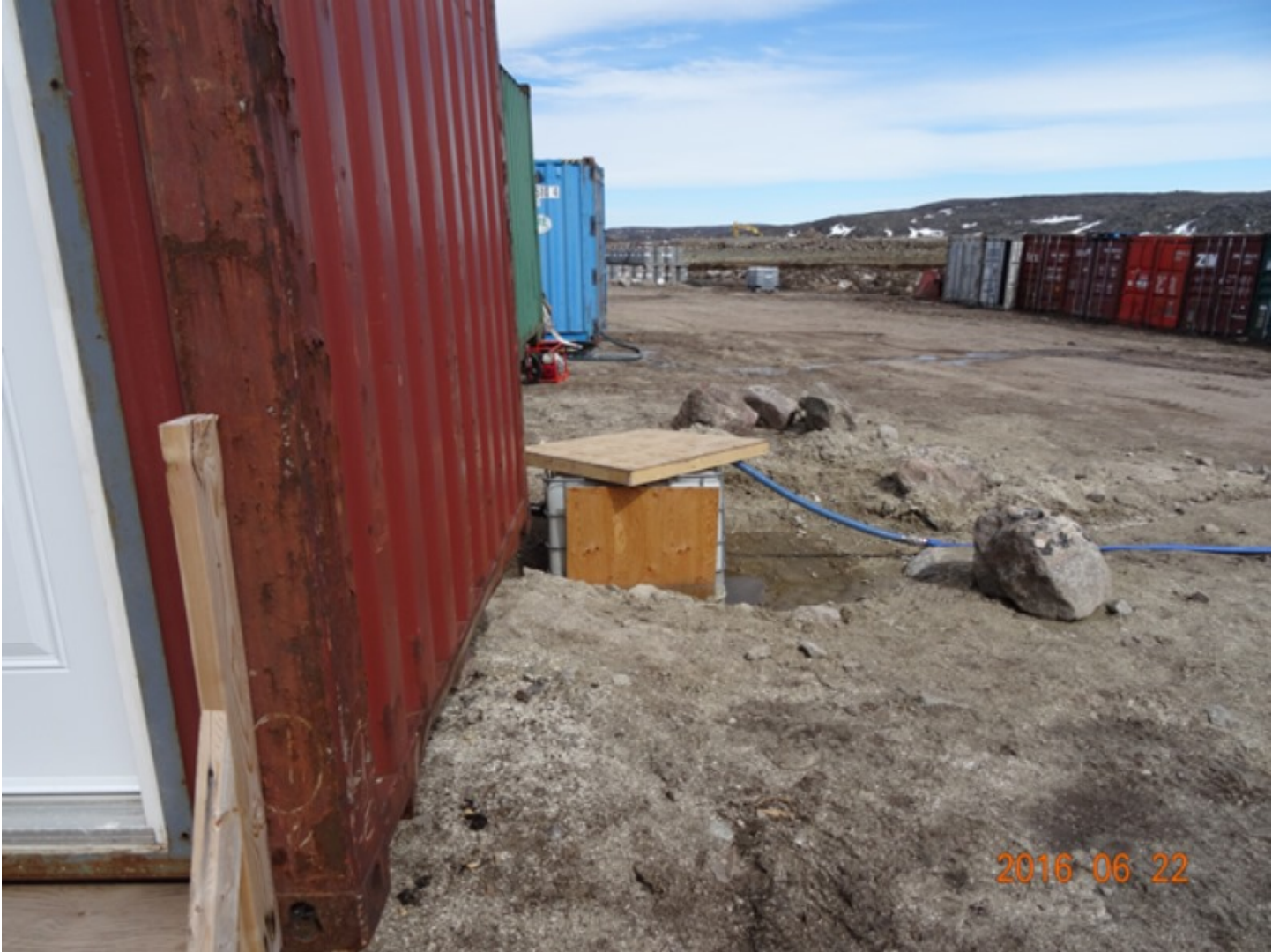
Figure 13 wastewater collection point for discharge to lagoon.
