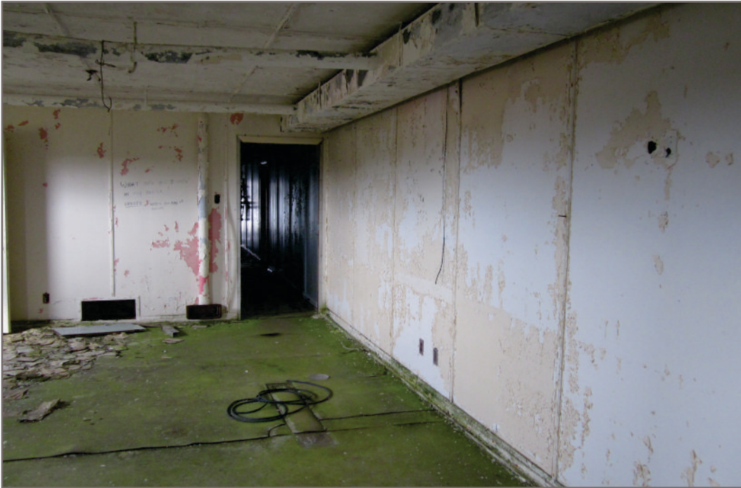
Photo H-13: Example of total and leachable lead painted ACM panels and wood (APEC 9 - Bunkhouse shown)
