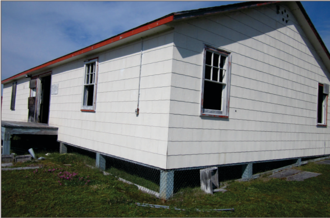
Photo H-1: Example of exterior ACM siding and total and leachable lead paint on wood (APEC 1 - Storage Shed 01 shown)
