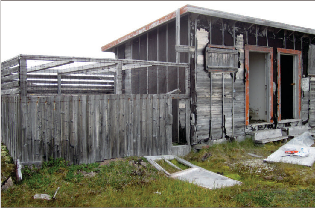
Photo H-11: Example of ACM shingles and total and leachable lead painted wood (APEC 8 - Chicken Coop shown)
