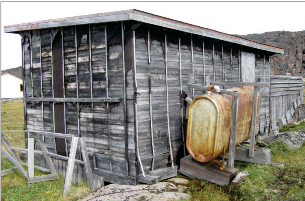
Photo H-12: Example of ASTs with organic liquid found on-site
