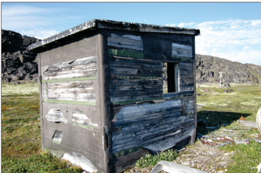
Photo H-8: Example of ACM green shingles on walls and roof (APEC 6 - Storage Shed 02)
