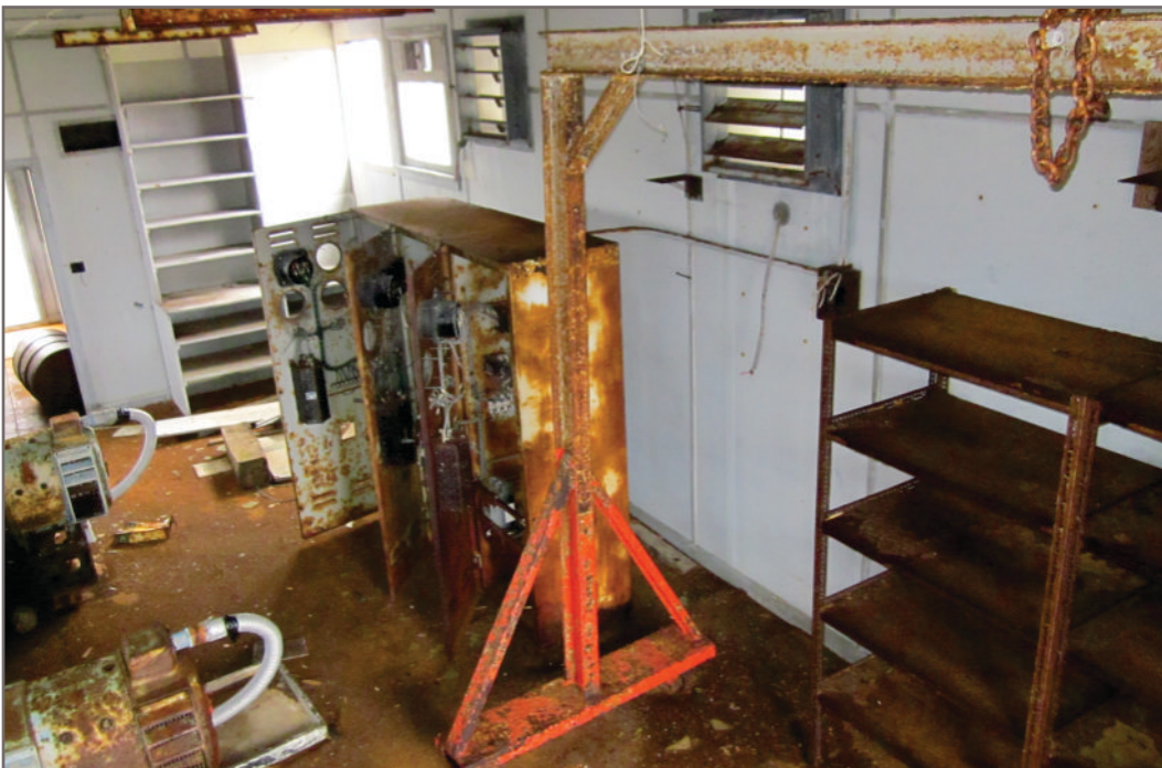
Photo H-14: APEC 10 - Generator Building – Mercury, PCBs and lead in electrical components, PCBs in light ballasts and mercury vapor in fluorescent lights
