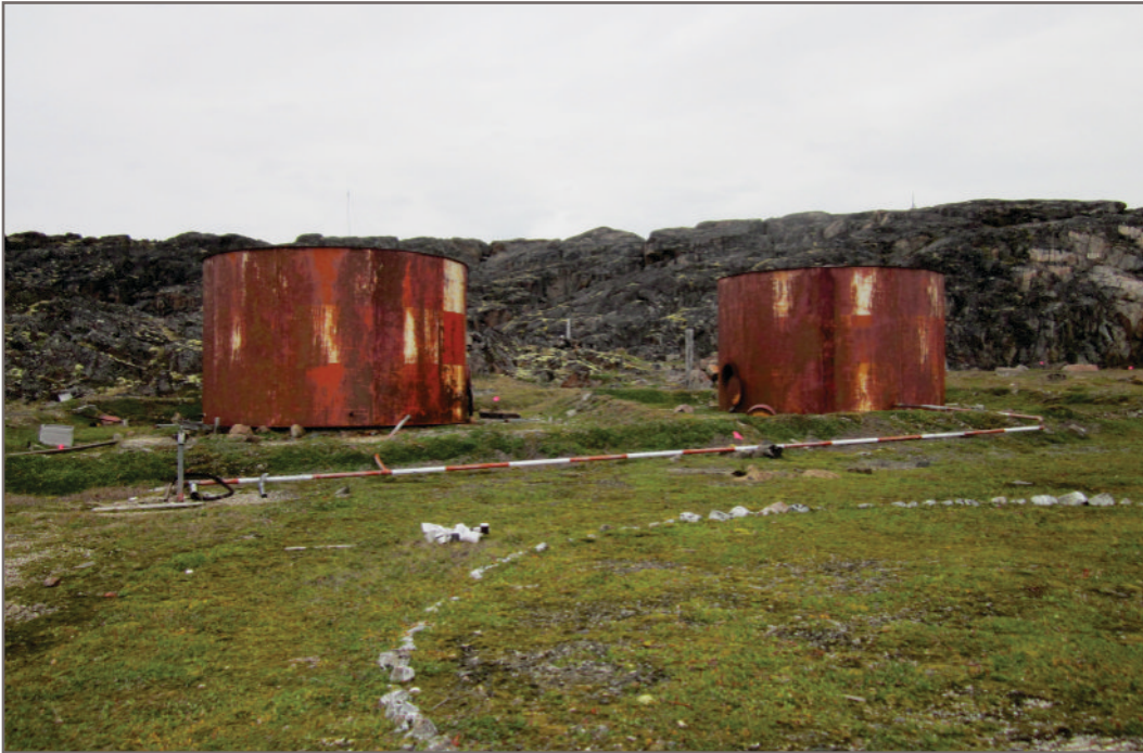
Photo H-17: APEC 14 - AST Tank Farm - Total lead painted ASTs
