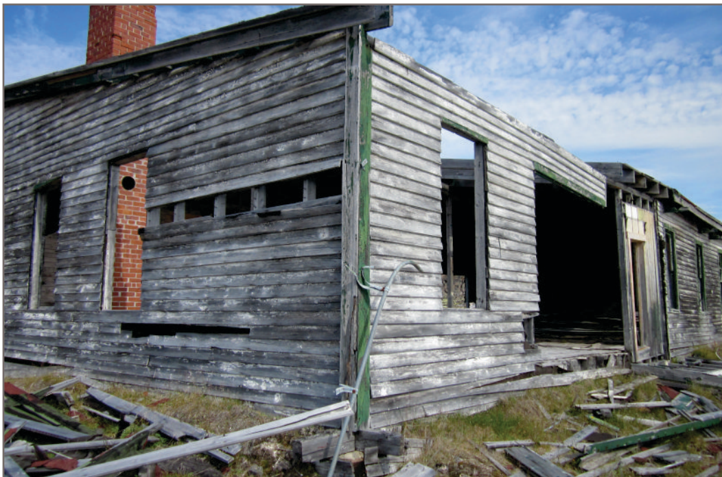
Photo H-3: Example of total and leachable lead paint on exterior and some interior wood (APEC 2 - Old Kitchen)
