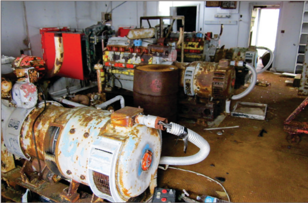
Photo H-15: APEC 10 - Generator Building - Total lead painted generators and equipment contents in three generators, lead acid batteries and total and leachable lead painted ACM panels
