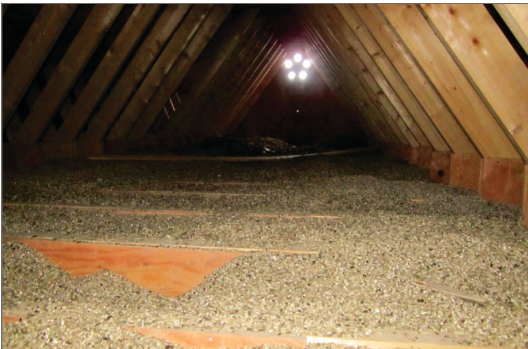
Photo H-2: Example of ACM attic insulation and fibreglass wall insulation is ACM contaminated from the attic (APEC 1 - Storage Shed 01 shown)
