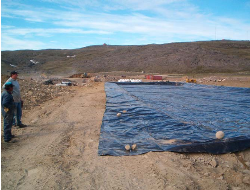
Photograph 3: 30 mil HDPE geomembrane over contour berms
