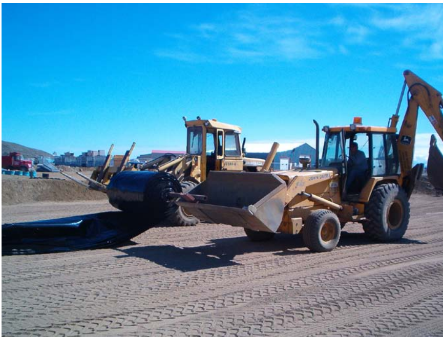
Photograph 2: Cell 3 surface smoothness and geomembrane deployment
