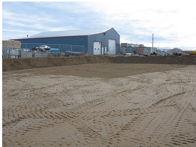
Prior to putting down liner floor of cell was hand raked to remove sharp stones and to smooth out the transition from walls to floor
