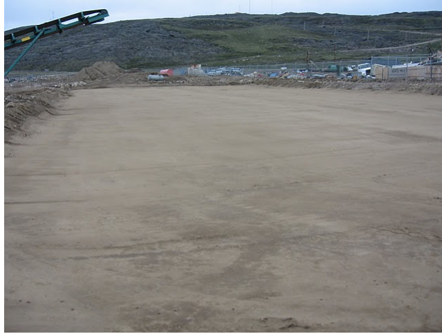
Site levelled stones packed and sand layer in place and packed.
