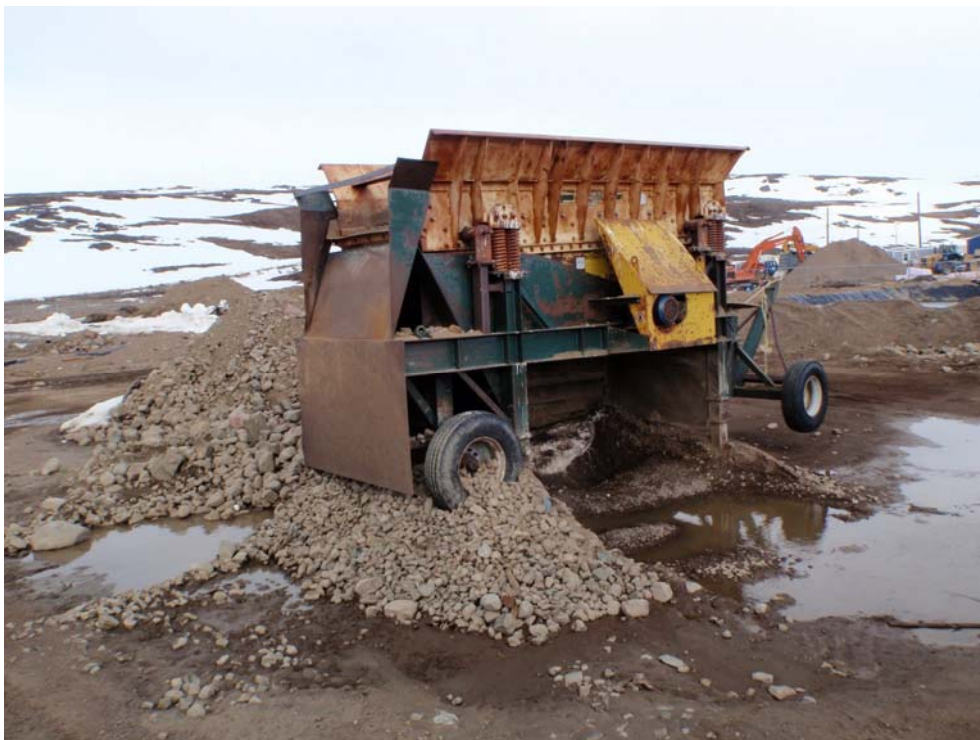
Shaker used to remove stone greater than 2 inch
