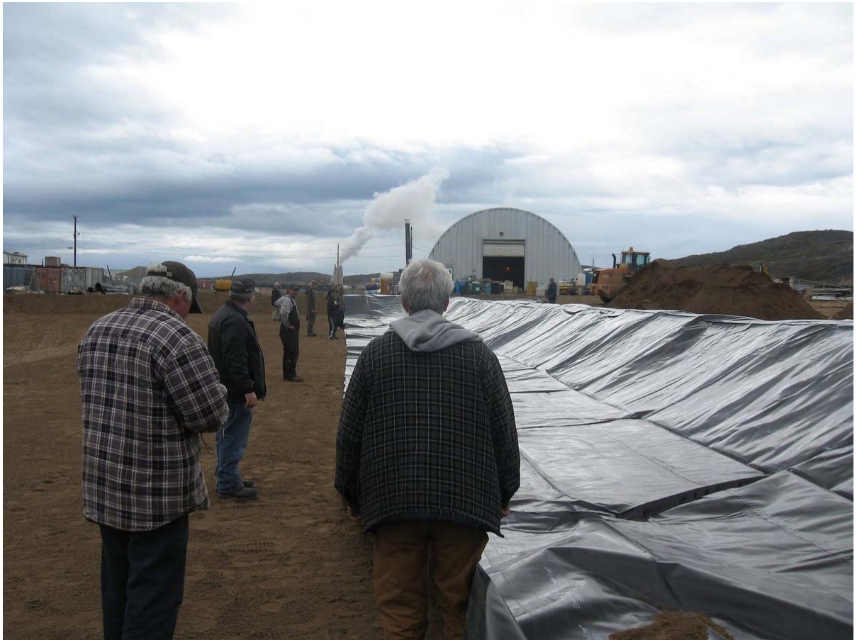
First couple folds out. Takes many hands to pull liner evenly into position.
