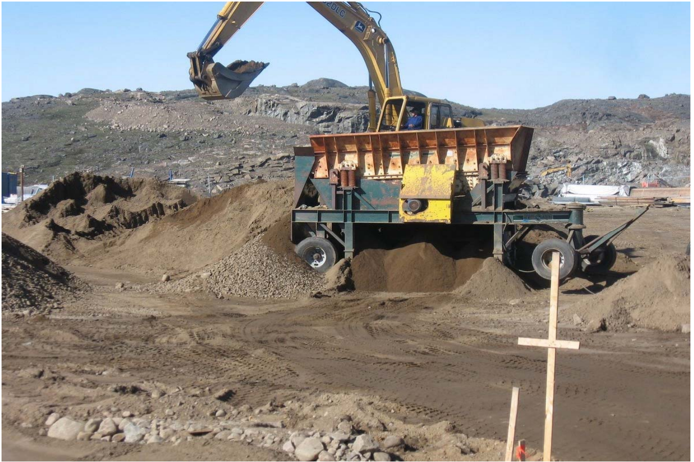
Sand was brought in and put through a shaker to remove all rocks down to less than \frac{1}{2} inch
