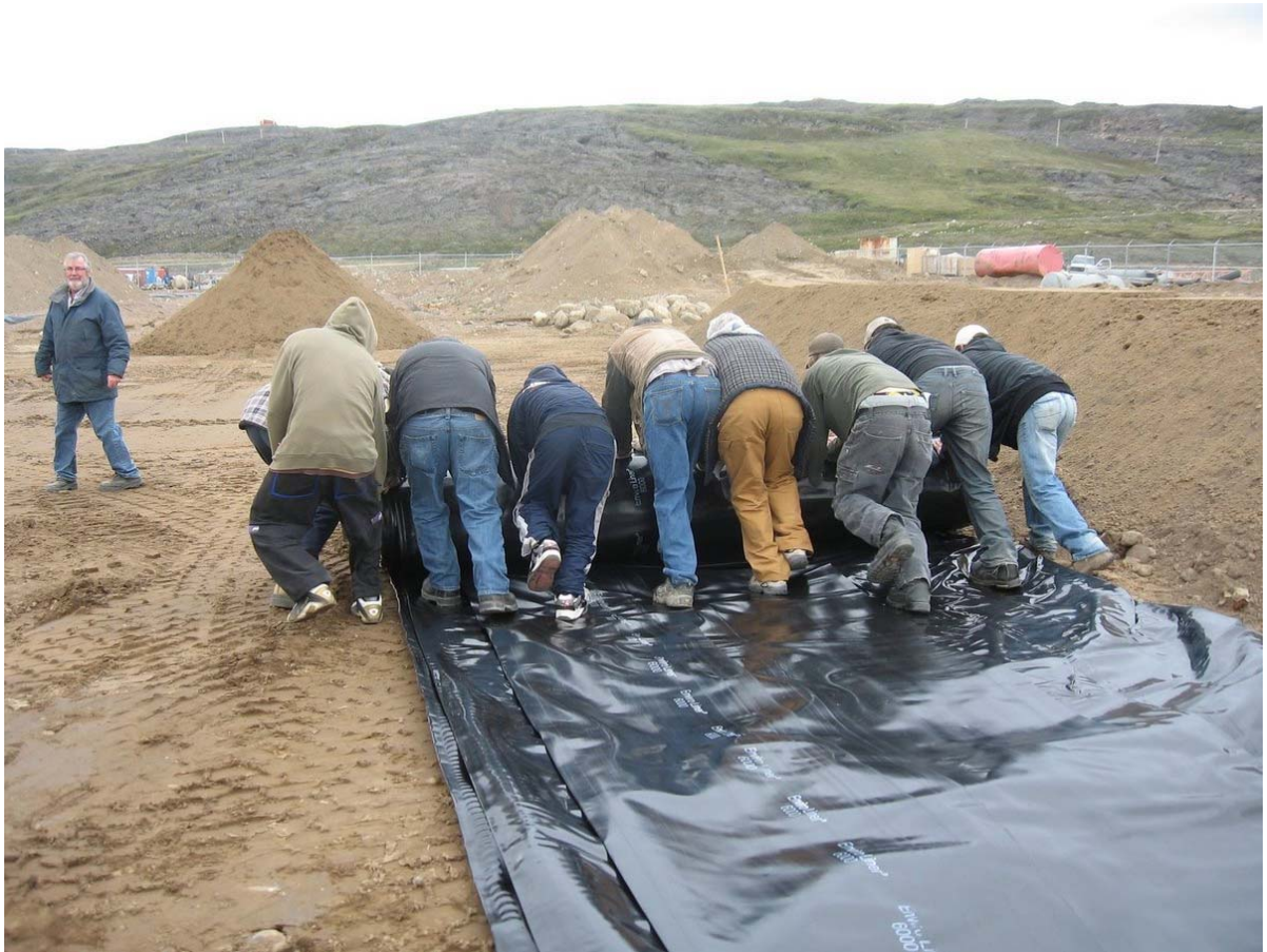
Unrolling of liner prior to unfolding across the width of the cell area
