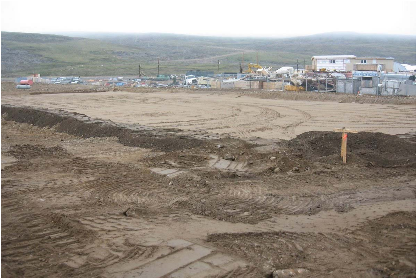
Walls were constructed of waste rocks in bottom and soils that pack on top to make for firm walls
