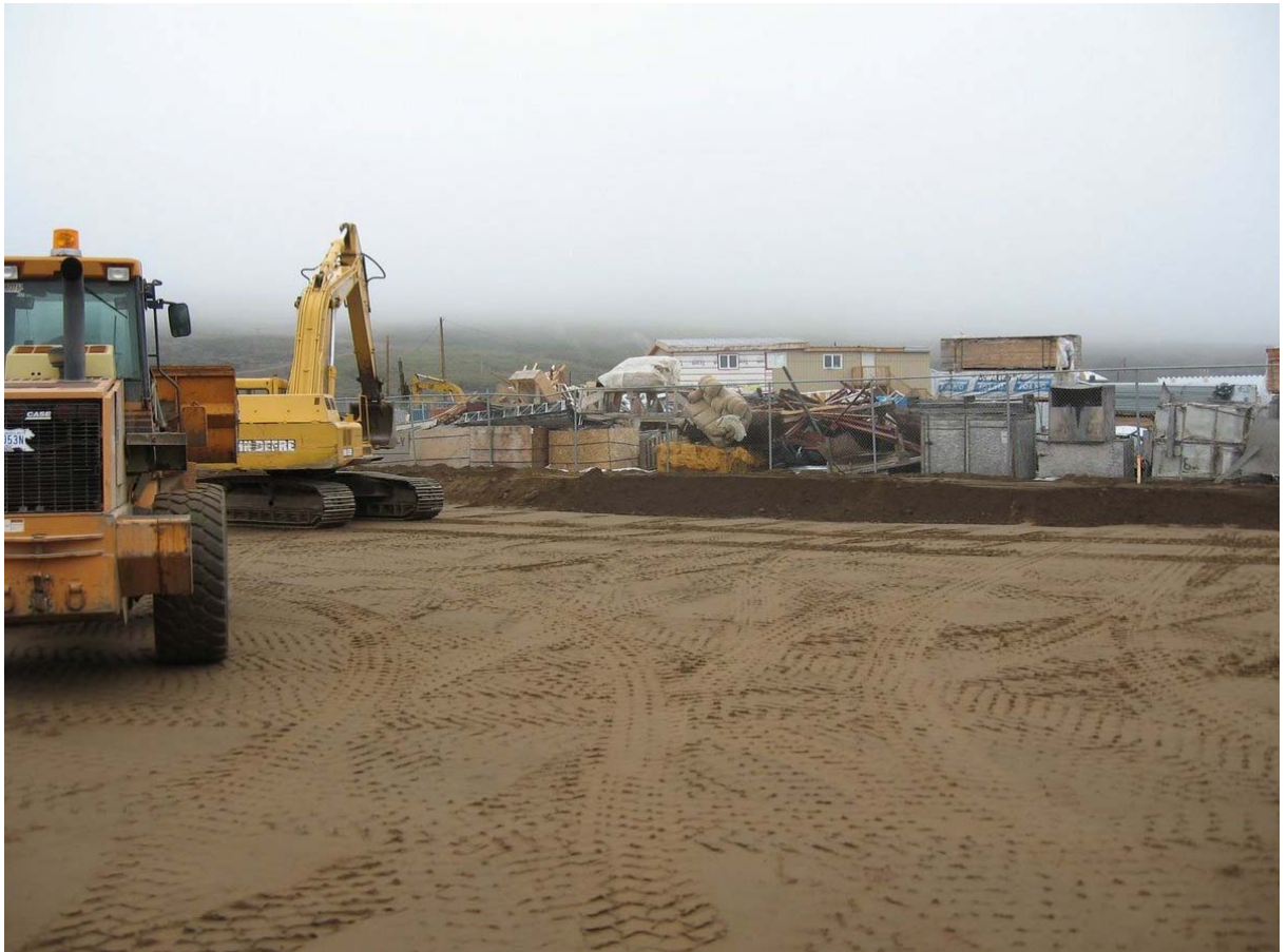
Excavator and loader used to carry materials and to pack walls tight
