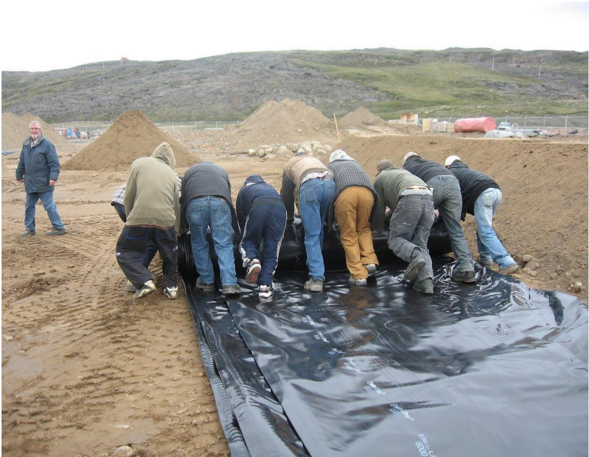
Unrolling of liner prior to unfolding across the width of the cell area
