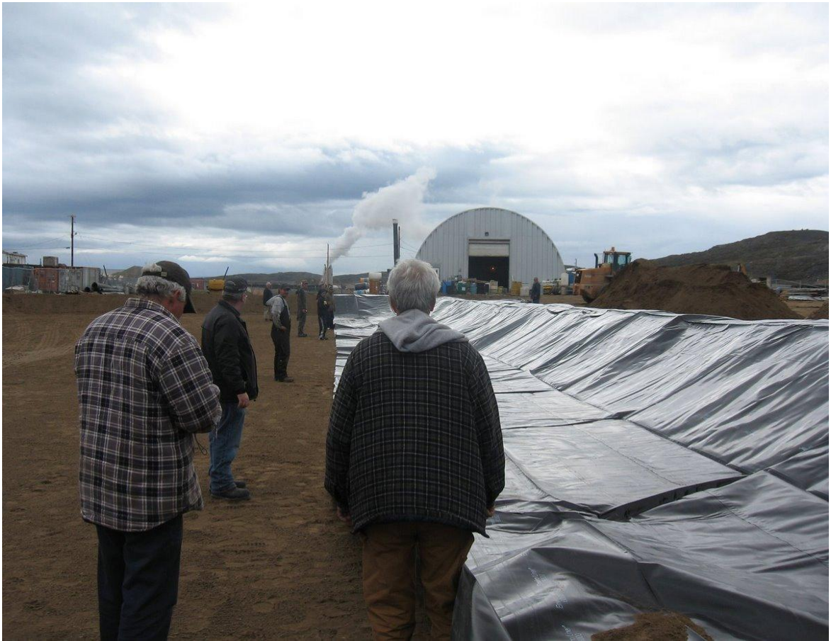
First couple folds out. Takes many hands to pull liner evenly into position.
