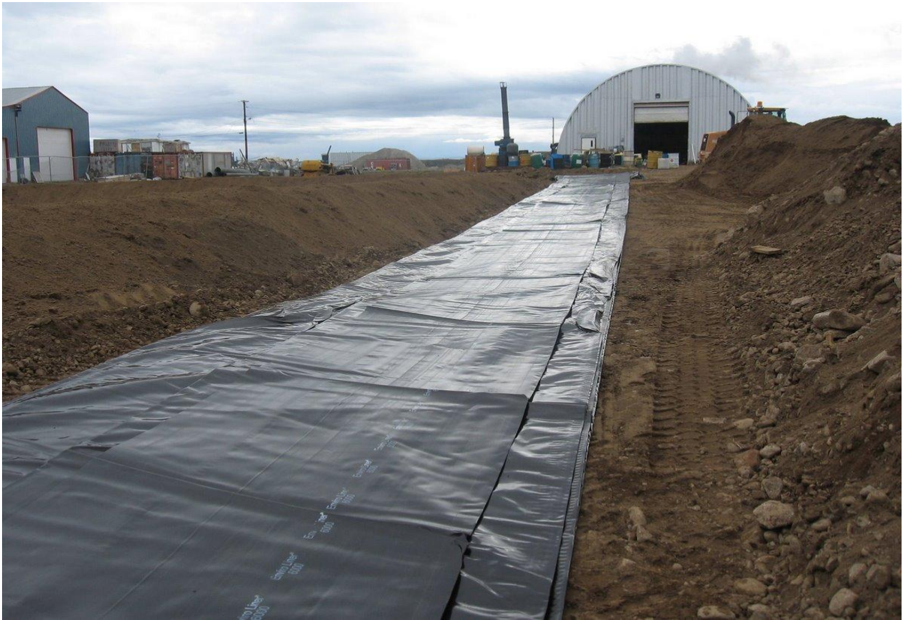
Shows length of cell area, liner unrolled and ready to unfold across the cell wall (left on photo)
