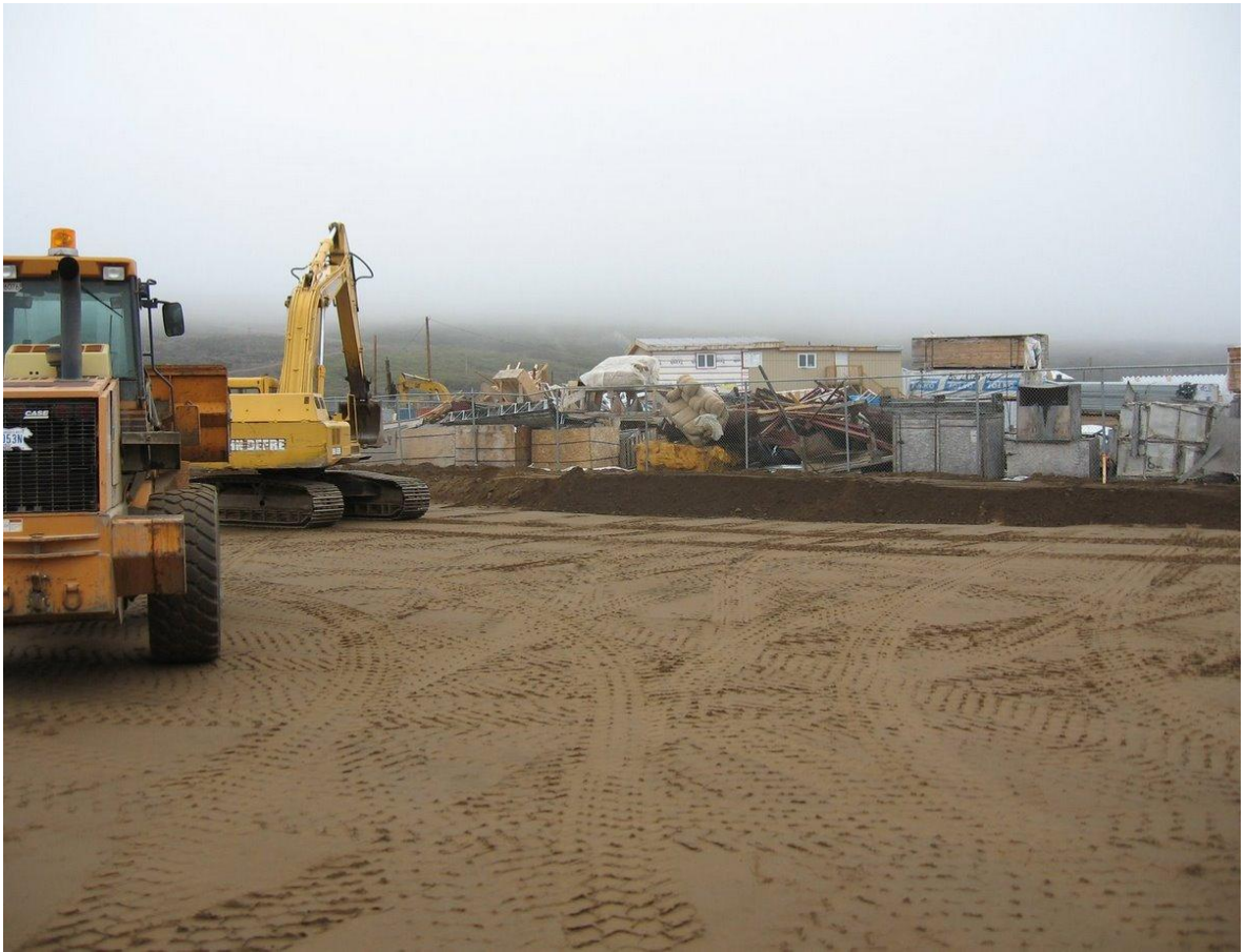
Excavator and loader used to carry materials and to pack walls tight
