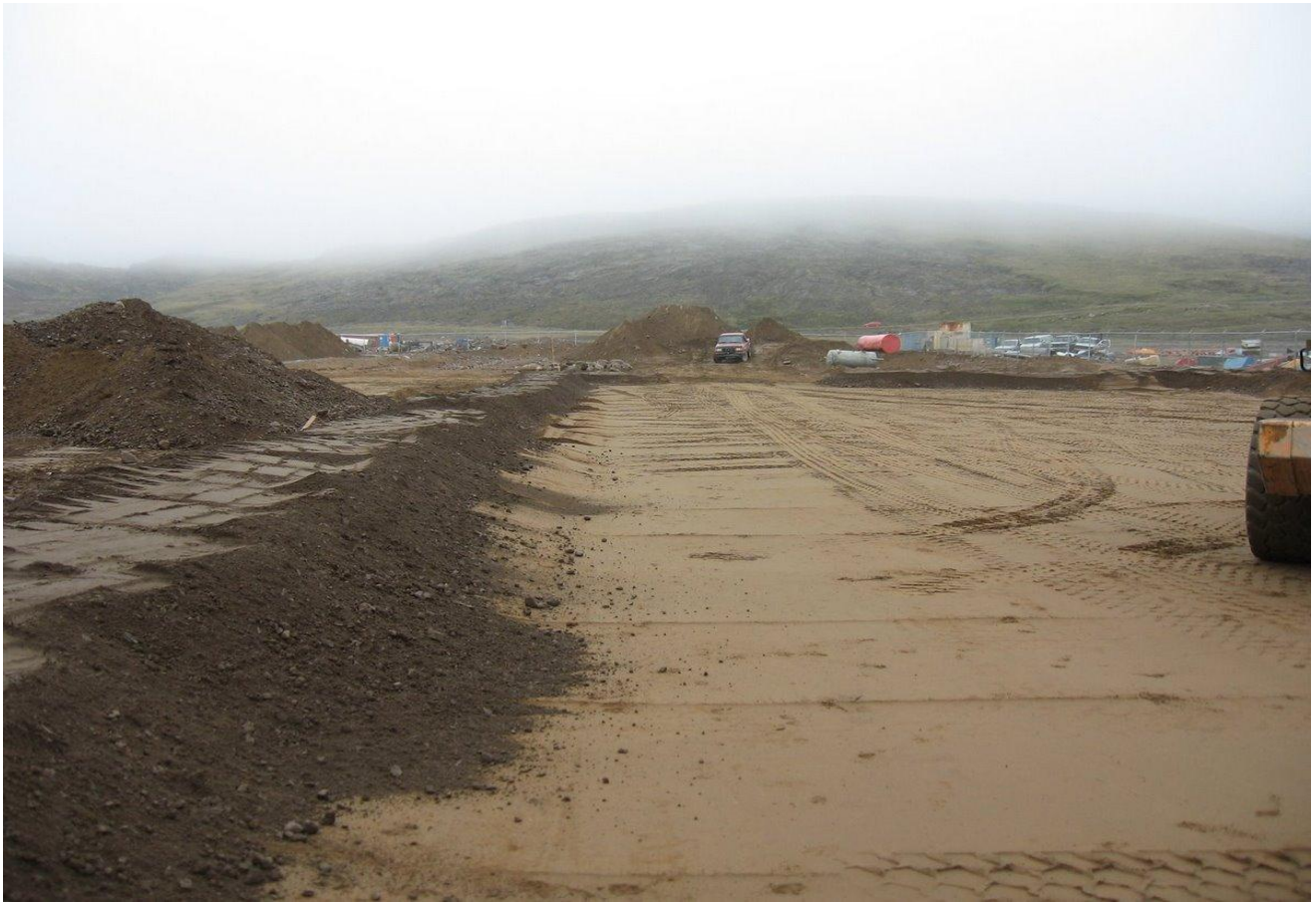
Small stones were raked out of inside cells and walls were covered with screened sand. To complete the formation of cell containment area.
