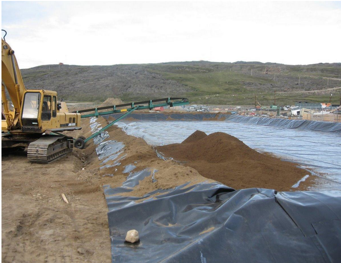
Screening plant and stacker used to get sand into new cell without damaging the liner. Sand was shoveled out until no more sand was available. Completion of cell will continue Summer of 2010 when city will allow removal of more sand from pit.
