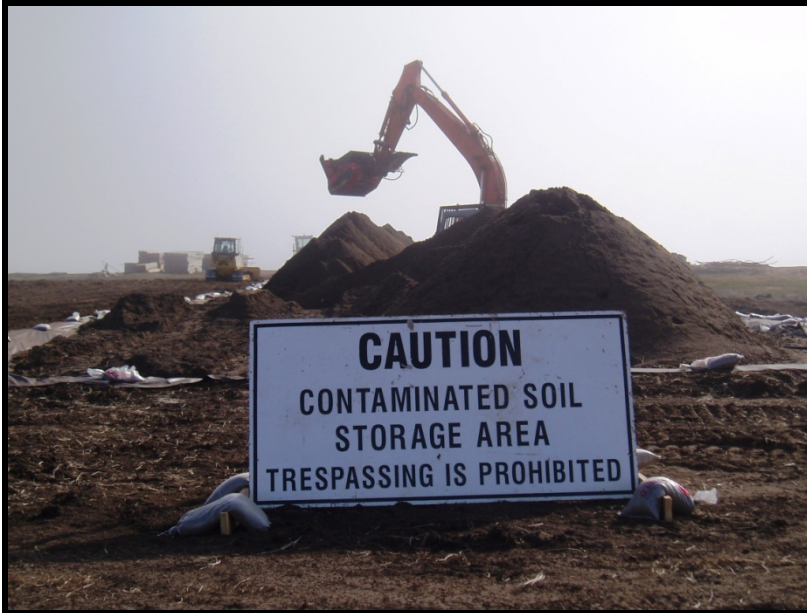
Figure 1 Allu Bucket Attached to Excavator
