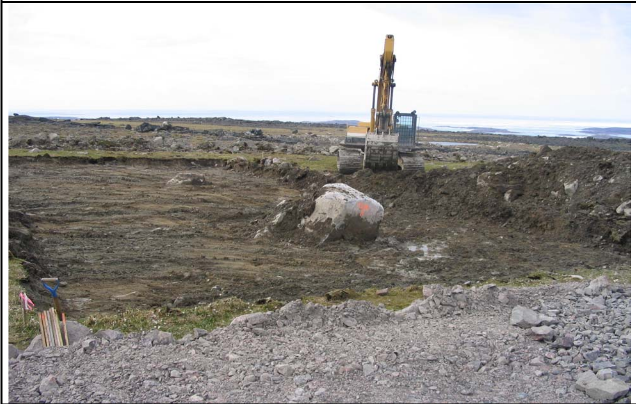
Photo 4: Contaminated soil excavation.
