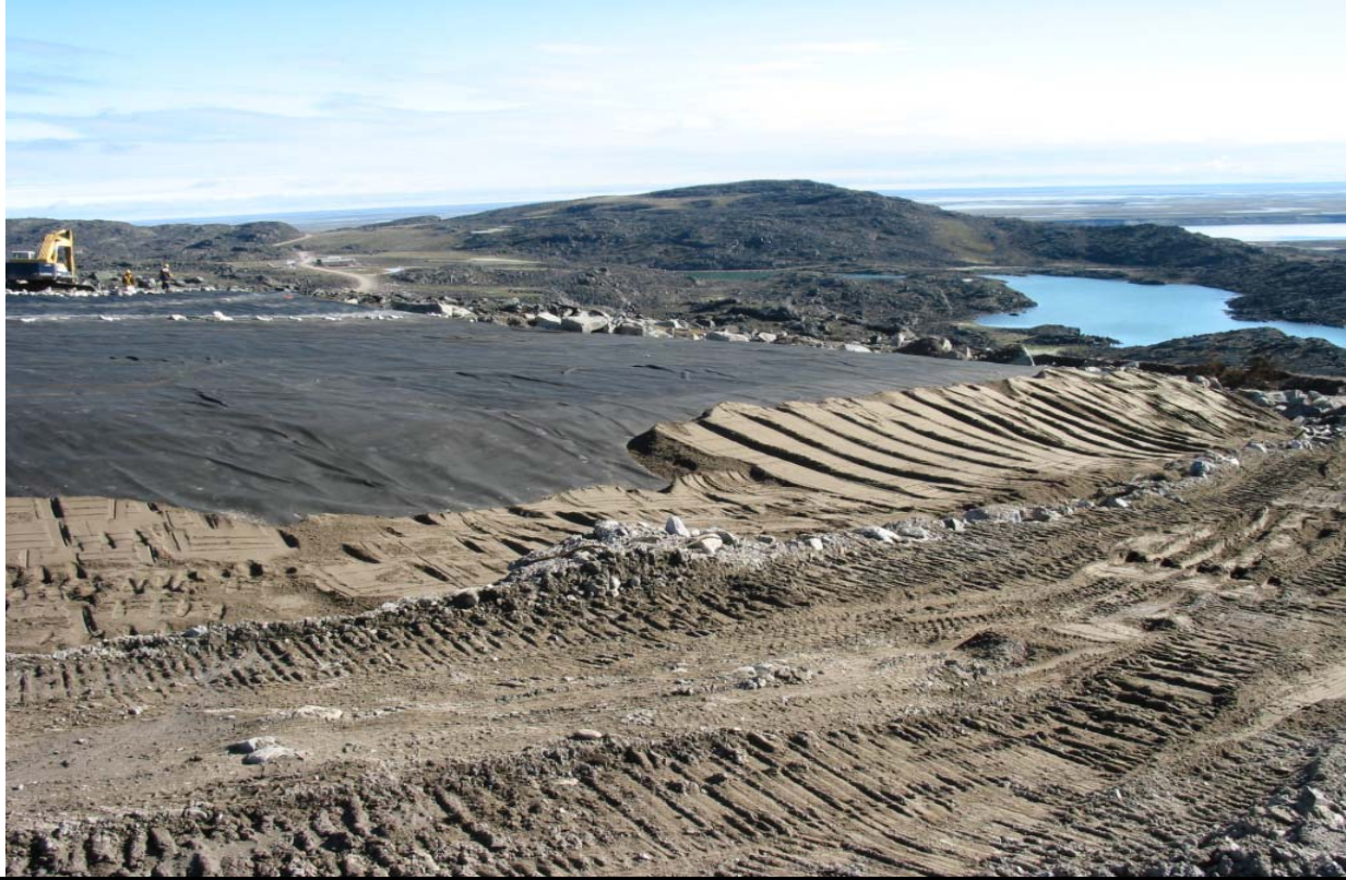
Photo 6: Liner and cover at the Upper Site Landfill.
