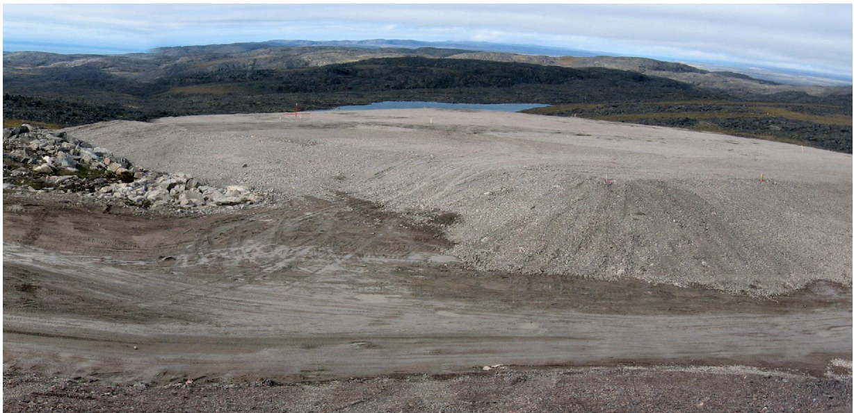
Photo 6: Station Non-Hazardous Waste Landfill
