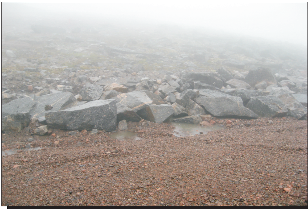
Photo 9 (Image 16) Upper Site Non-Hazardous Waste Landfill Ponded water along southwest facing toe of landfill.
