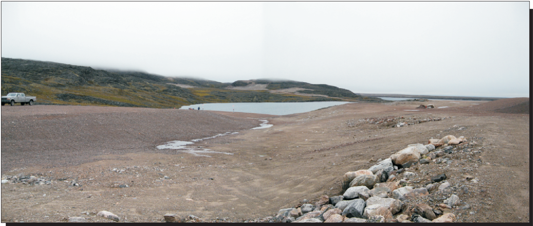
Photo 23 (Image 78) Lower Site Landfill Ponding along southeast side of landfill looking towards VT-11 and VT-12.
