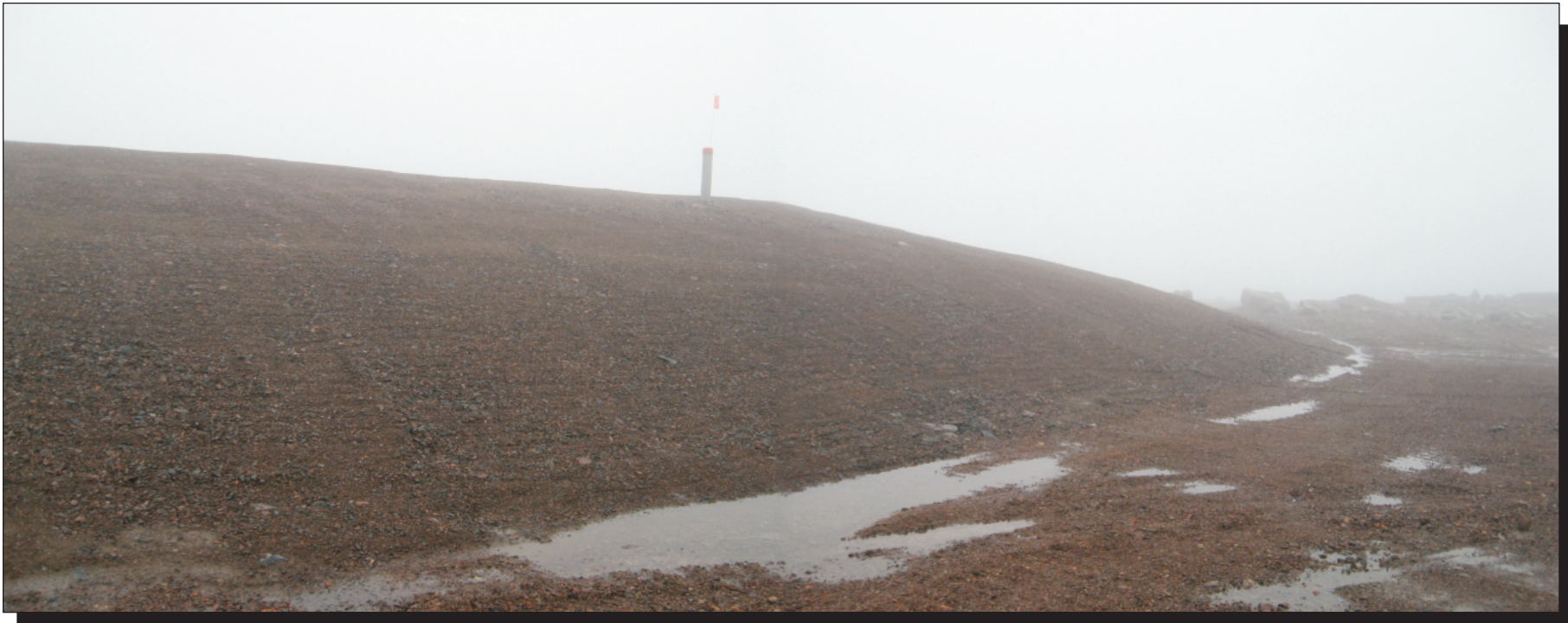
Photo 2 (Image 13) Upper Site Landfill Ponded water along toe of west facing slope looking south towards VT-4.
