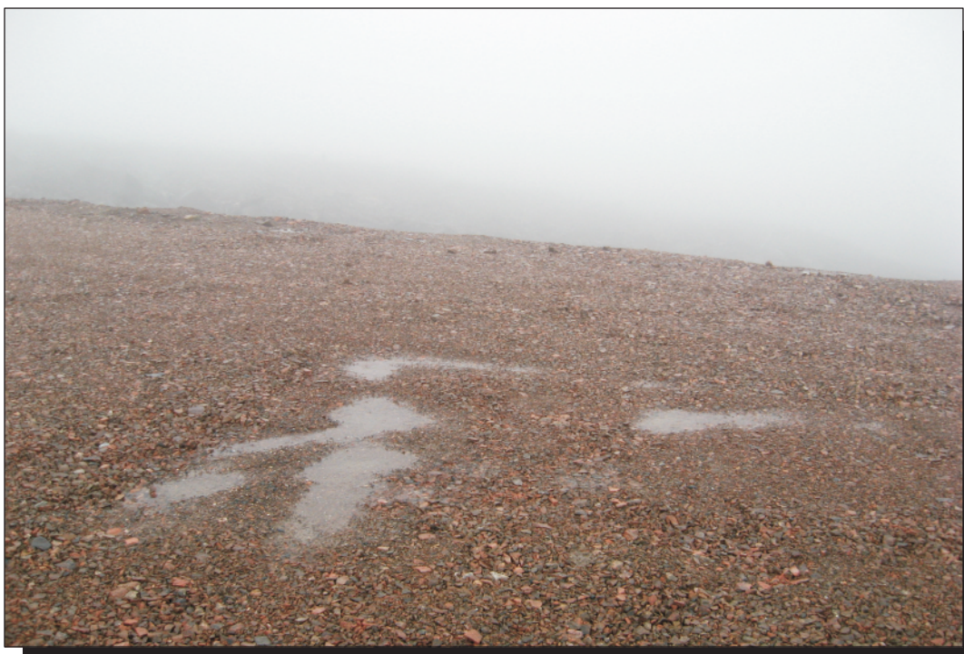
Photo 10 (Image 17) Upper Site Non-Hazardous Waste Landfill Ponded water on surface at northwest corner of landfill.
