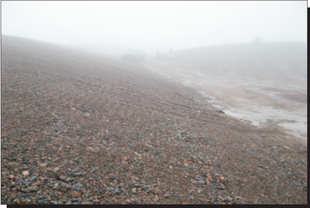
Photo 11 (Image 40) Tier II Soil Disposal Facility Ponded water along northeast facing slope looking northwest from east corner of landfill.
