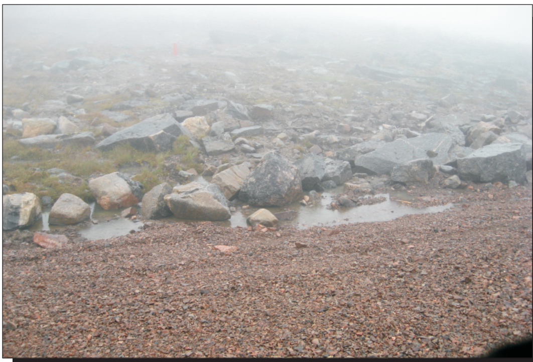
Photo 8 (Image 15) Upper Site Non-Hazardous Waste Landfill Ponded water along southwest facing toe of landfill.
