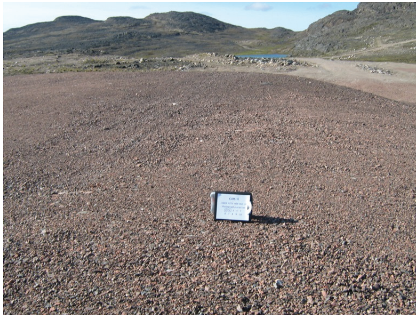
Photograph LNH-2B. Facing west along the crest from the centre of the north crest. Some tire tracks visible but no damage or rutting.____ ↑
