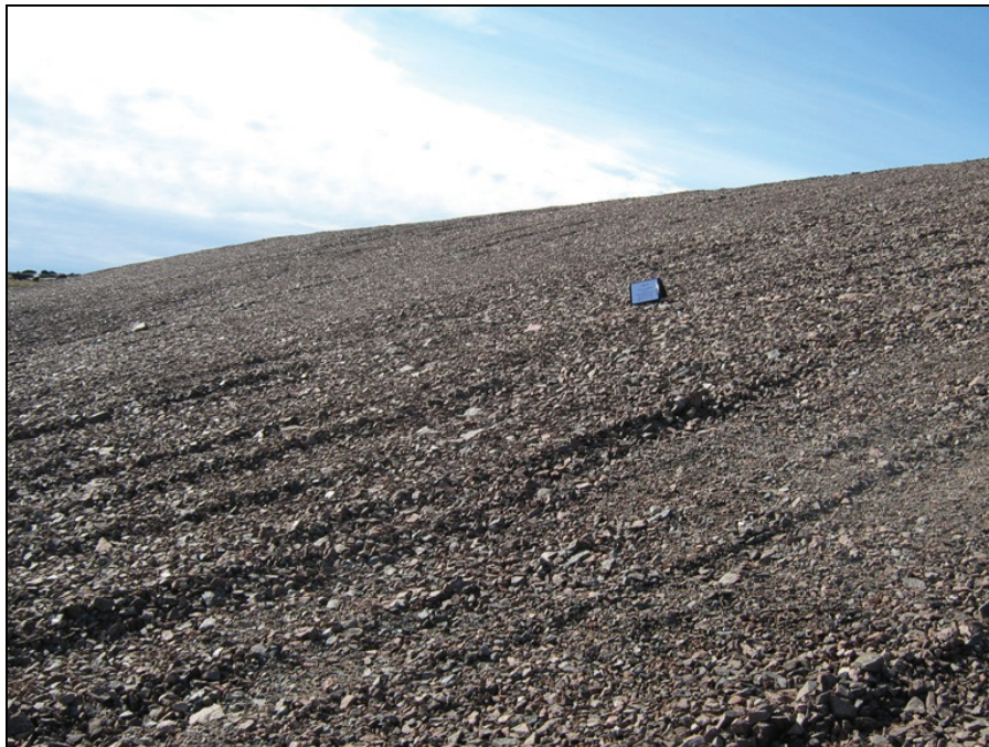
Photograph TII-7. South slope from southeast toe facing west. Some seepage from south slope and minor ponding at toe. No staining.____ ↑
