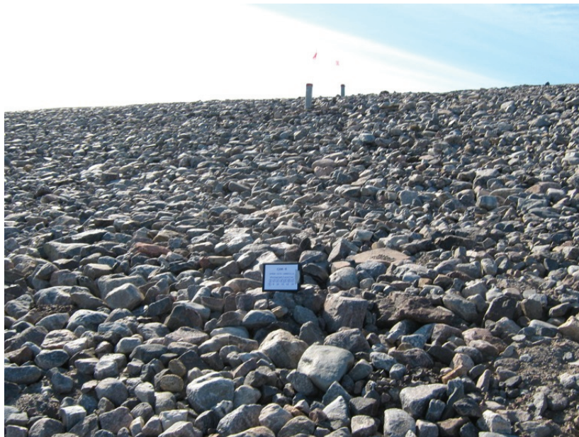
Photograph USL-8. Toe of rip-rap below thiermistors.____ ↑
