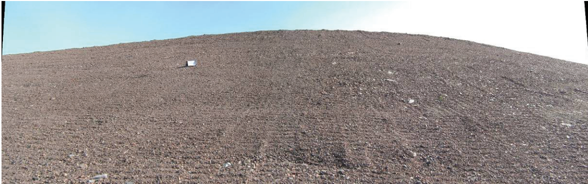
Photograph LSL-10. Panoramic photo facing southeast to the north slope at northwest end. Minor erosion of fines but self armouring. ↑
