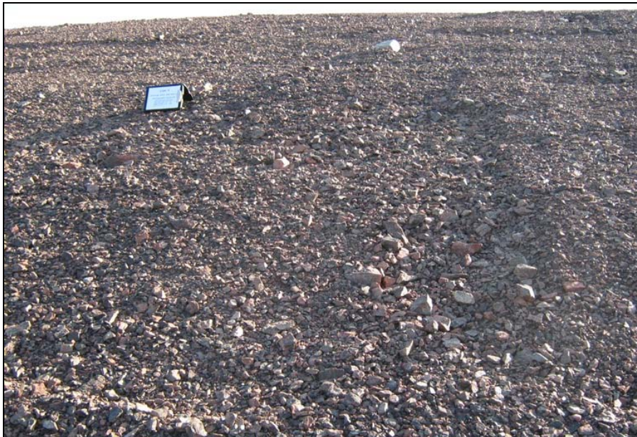
Photograph SNH-8. East slope. Area of possible minor erosion with gullies about 0.5m wide and less than 0.1m deep that appear to be self healing with larger rock in cover fill. ↑
