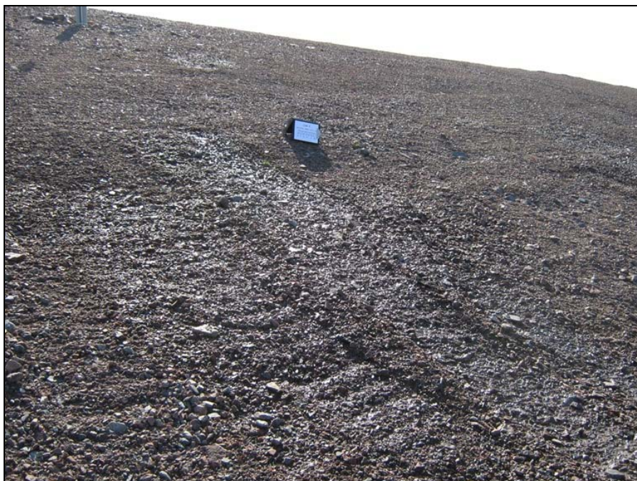
Photograph LSL-7. Facing southwest to the north slope near thermistors. Seepage from lower half of slope, with no staining observed. Very small tufts of grass/vegetation observed. ↑
