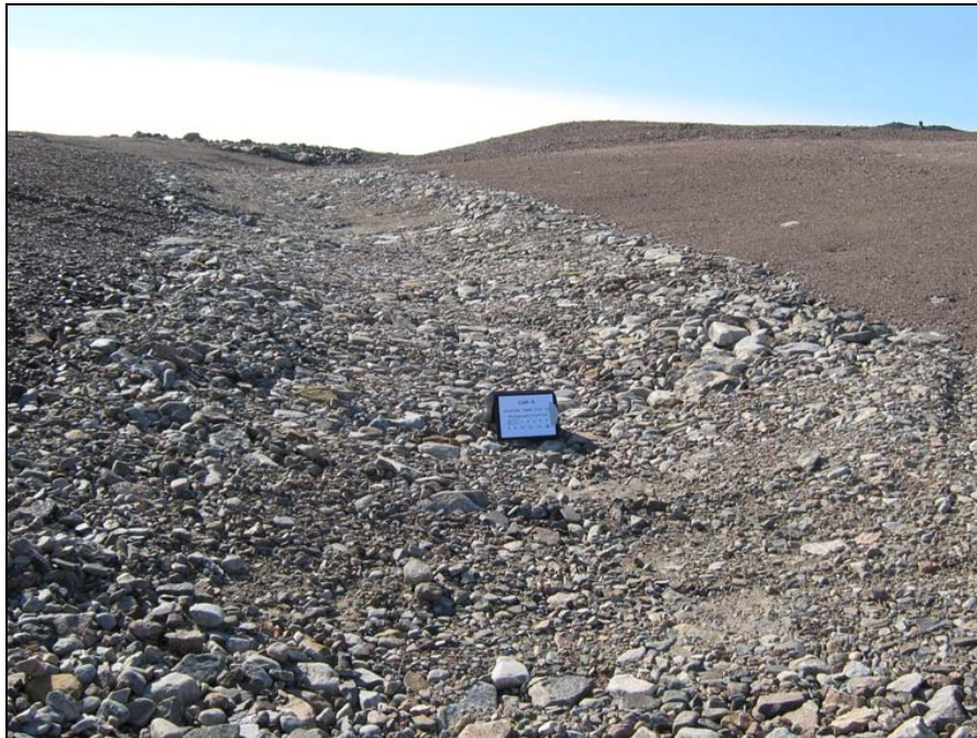
Photograph LSL-2A. Looking west, upstream, along the rip-rap lined drainage channel. ↑
