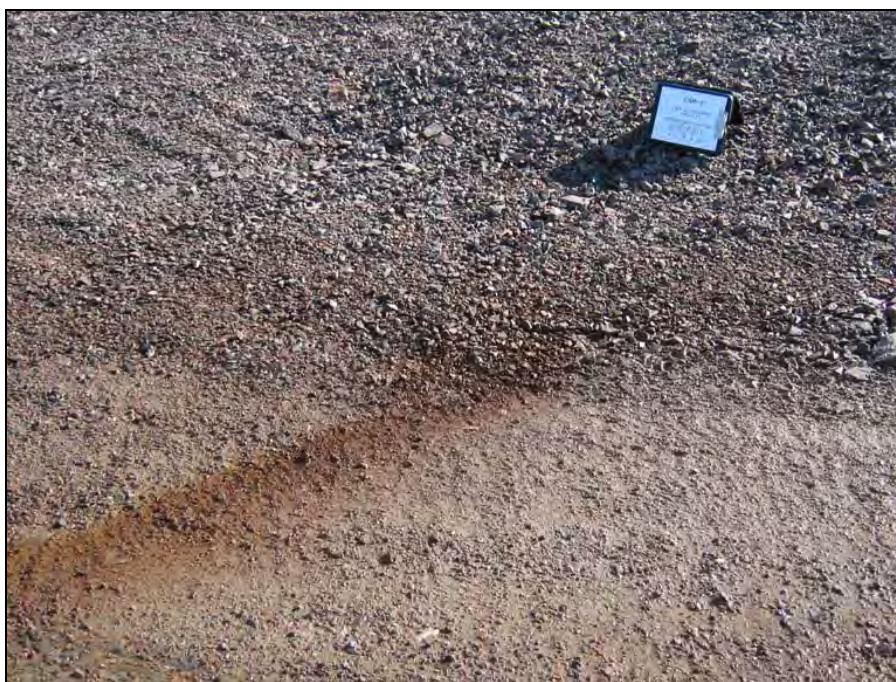
Photograph TII-4A. At the northeast toe. Some seepage with orange staining. Some water drainage along the road at the toe. ↑
