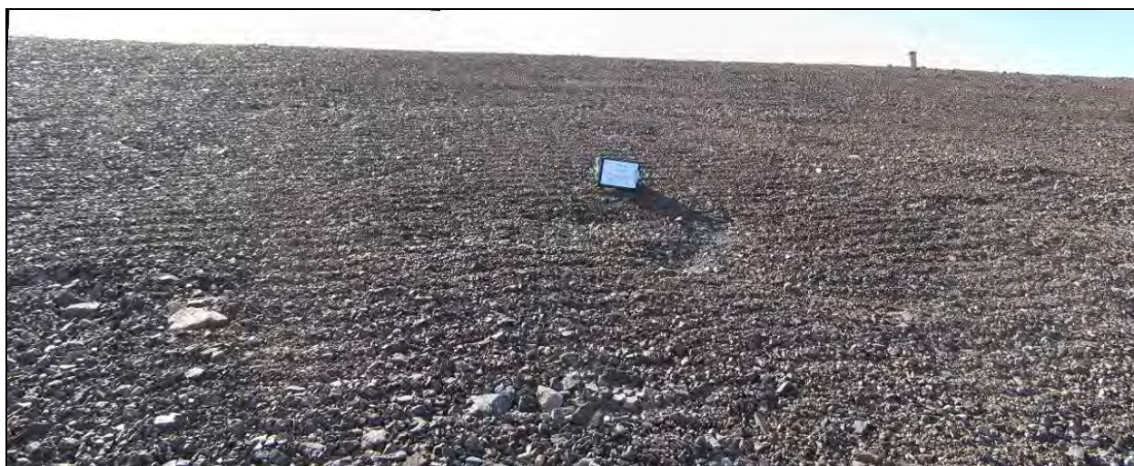
Photograph TII-6. Panoramic photo of the southeast slope. Some water seeping out of slope face. No staining. ↑
