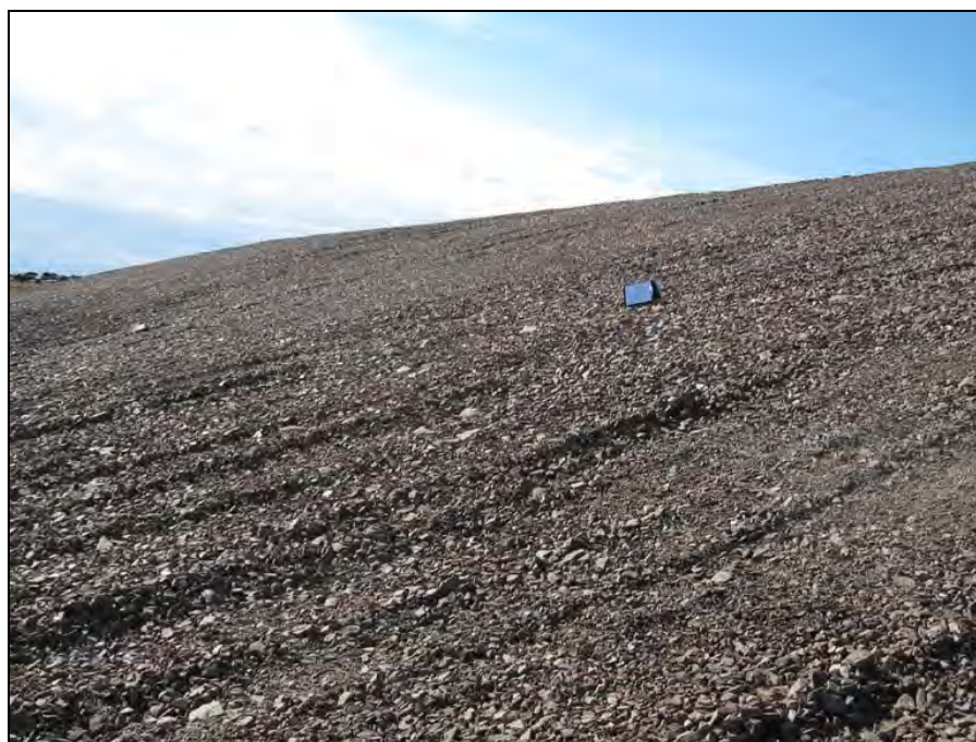
Photograph TII-7. South slope from southeast toe facing west. Some seepage from south slope and minor ponding at toe. No staining. ↑
