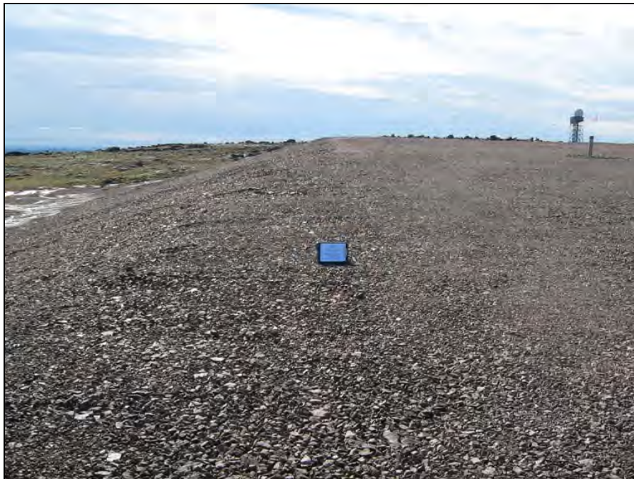
Photograph TII-5B. Southeast crest facing west. Some coarse rockfill along crest edge but there does not appear to be tension cracks. ↑
