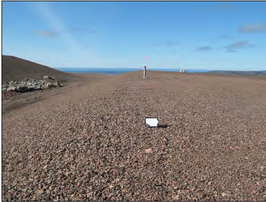
Photograph TII-9B. Facing north along crest from the southwest corner of the landfill. Some ponded water along toe. No staining. ↑
