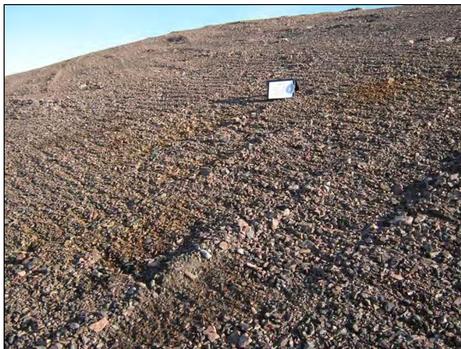
Photograph SNH-7A. Facing slope. Some seepage and orange staining over 10m x 10m area on lower half of east slope, towards the northeast corner toe. ↑
