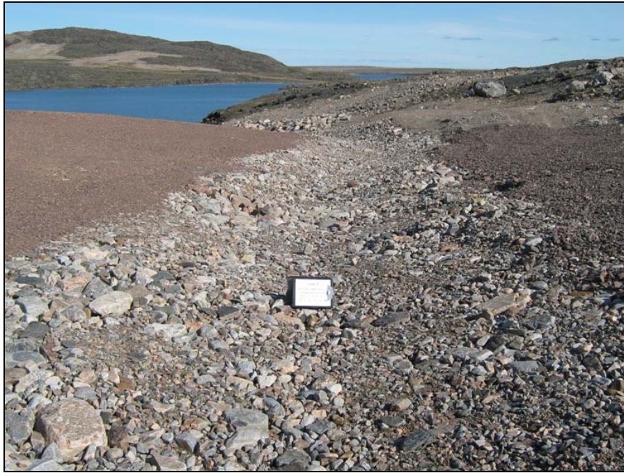
Photograph LSL-2B. Facing east, downstream, along the rip-rap lined drainage channel. ↑
