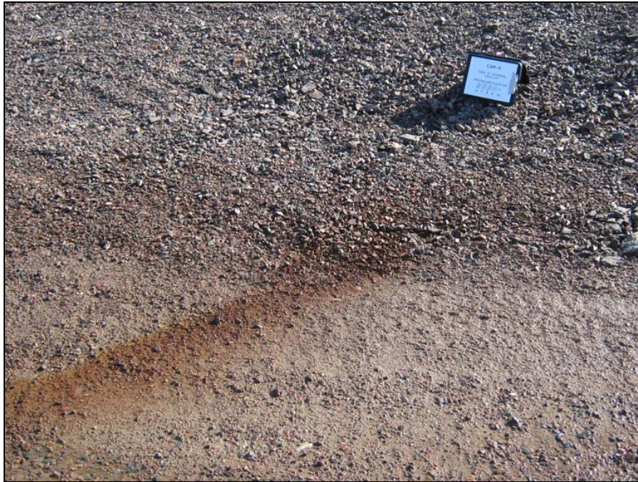
Photograph TII-4A. At the northeast toe. Some seepage with orange staining. Some water drainage along the road at the toe. ↑
