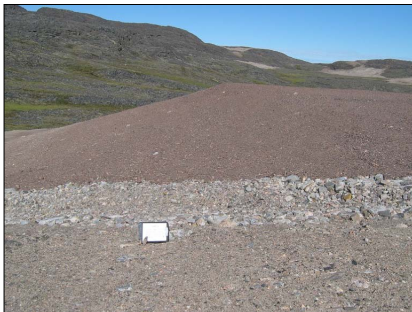
Photograph LSL-13. Facing northeast to the west slope and rip-rap lined drainage ditch at the toe of the landfill. ↑
