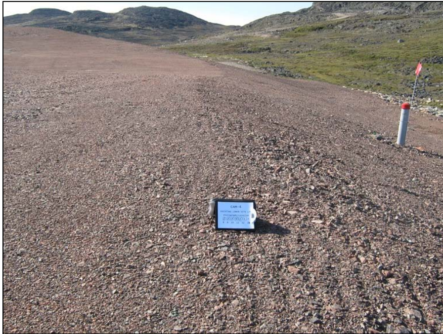
Photograph LSL-6. Facing west long the north crest. Some seepage from lower half of north face. No staining observed. ↑
