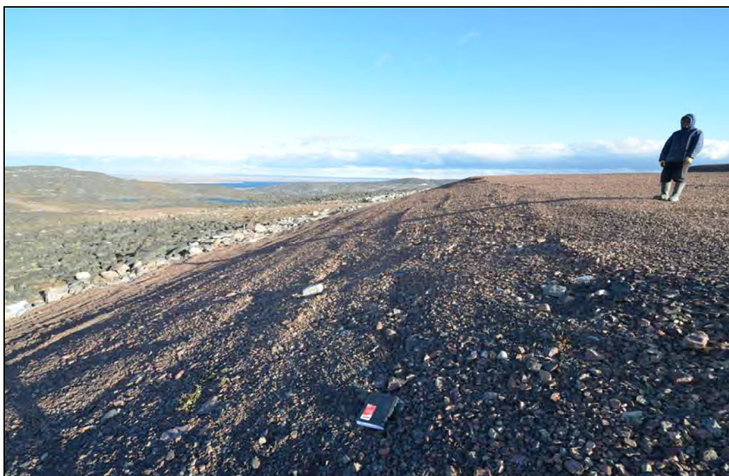
Photo 2: 2013-C4-LS-67 – Feature H – View E of an area of settlement on the northeast side slope. New observation.
