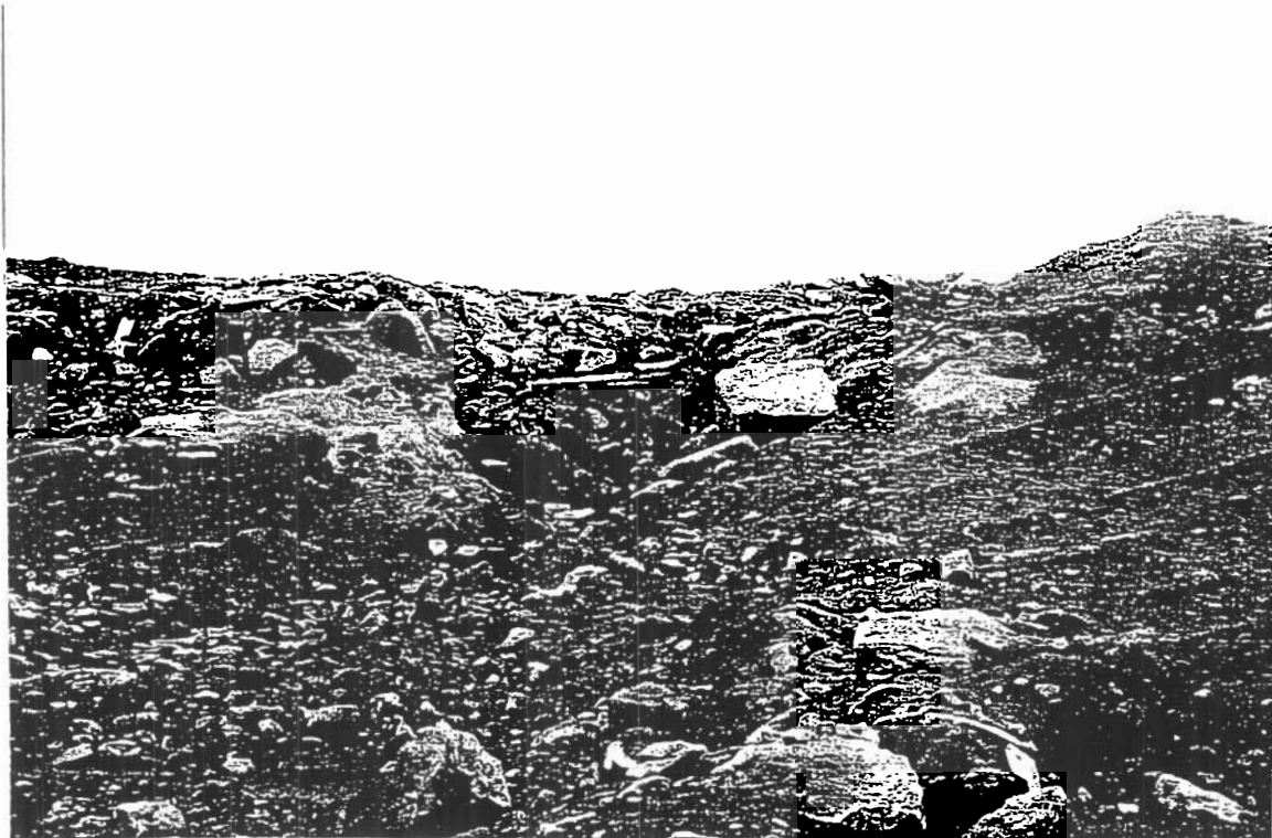
8. View of main landfill showing flowing erosion channel and exposed debris.
