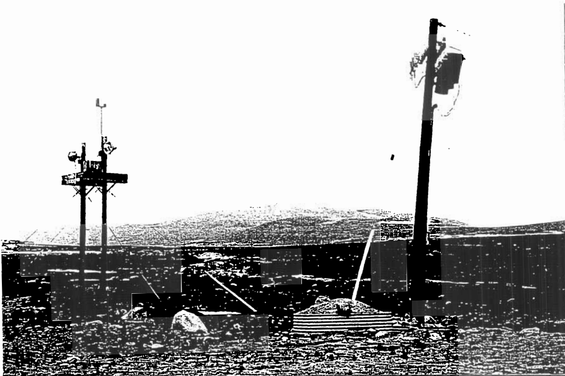
10. Pole-mount transformer and deacon tower located on airstrip apron.
