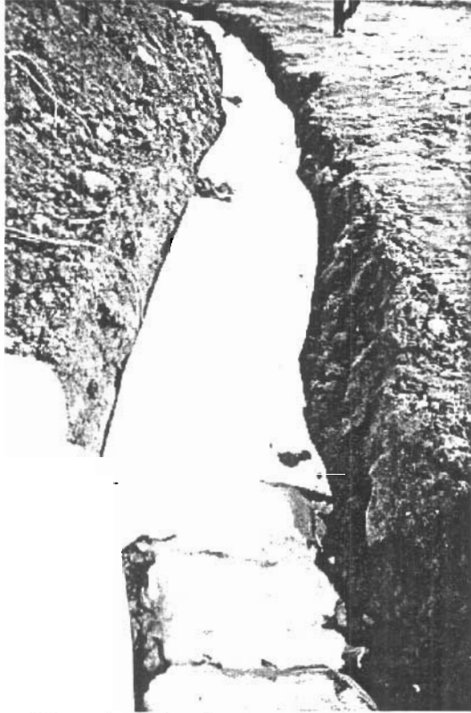
Photo 1 – Two layers of sorbant sweeps placed on bottom instead of pillows.
