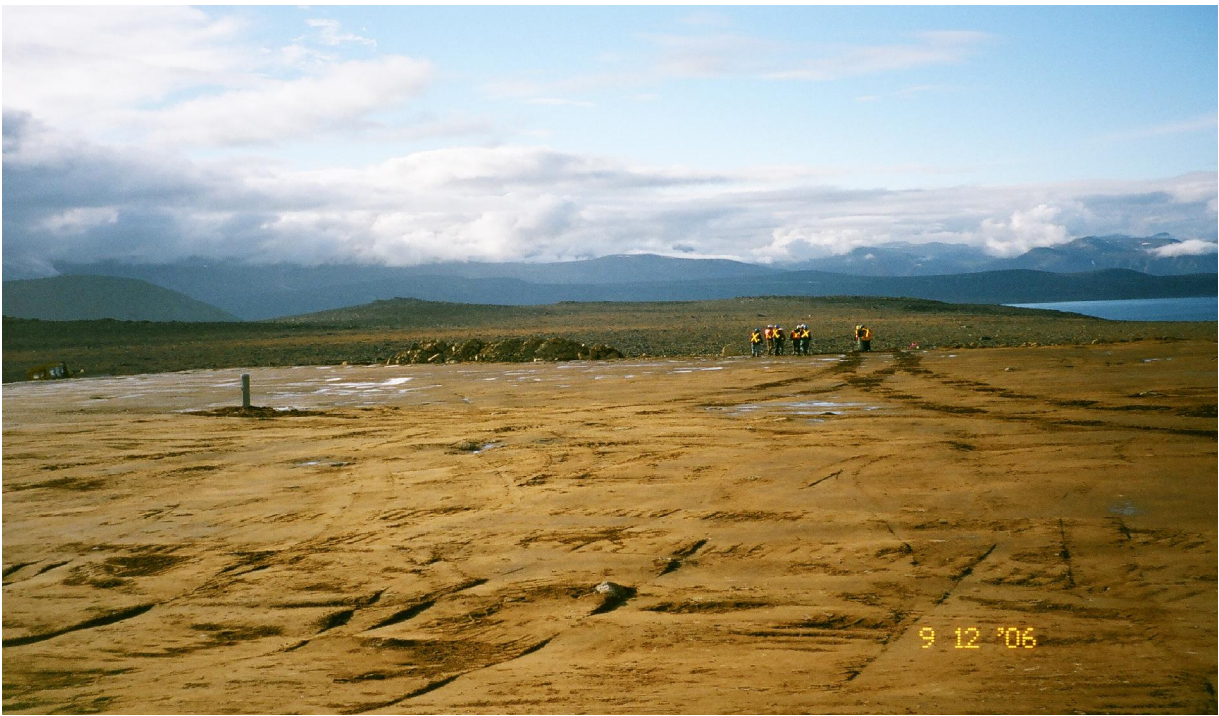
Photo 5: Middle Site Landfill – Tier II Soil Disposal Facility Cell
