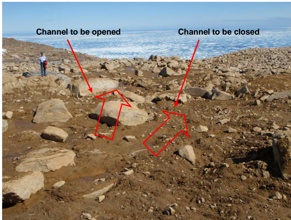
Photograph 11. Water diversion work, north side - Main Landfill ↑
