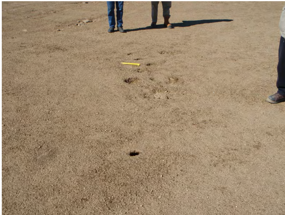
Photograph 12. Settlement pockets - Station Area Non-Hazardous Landfill ↑
