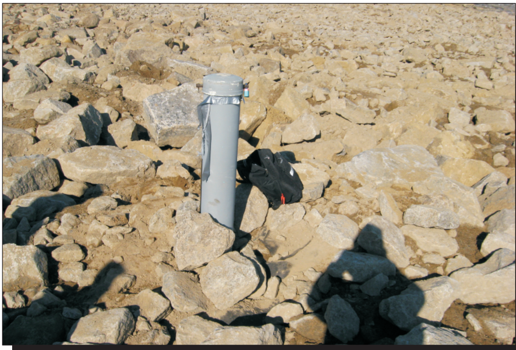
Photo 17 (Image 24 USMLF) Main Landfill - Non-woven geotextile exposed next to VT-5.
