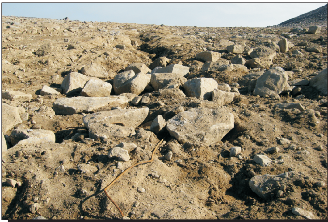
Photo 8 (Image 29 USMLF) Main Landfill - Partially exposed metal cable and erosional feature downslope of landfill.
