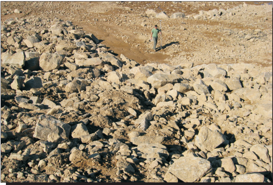
Photo 25 (Image 72 MSNHWLF) Middle Site Non-hazardous Waste Landfill - Minor erosion and migration of fine-grained sediment on northwest facing slope.
