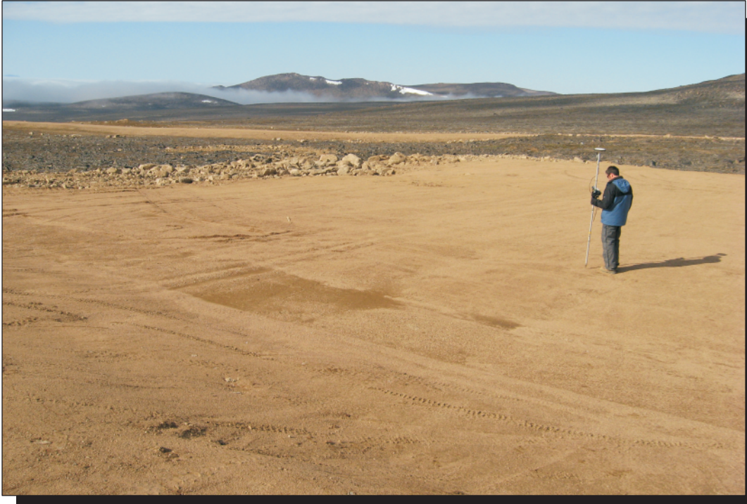
Photo 24 (Image 58 MSTII) Middle Site Non-hazardous Waste Landfill - Subtle depression and wet area on surface of landfill.
