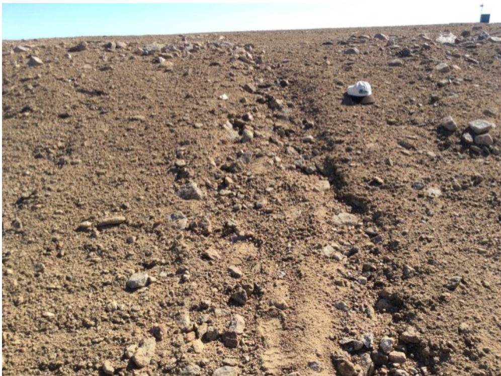
Photo 138: FOX-5 – Station Area NHWL – Northwest slope facing southeast – Feature S – self-armouring erosion channels (Acceptable) (ATT87_Photo87.jpg)
