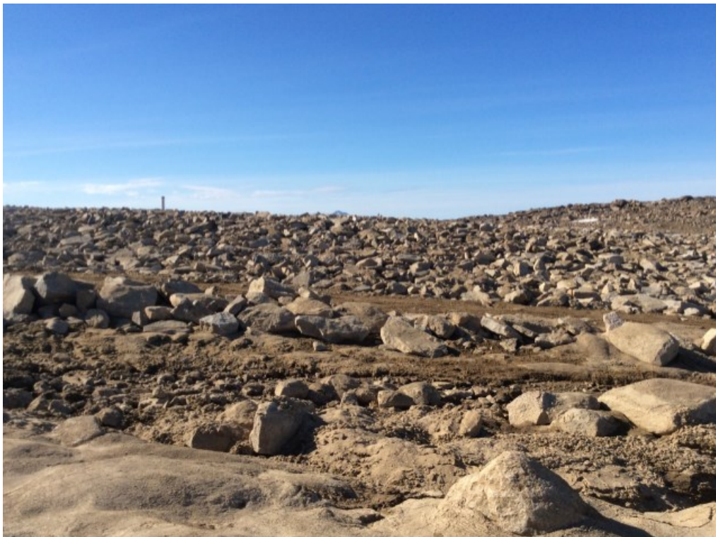
Photo 69: FOX-5 – Main Landfill – Southeast toe facing northwest with boulder rip rap slope in background – Feature F erosion channel along toe in foreground (Acceptable) (ATT39_Photo39.jpg)
