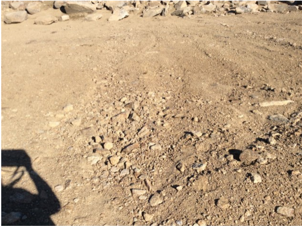
Photo 123: FOX-5 – Station Area NHWL – Northeast slope facing northeast – Feature E – self-armouring erosion (Acceptable) (ATT88_Photo88.jpg)
