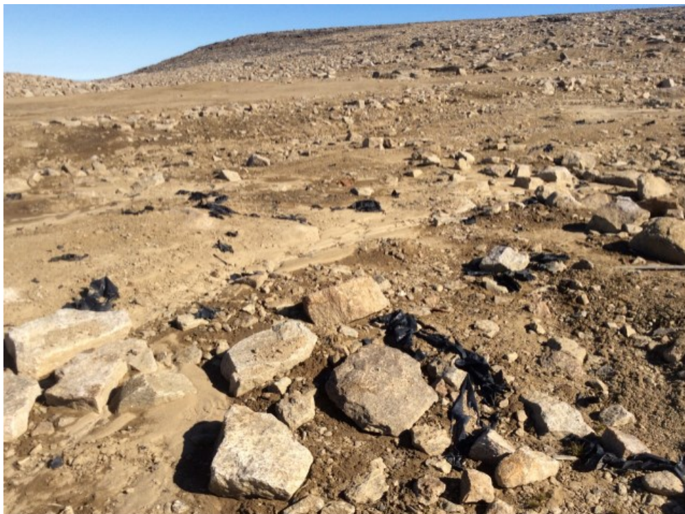
Photo 81: FOX-5 – Main Landfill – South toe facing southeast – Feature K – exposed shredded plastic debris around MW-10 (Acceptable) (ATT103_Photo103.jpg)
