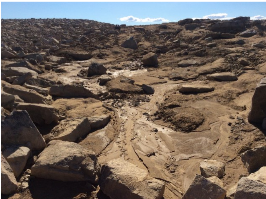
Photo 66: FOX-5 – Main Landfill – North toe facing southwest – Figure H – erosion channel along toe (Acceptable) (ATT36_Photo36.jpg)
