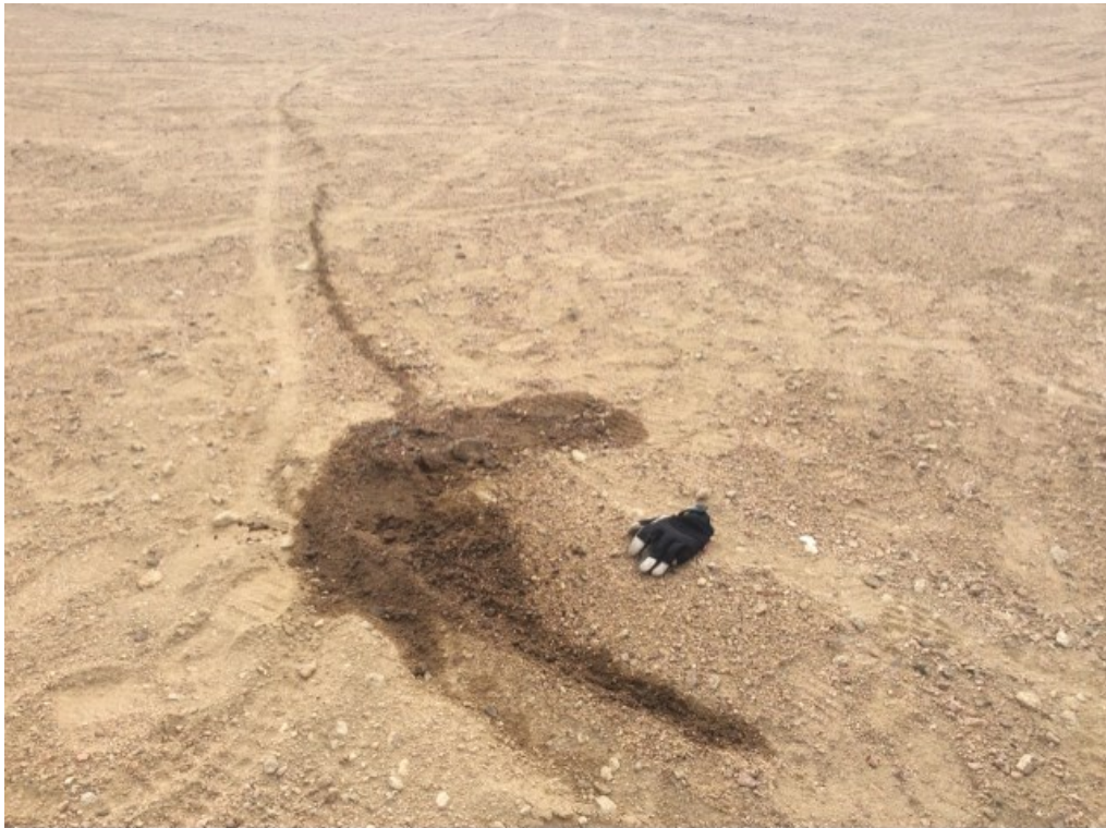
Photo 39: FOX-5 – Middle Site NHWL / Tier II DF – Northwest crest surface facing southeast – Feature Q – hydrocarbon staining not related to landfill performance (Acceptable) (ATT58_Photo58.jpg)
