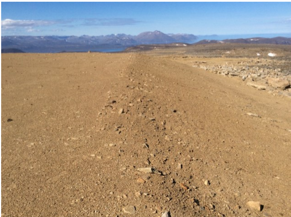
Photo 112: FOX-5 – Station Area NHWL – Crest edge, east corner, facing northwest – previously observed settlement (Feature F) considered rough grading (Acceptable) (ATT26_Photo26.jpg)
