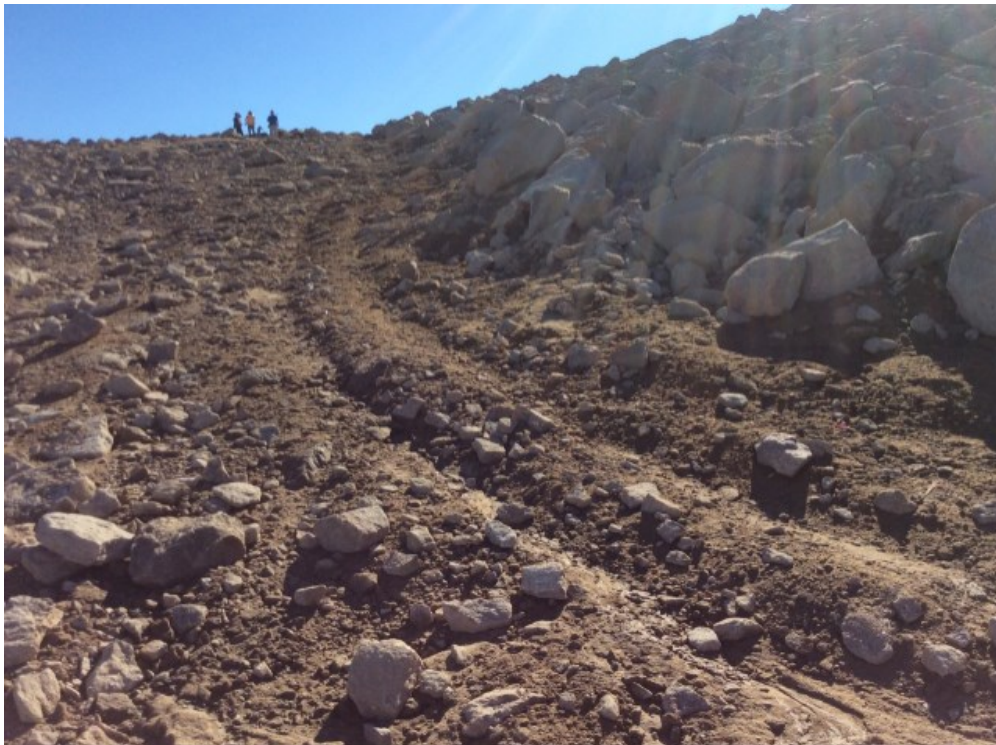
Photo 80: FOX-5 – Main Landfill – Northeast toe facing south – Feature D – north end of erosion channel along toe (Acceptable) (ATT108_Photo108.jpg)
