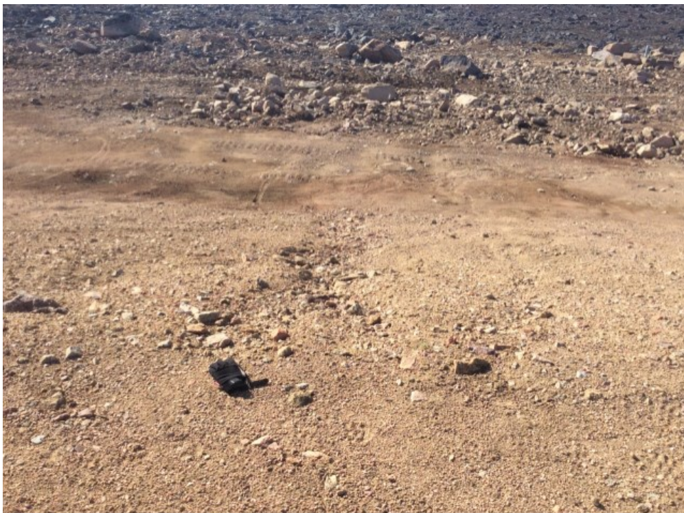
Photo 36: FOX-5 – Middle Site NHWL / Tier II DF – South slope facing southwest – Feature C – self-armouring erosion channels (Acceptable) (ATT46_Photo46.jpg)
