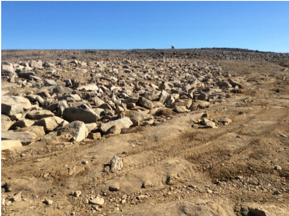
Photo 65: FOX-5 – Main Landfill – Boulder rip rap on west slope facing southeast (ATT35_Photo35.jpg)
