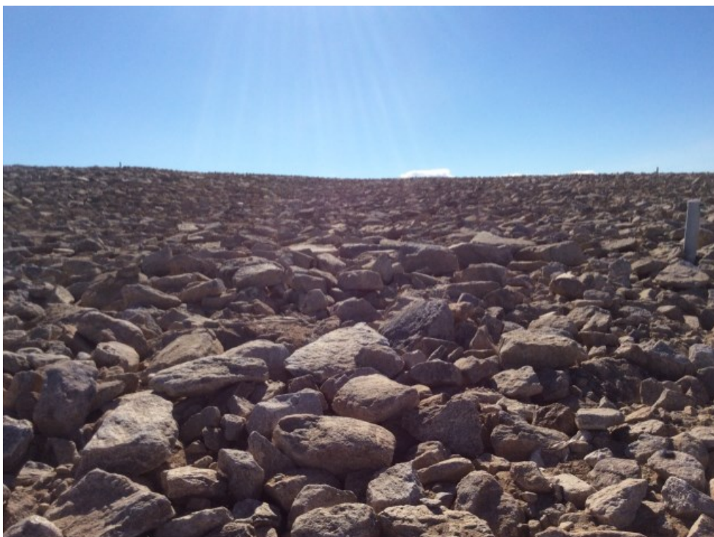
Photo 68: FOX-5 – Main Landfill – East crest surface facing southwest with boulder rip rap (ATT38_Photo38.jpg)
