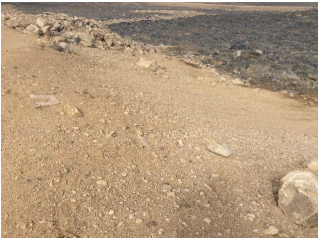
Photo 32: FOX-5 – Middle Site NHWL / Tier II DF – North slope facing northwest – Previously observed Feature M erosion channels have self-armoured (Acceptable) (ATT56_Photo56.jpg)
