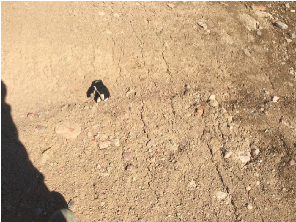
Photo 30: FOX-5 – Middle Site NHWL / Tier II DF – Northeast slope facing north – Feature H – Parallel cracking on slope (Acceptable) (ATT52_Photo52.jpg)
