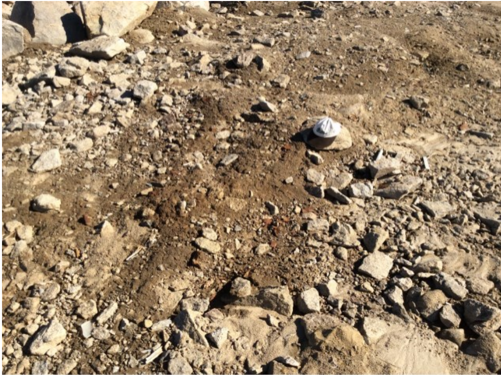
Photo 79: FOX-5 – Main Landfill – West toe facing northwest – Feature I – metal debris exposed by erosion around toe of landfill (Acceptable) (ATT105_Photo105.jpg)
