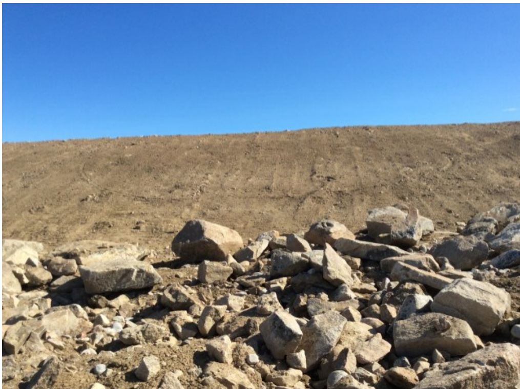
Photo 118: FOX-5 – Station Area NHWL – Northwest slope facing southeast - Motorbike tracks on slope – Previously observed settlement (Feature Q) is likely rough grading and not significant (ATT32_Photo32.jpg)
