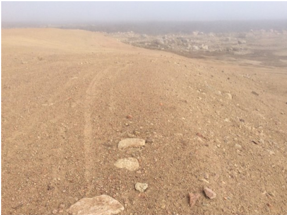
Photo 12: FOX-5 – Middle Site NHWL / Tier II DF - Crest facing northeast – Previously observed erosion channels (Feature F) were not observed in 2016 and could have been early self-armouring, north end of thin minor crack along crest edge (Feature O – not visible in photo) (ATT14_Photo14.jpg)
