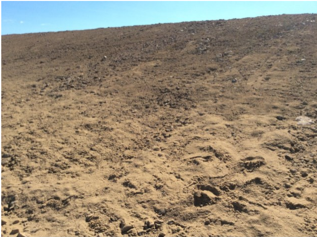
Photo 139: FOX-5 – Station Area NHWL – Northeast slope facing southeast – Feature E – self-armouring erosion channels (Acceptable) (ATT97_Photo97.jpg)
