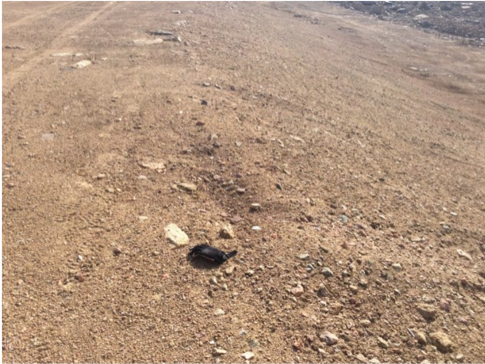
Photo 35: FOX-5 – Middle Site NHWL / Tier II DF – South crest edge facing southeast – Feature N – minor settlement at crest edge (Acceptable) (ATT44_Photo44.jpg)
