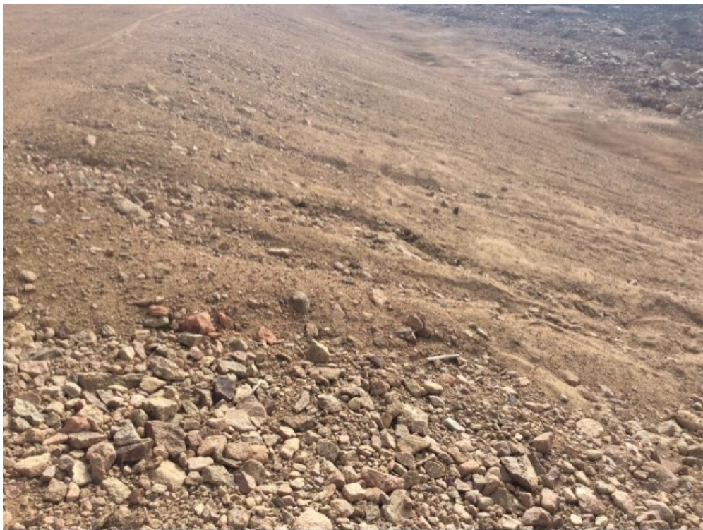
Photo 24: FOX-5 – Middle Site NHWL / Tier II DF – South slope facing southeast – Feature C – Self-armouring erosion (Acceptable) (ATT42_Photo42.jpg)
