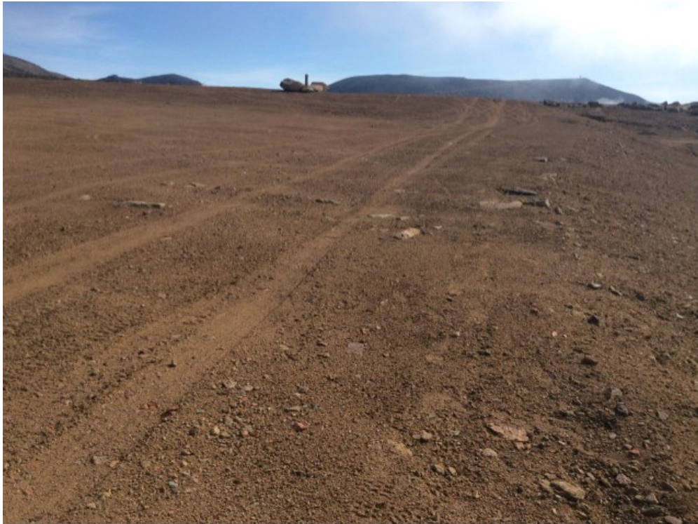
Photo 25: FOX-5 – Middle Site NHWL / Tier II DF – Southeast crest surface facing southeast – Feature D – Vehicle tracks from trucks, quads and dirt bikes are present over most of the landfill surfaces (Acceptable) (ATT45_Photo45.jpg)
