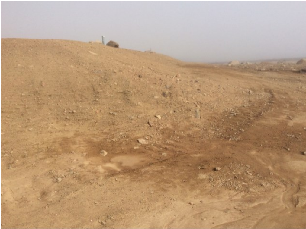
Photo 9: FOX-5 – Middle Site NHWL / Tier II DF - Southeast toe facing north – Previously observed settlement (Feature E) likely just rough grading (ATT11_Photo11.jpg)
