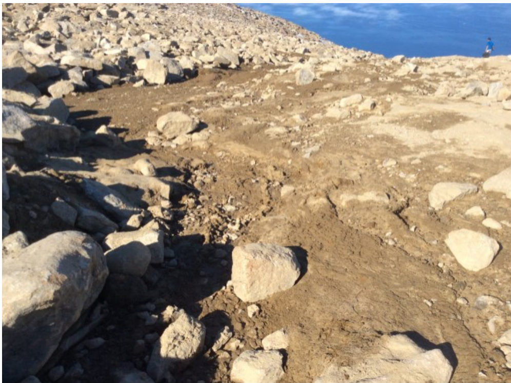
Photo 76: FOX-5 – Main Landfill – East toe facing northeast – Feature D – south end of erosion channel along north east toe (Acceptable) (ATT110_Photo110.jpg)
