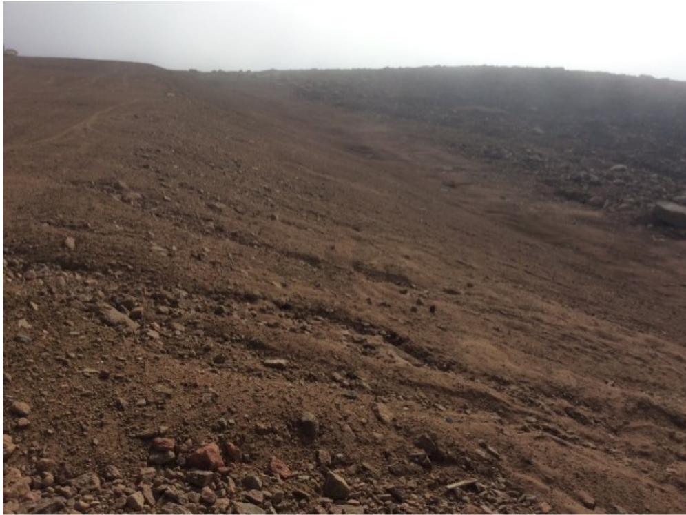
Photo 23: FOX-5 – Middle Site NHWL / Tier II DF – South slope facing southeast – Feature C – Self-armouring erosion, multiple channels (Acceptable) (ATT43_Photo43.jpg)
