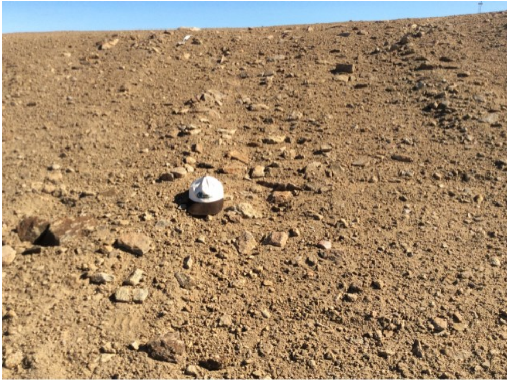
Photo 135: FOX-5 – Station Area NHWL – Northwest slope facing southeast – Feature P – minor self-armouring erosion (Acceptable) (ATT100_Photo100.jpg)
