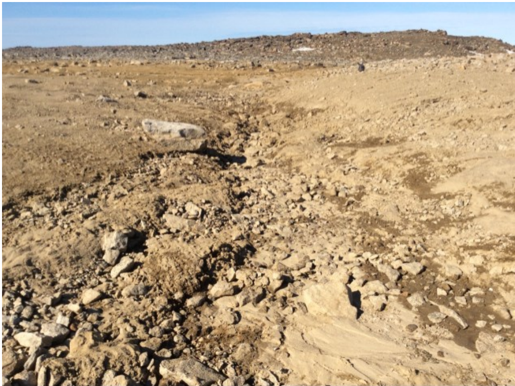
Photo 64: FOX-5 – Main Landfill – Drainage ditch, west of landfill, facing north – Feature H – erosion channel (Acceptable) (ATT34_Photo34.jpg)
