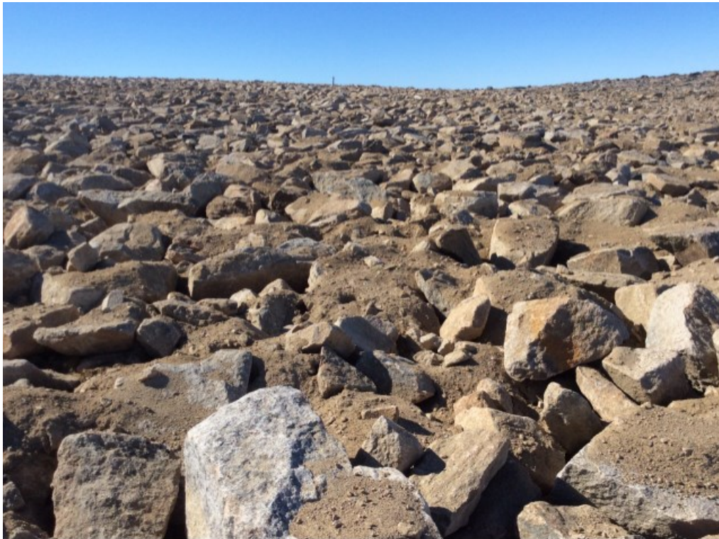
Photo 71: FOX-5 – Main Landfill – Crest surface facing west, boulder rip rap with sand and gravel on top (ATT41_Photo41.jpg)
