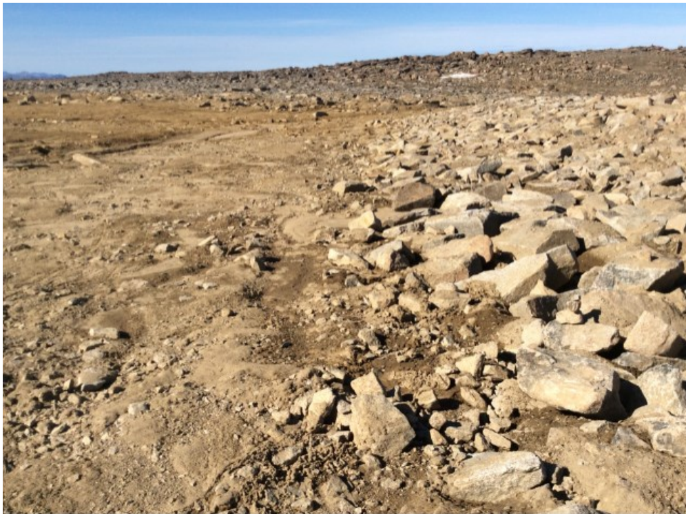
Photo 78: FOX-5 – Main Landfill – Southwest toe facing northwest – Previously observed erosion (Feature H) around toe of landfill (Acceptable) (ATT104_Photo104.jpg)
