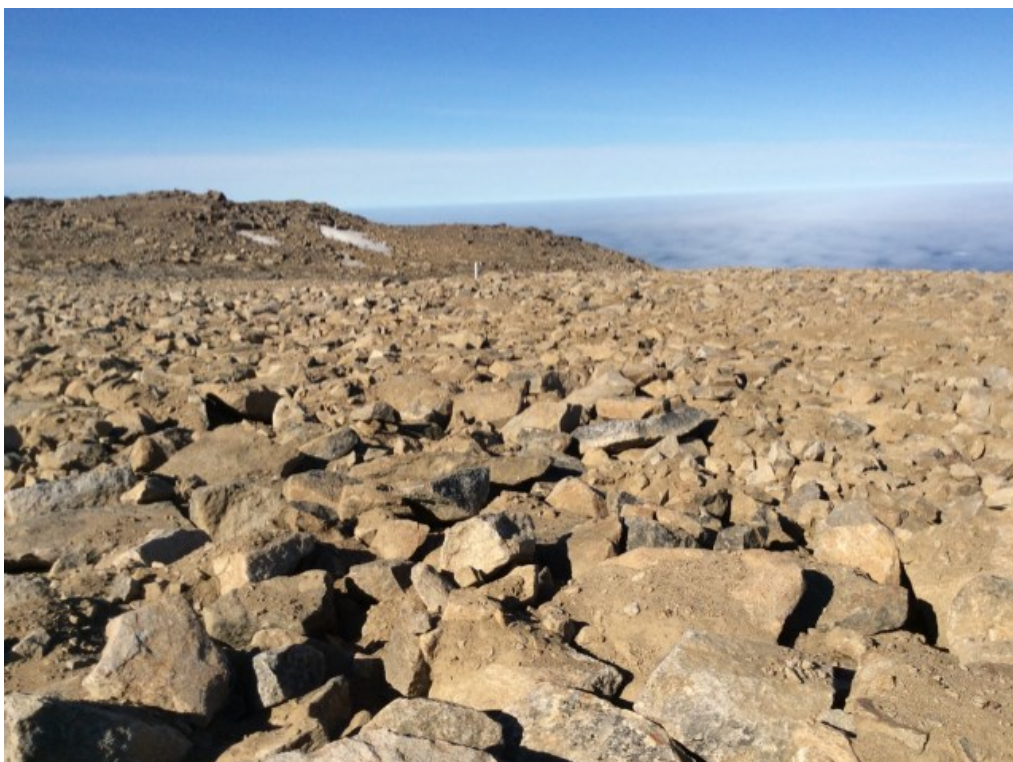
Photo 70: FOX-5 – Main Landfill – South crest surface facing north with boulder rip rap (ATT40_Photo40.jpg)
