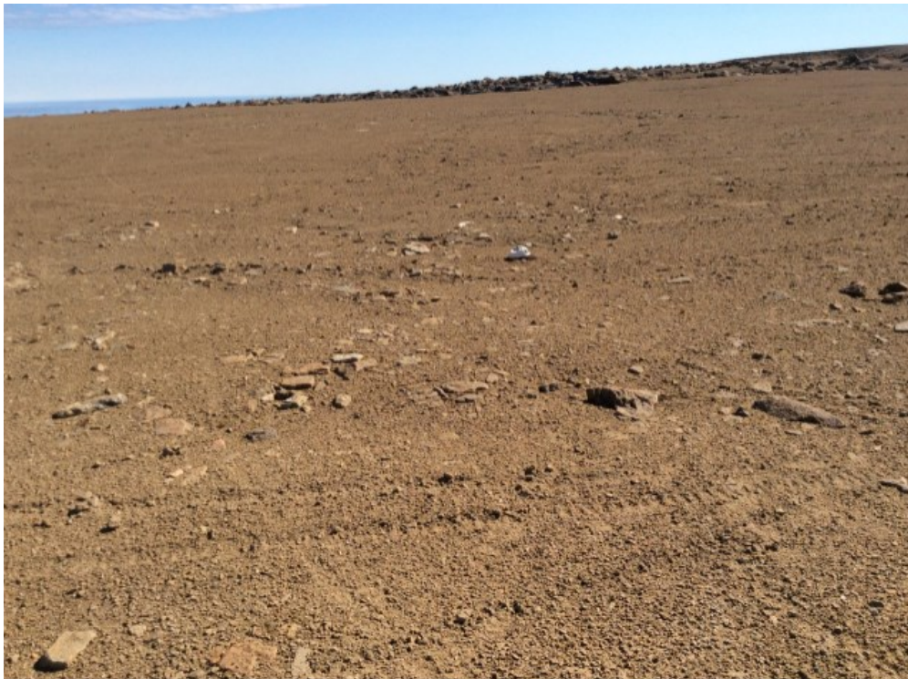
Photo 134: FOX-5 – Station Area NHWL – North crest surface facing northwest – Previously observed settlement (Feature O) on crest are very shallow depressions and not considered significant (ATT85_Photo85.jpg)
