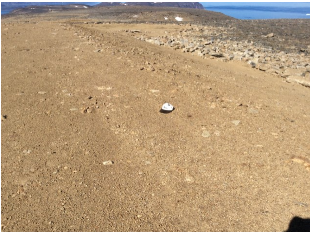
Photo 122: FOX-5 – Station Area NHWL – Northeast crest facing north – Previously observed settlement (Feature D) is very shallow and not considered significant (ATT89_Photo89.jpg)
