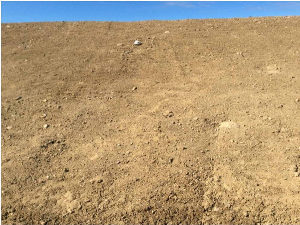
Photo 126: FOX-5 – Station Area NHWL – Southeast slope facing northwest – Feature H – minor self-armouring erosion (Acceptable) (ATT96_Photo96.jpg)
