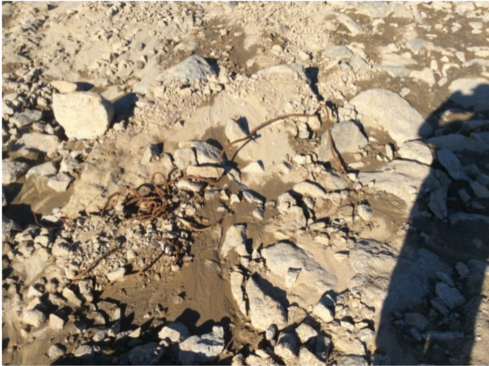
Photo 75: FOX-5 – Main Landfill – Steel cable at east toe - Example of previously observed Features B, C and E which are not exposed waste materials but construction debris/remnants (Acceptable) (ATT111_Photo111.jpg)
