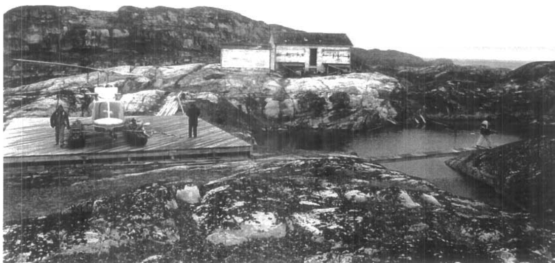
Photo 4.2 Facing southeast at freshwater pond/reservoir west of main house. Reservoir already has a substantial amount of debris in it
