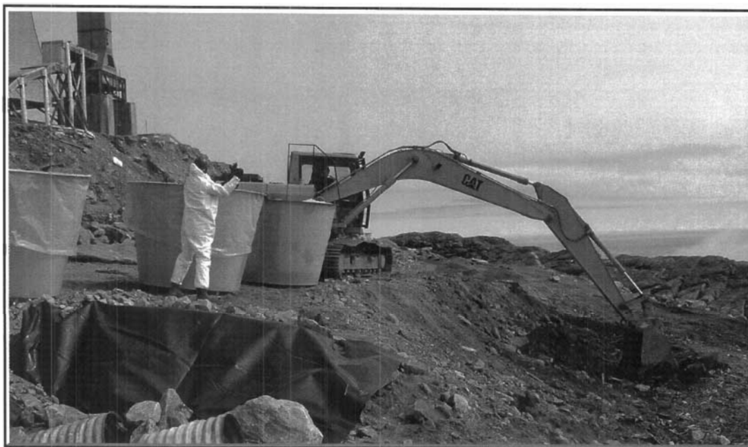
Photograph 3.2 Excavation of CEPA Soil (> 2000 ppm) in S1/S4 Valley
