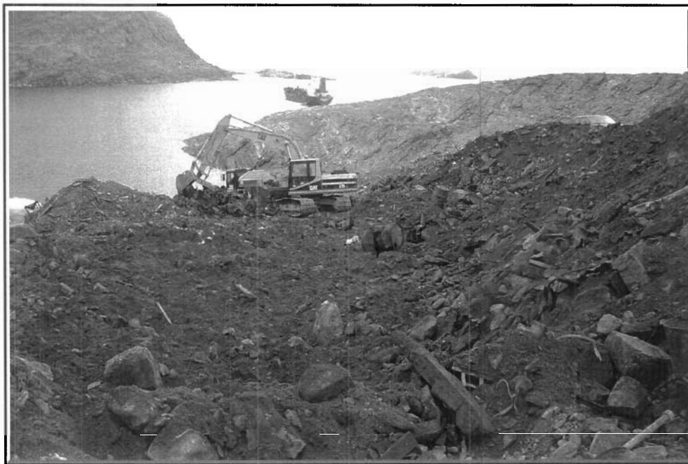
Photograph 5.1: Excavation of Waste Debris at the Lead Beach Dump
