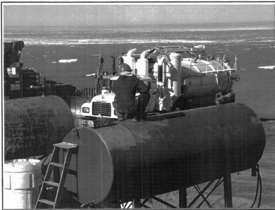
Photograph 7.2: Painting the Gasoline Tank Near the Core Camp
