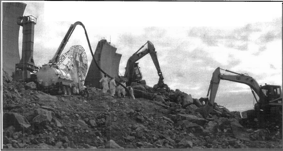
Photograph 3.1 Excavation and Vacuuming of CEPA Soil in S1/S4 Valley
