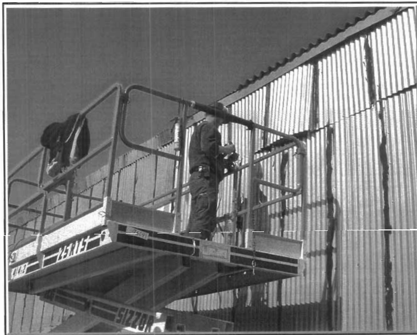
Photograph 9.1 Repairs to Main PCB Storage Building Cladding
