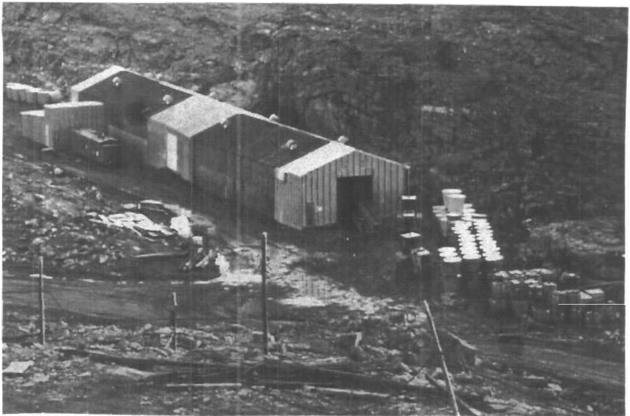
Photograph V-3: The Main PCB Storage Facility in Which Excavated CEPA Soil is Stored Awaiting Containerisation in Steel Conical Containers.
