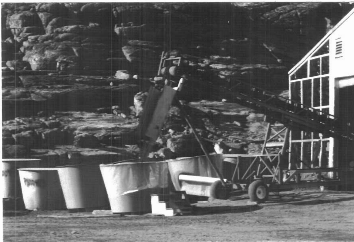
Photograph I-2: Filling the Conical Steel Containers with PCB Contaminated Soils from the Main PCB Storage Facility
