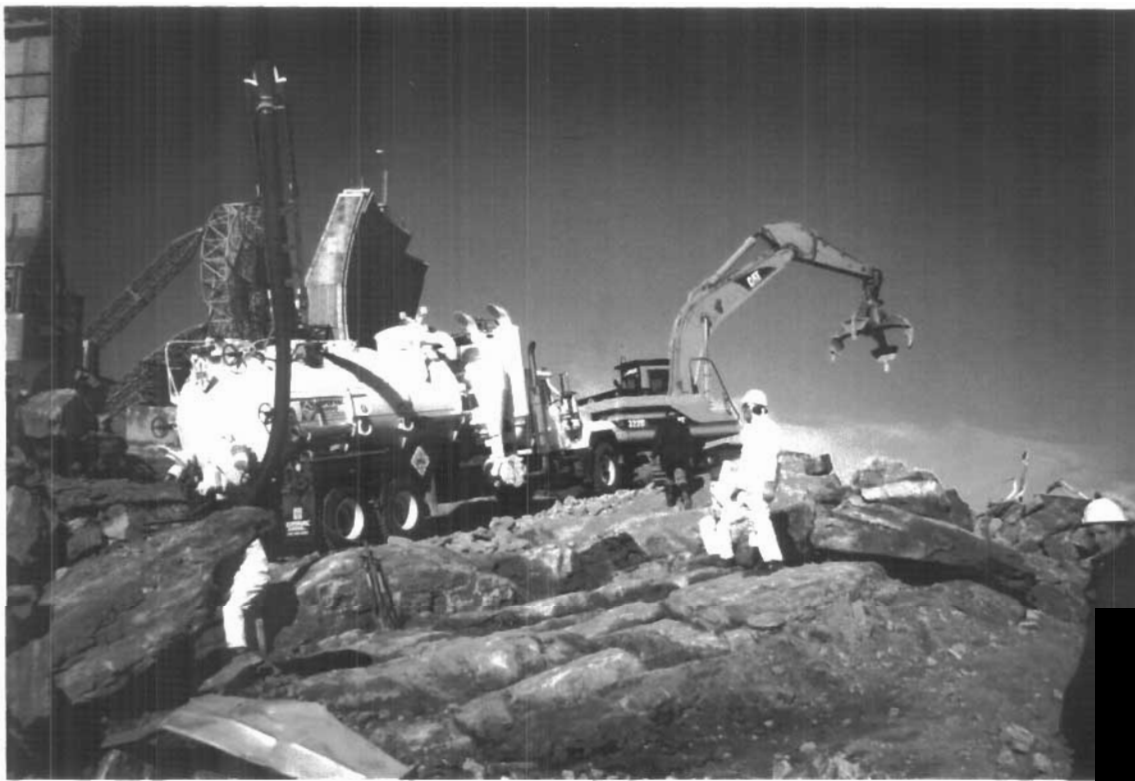
Photograph I-1: Excavating and Vacuuming PCB Contaminated Soils at the S1/S4 Valley Area
