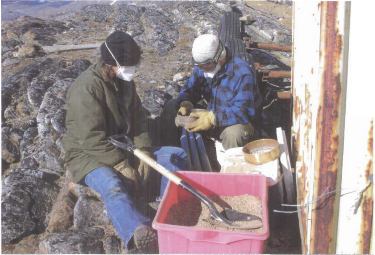
Photograph VI-8: Sieving Sand and Gravel for Filter Material
