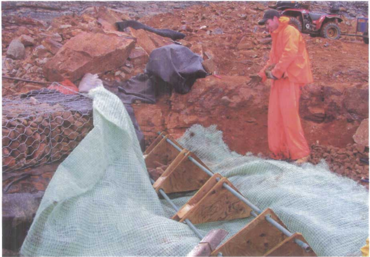
Photograph VI-12: Constructing One of the “Chevron” Water Impediment Sediment Trap Devices
