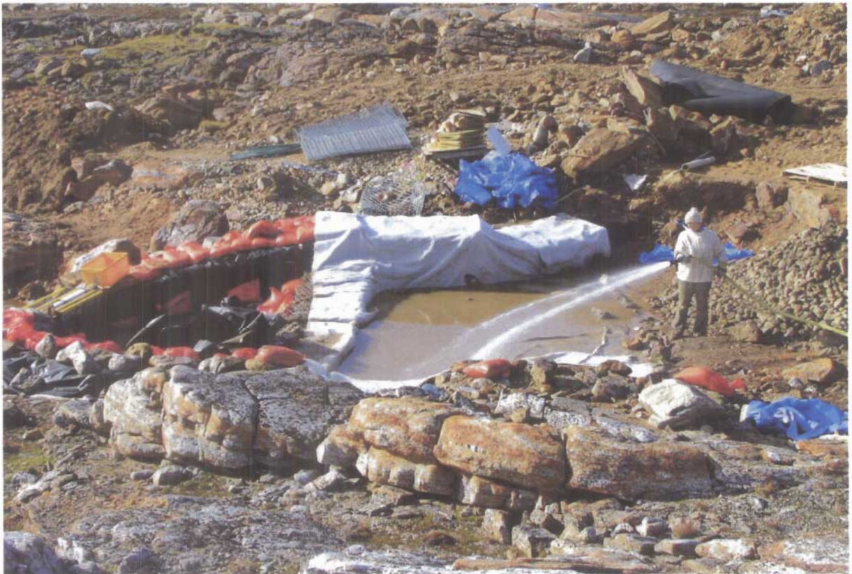
Photograph VI-11: GCL Was Used to Line the New Area and Force All the Drainage Water Through the Filter Box
