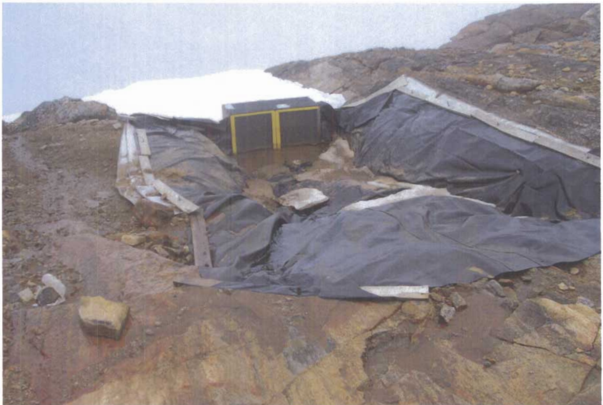
Photograph VI-15: The Furniture Dump Barrier at the Start of the 2004 Season: Note That Some Water and Sediment Had Not Passed Through the Funnel
