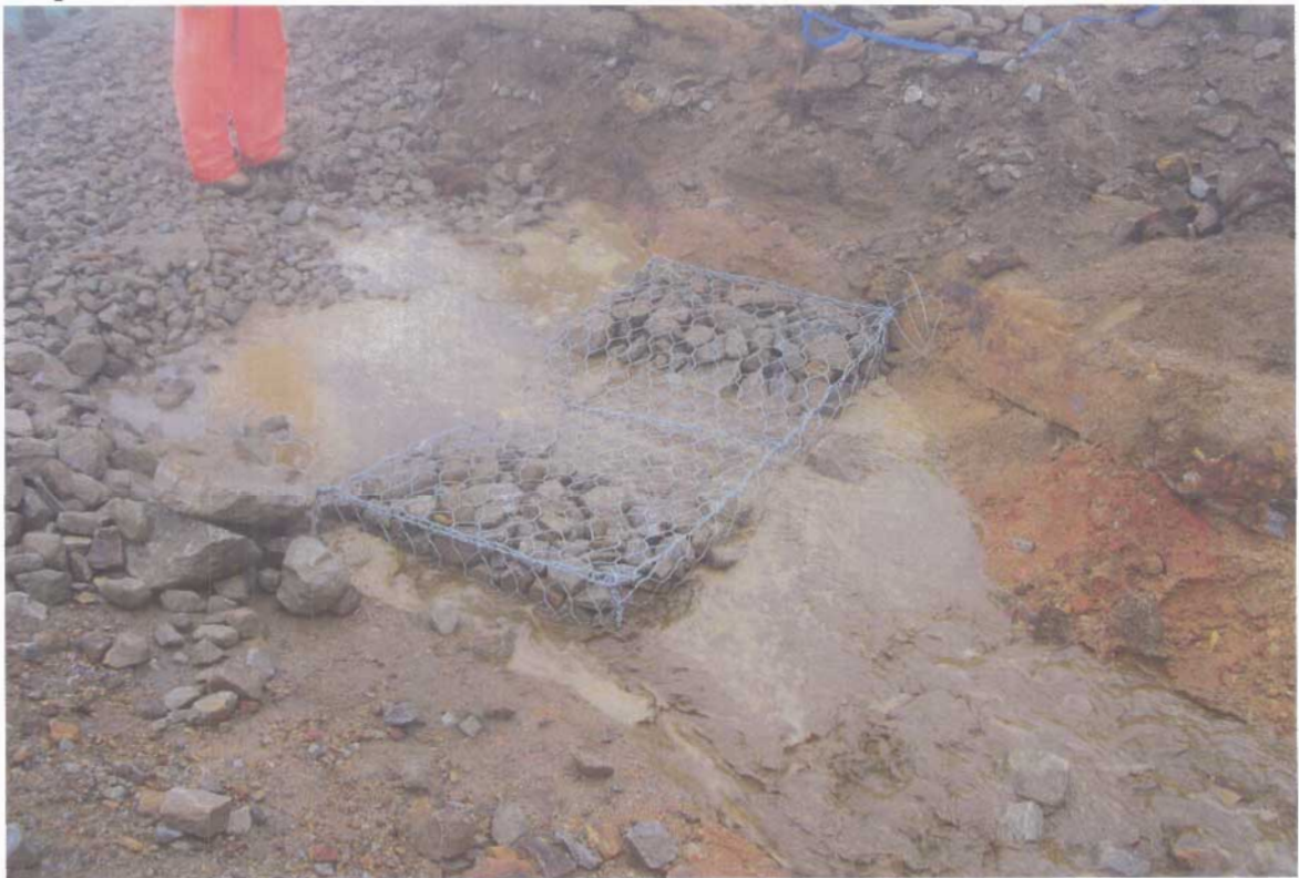
Photograph VI-13: The “French Bridge” Sediment Trap
