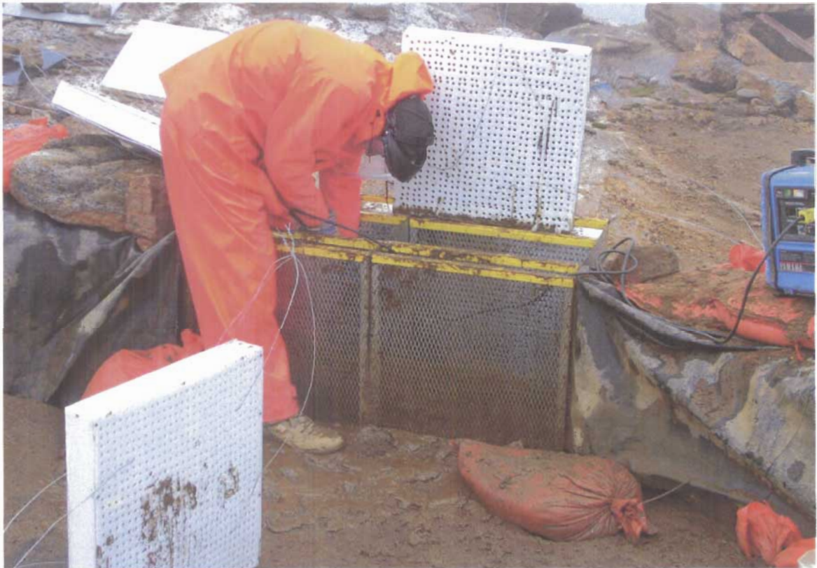
Photograph VI-9: Adapting the Filter Box for the New Filter Arrangement
