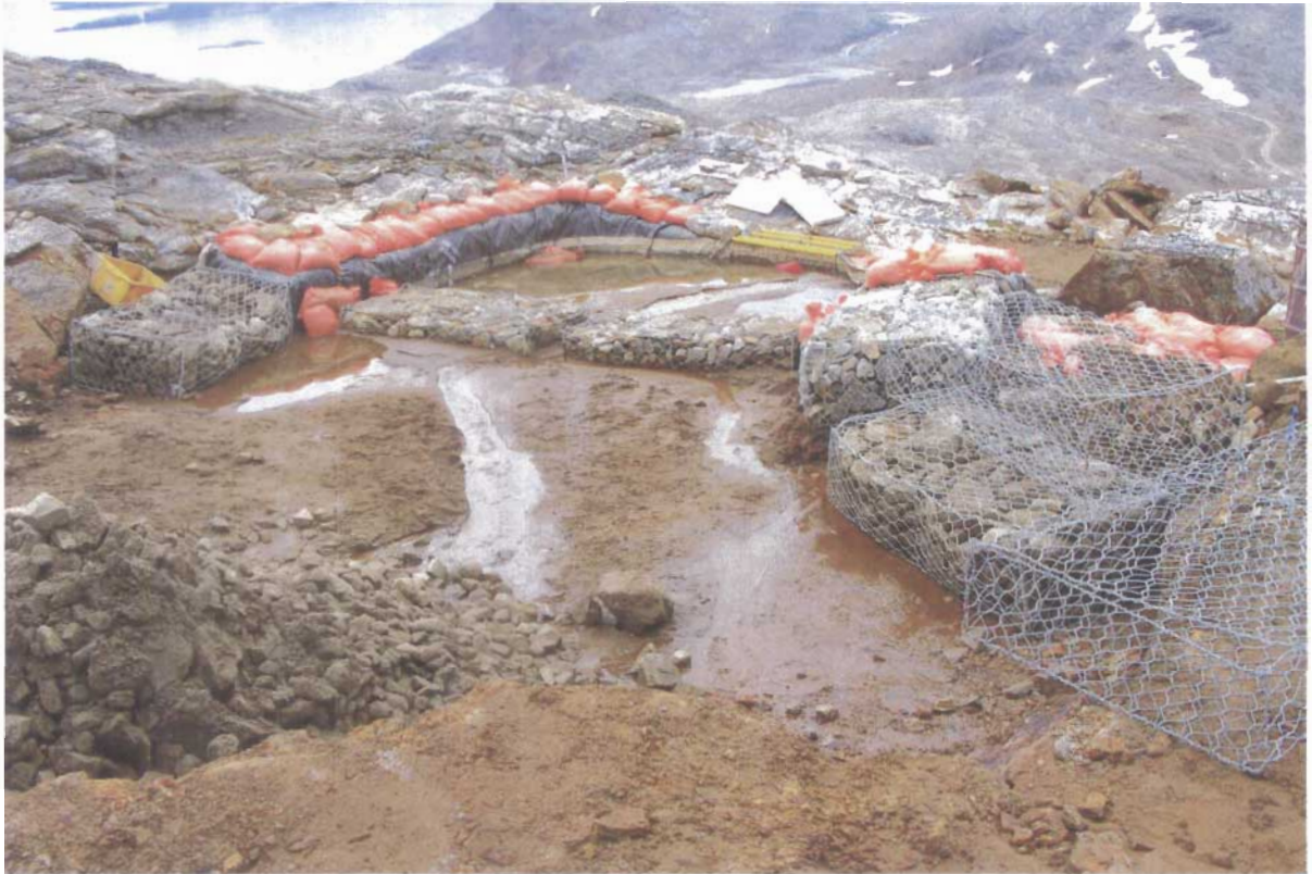
Photograph VI-10: Gabions Were Used to Extend the Length of the Funnel Trap
