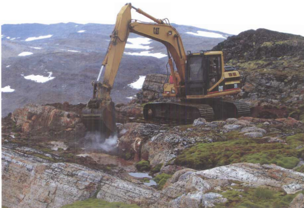
Photograph II-8: Starting the Excavation of Tier II Soil in the S1/S4 Valley at the End of the Valley Where a Lush Cover of Moss Predominates
