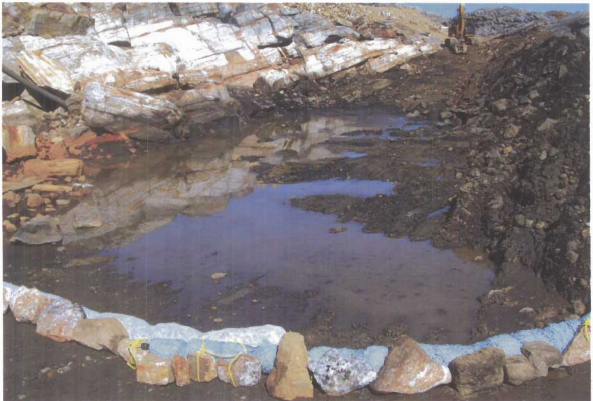
Photograph II-10: The Heavily Oiled Area in the S1/S4 Valley Was Boomed During Excavation of the Tier II Soil
