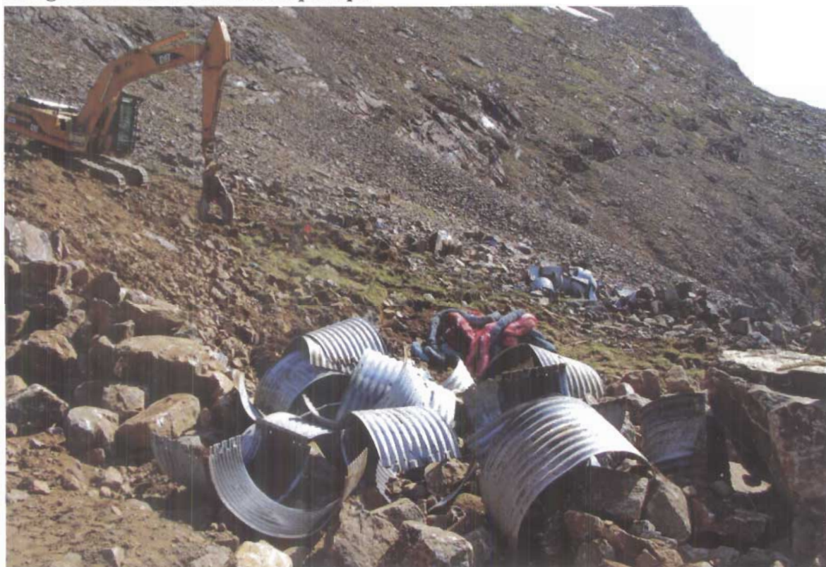
Photograph II-4: The Barrier Placed Across the Drainage Pathway in 1994 Was Removed. Analysis of the Barrier Material Showed That the PCB Level Was Tier II
