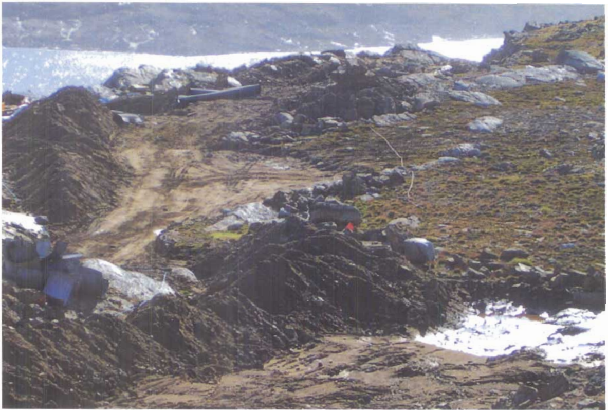
Photograph II-9: The Tier II Soil Excavated in the S1/S4 Valley Was Scraped into Piles
