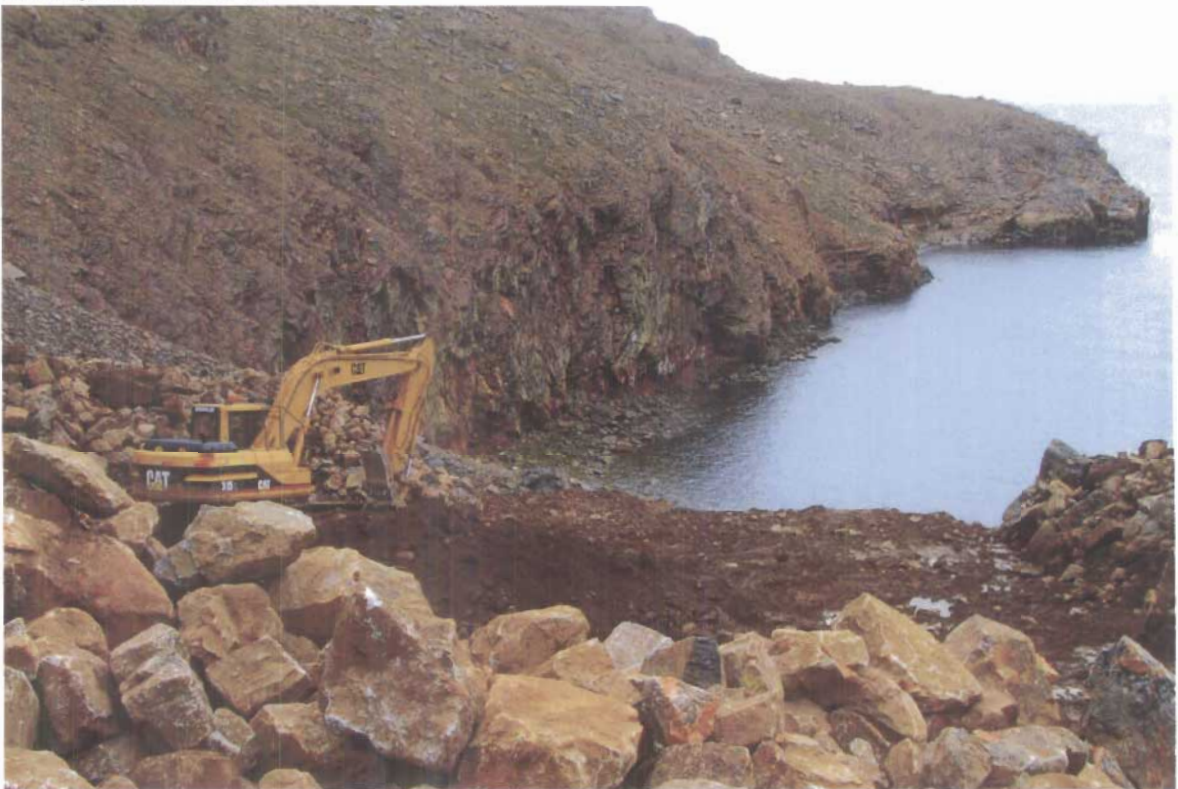
Photograph II-2: During the CEPA Soil Excavation Large Rocks Were Separated: The Excavated Soil Was Then Passed Through a Screener and Containerised
