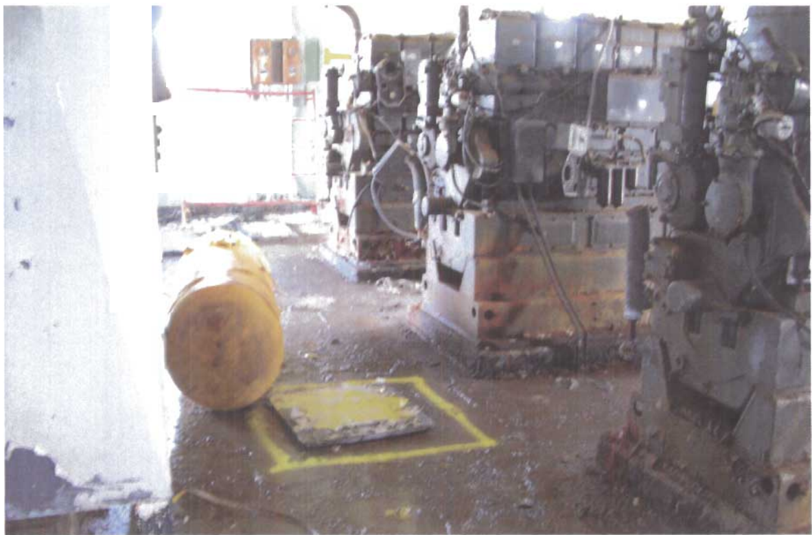
Photograph III-2: The Interior of Building S4 Prior to Demolition: The Area Marked in Yellow was Contaminated Above 50 ppm with PCBs
