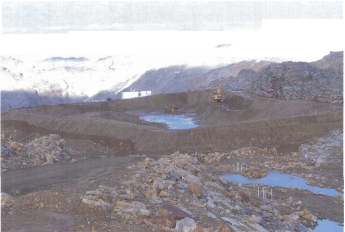
Photograph III-3: Construction of the Berms of the Tier II Landfill
