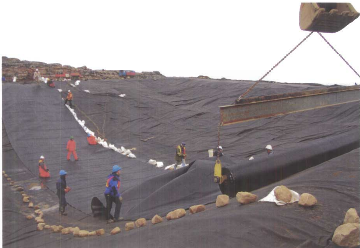
Photograph III-4: Installation of the Tier II Landfill Liner
