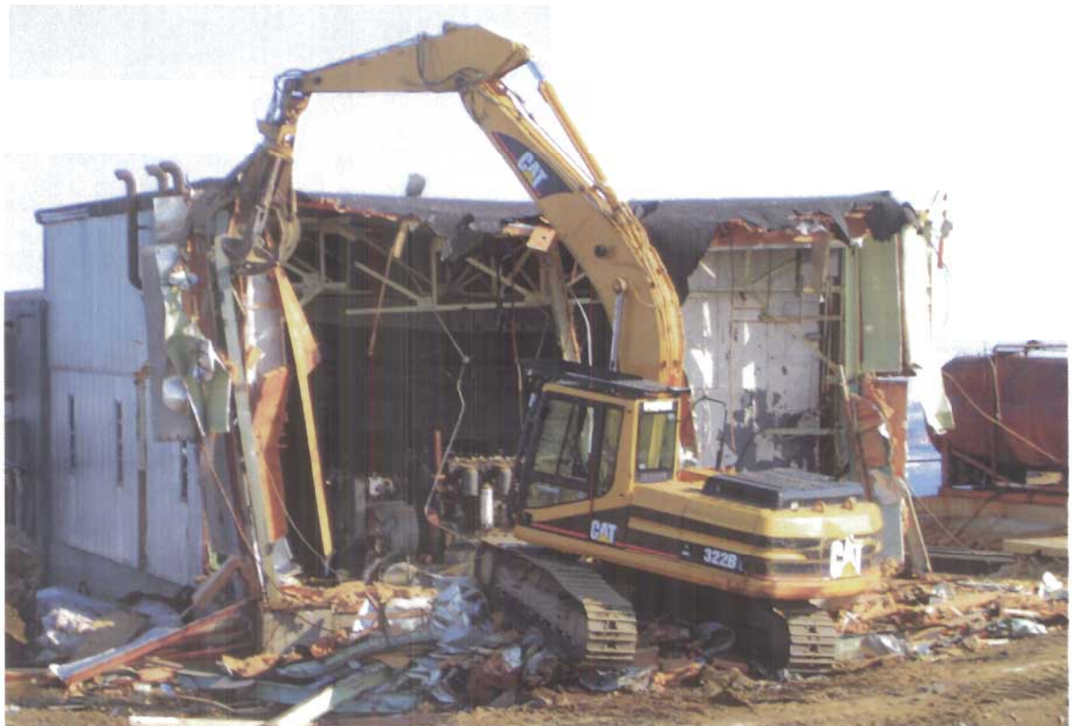
Photograph III-1: Demolishing Building S4. The Concrete Floor of the Building is Contaminated With PCBs and Will be Covered With Clean Fill
