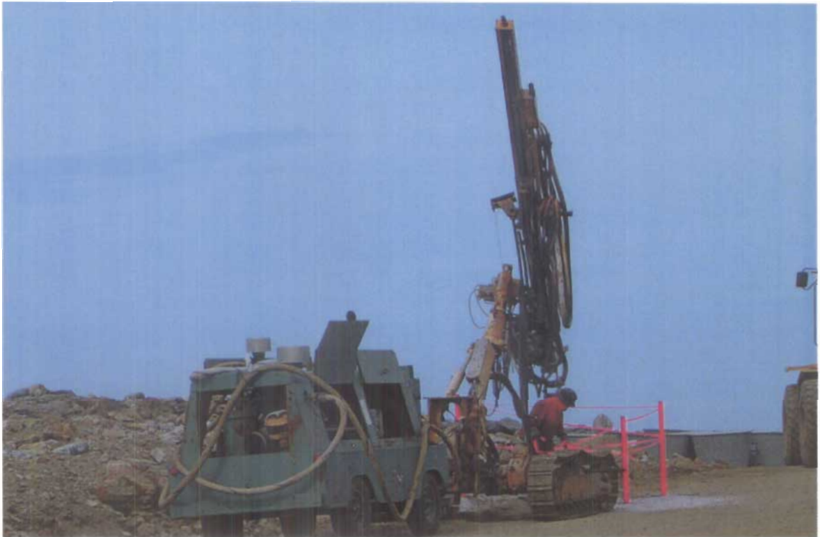
Photograph III-5: Installation of a Monitoring Well at Resolution Island
